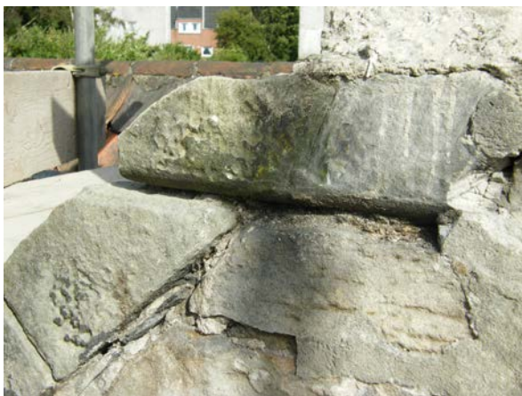
Figure 8 Reused stone within the 1888 rebuilding
