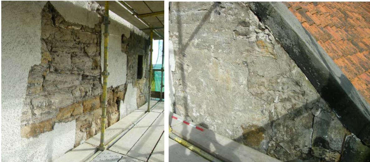
Figure 3 Horizontal break between the orange and pinker masonry and built over crow-steps Figure 4 Evidence for former crow-stepped gable head as revealed
