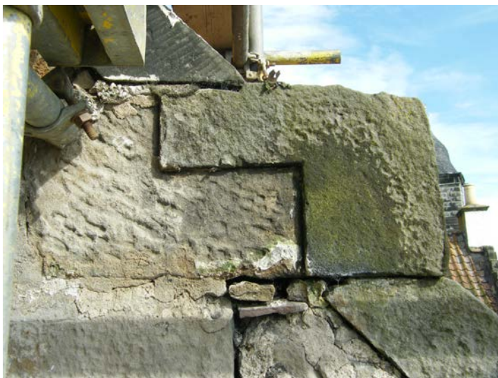
Figure 6 Intermediate skew stone
