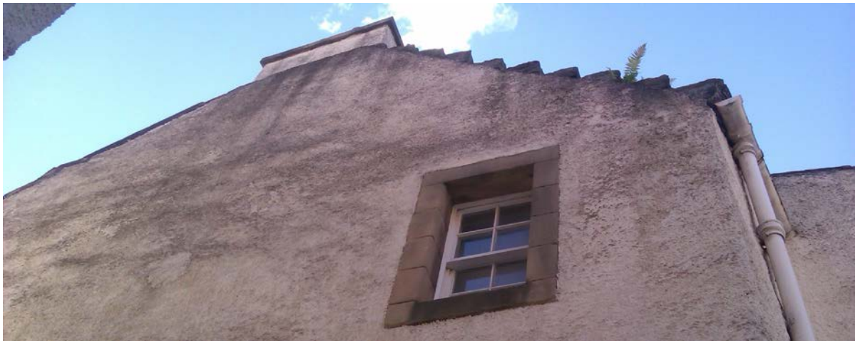
Figure 4 East gable wall showing surviving crow-steps on the rear pitch
