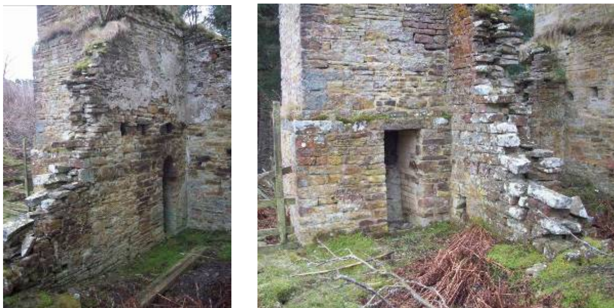
Plate 9 and 10: Arched interior opening and lintelled exterior
