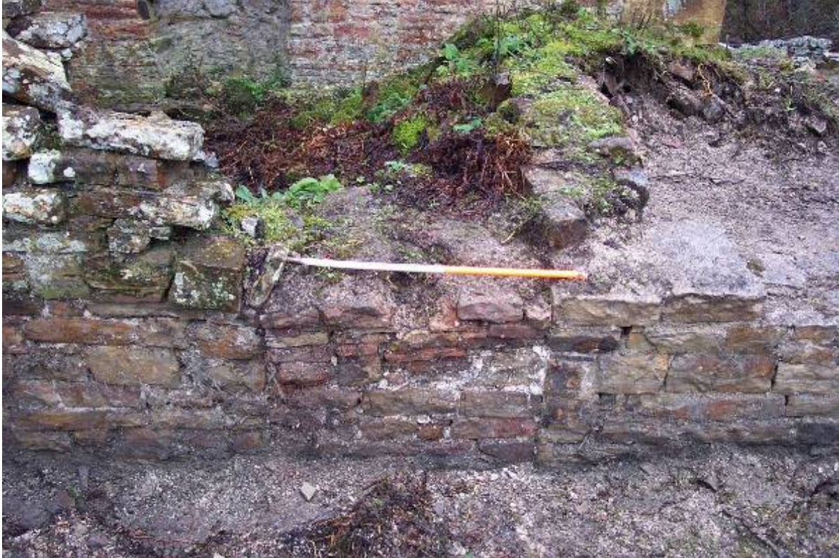
Plate 2: Blocked door uncovered during clearance.
