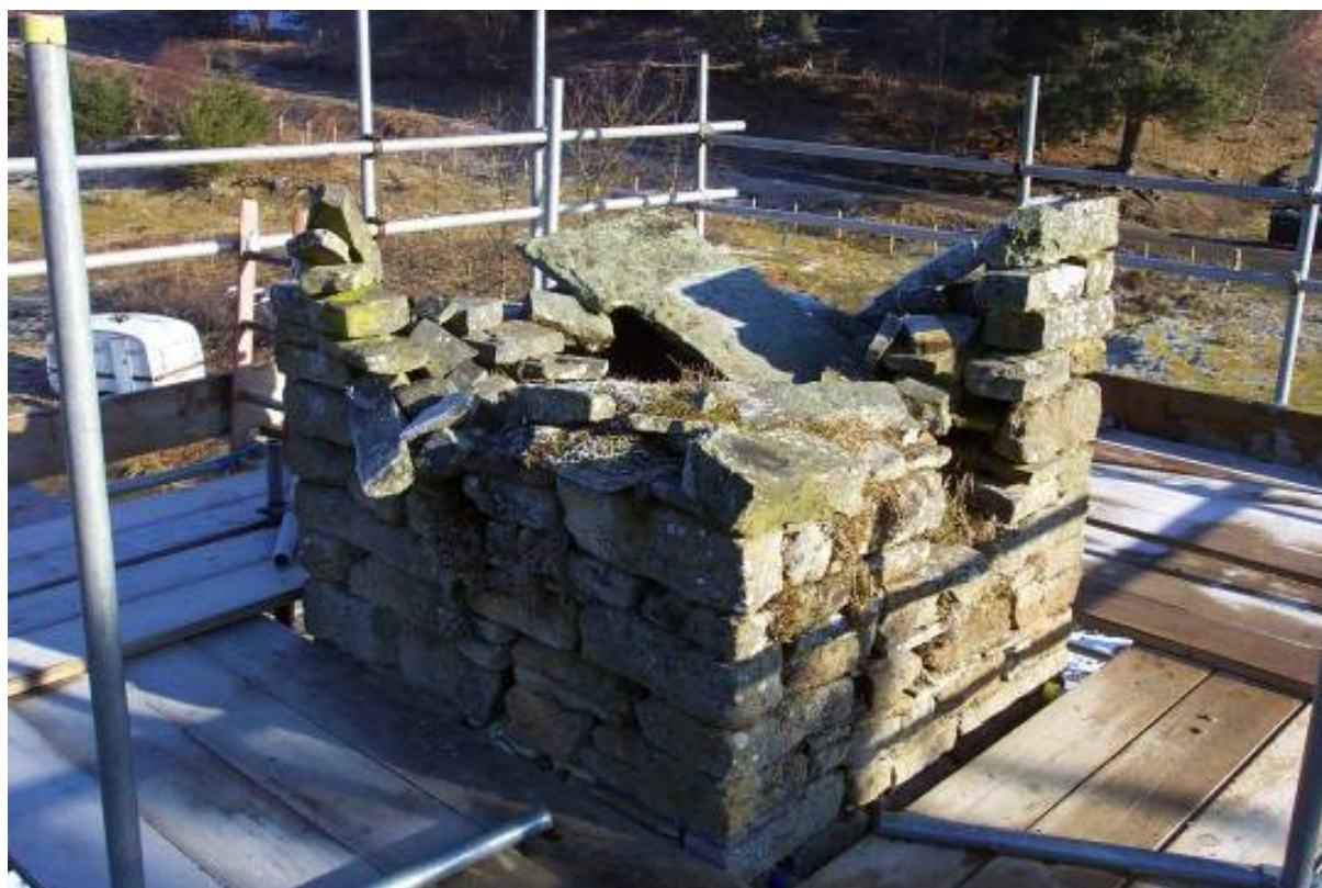
Plate 11: Top of chimney from scaffolding
