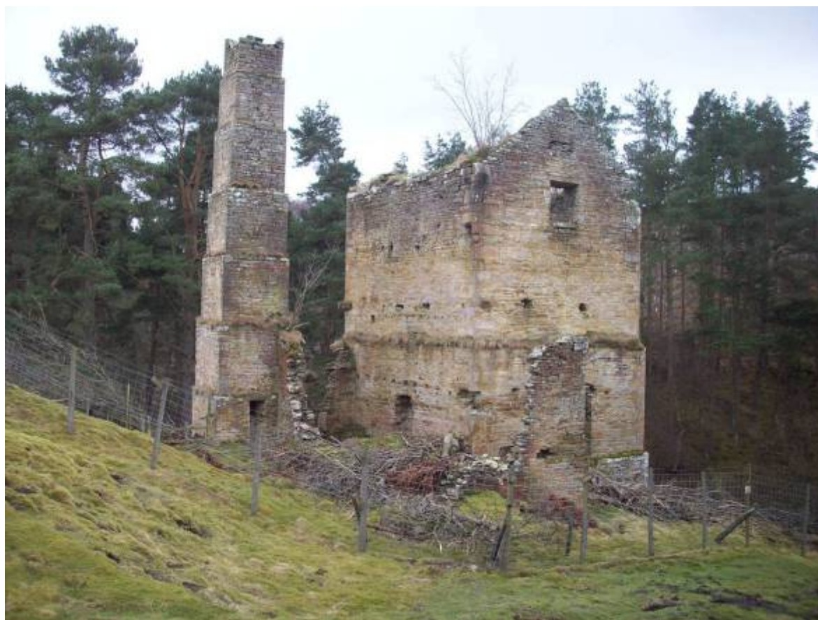
Plate 1: Pre clearance of boiler house.
