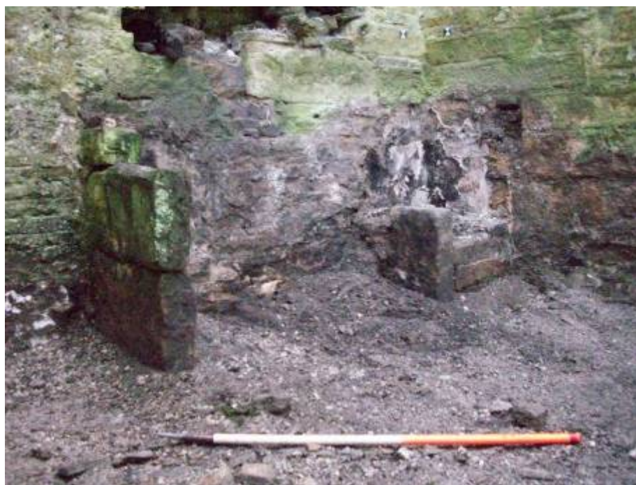
Plate 5: Inserted kitchen range in NE corner
