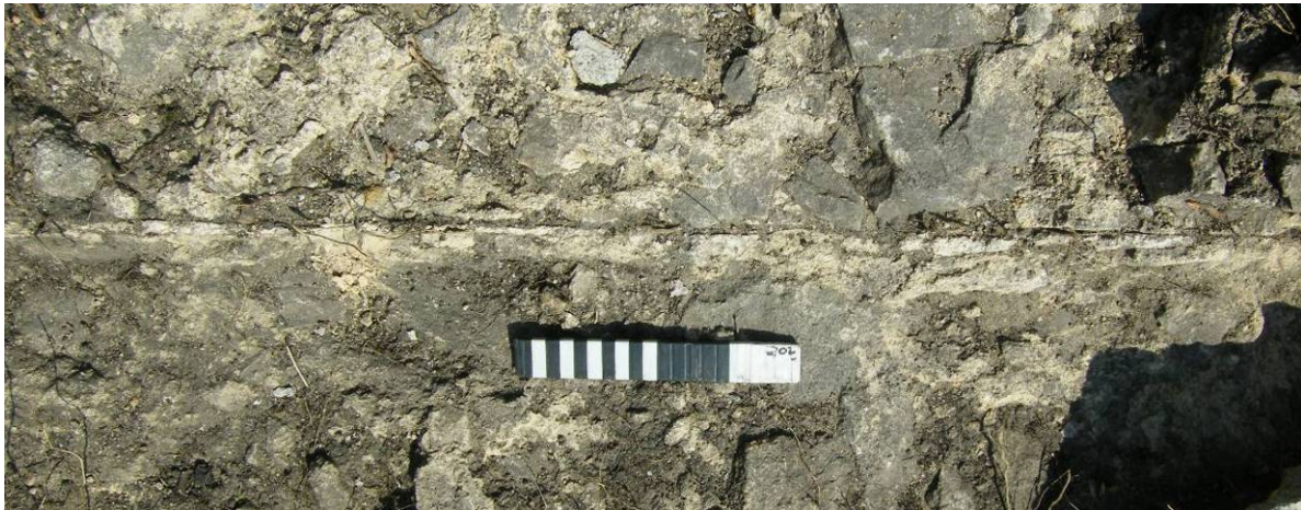
Plate 5.8 Detail of junction of chapel masonry 1023 (top) with that of the earlier gable wall 1010, preserving the original external plastered wall finish of the latter; east at top
