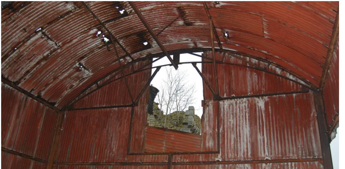
Plates 4.3 – 4.7 Dutch barn – internal views and constructional details
