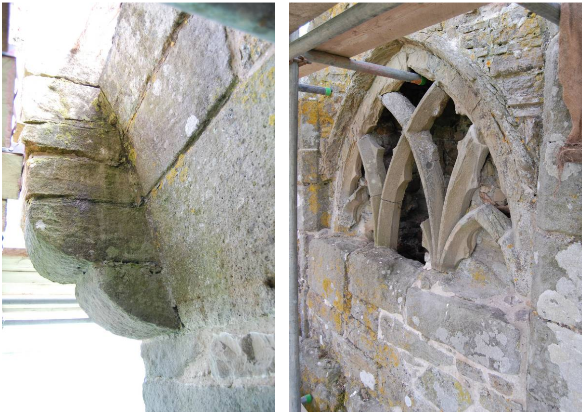
Plate 4.8 The SE angle tower of the chapel, upper parts showing arch springing on its north side Plate 4.9 Traceried head of secondary window within the east gable wall
