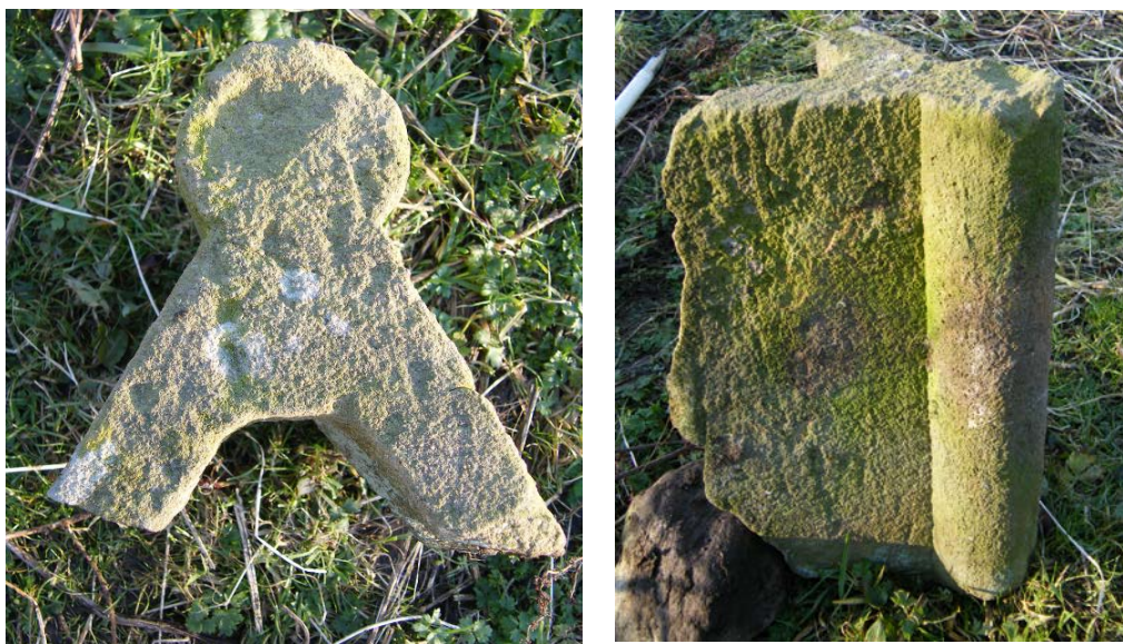
Plate 4.13 Medieval ridge-stone reused as a field wall coping
