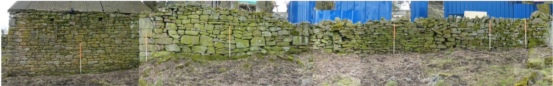
Plate 6.19 Composite view of boundary wall, north side, showing differing construction
