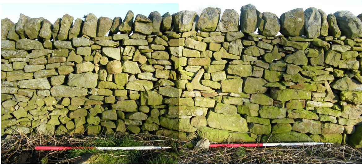
Plate 4.12 Field wall running south from the SE angle of the chapel range, west side. Note the medieval ridge stones incorporated within the wall
