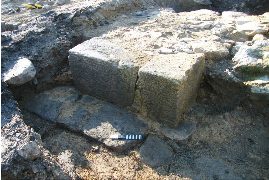
Plate 6.5 Base of pilaster buttress at the centre of the east gable wall of the early range; looking SW
