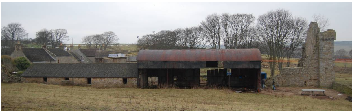
Plate 4.2 General view of the barn and adjacent structures from the south
