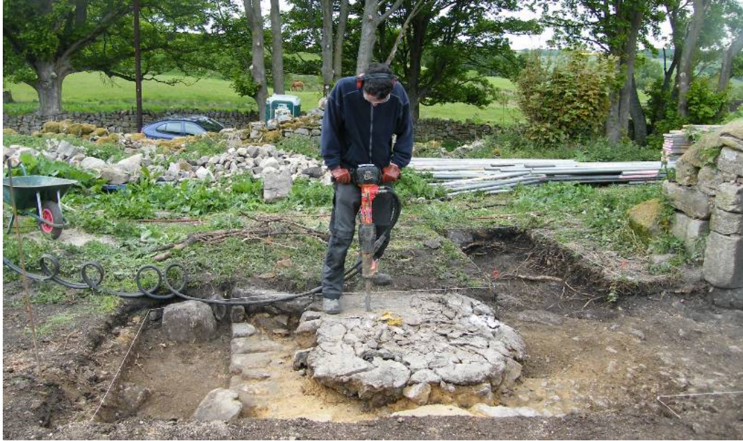
Plate 5.2 breaking the concrete pier base 1004, looking north
