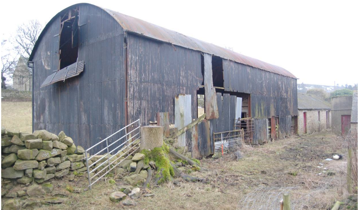
Plate 4.1 General view of the Dutch barn from the NE
