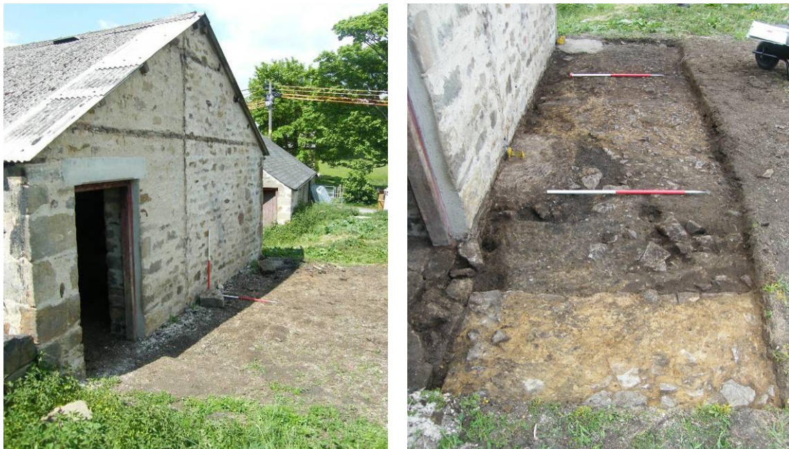
Plate 5.10 Trench 2, before excavation, looking NW
