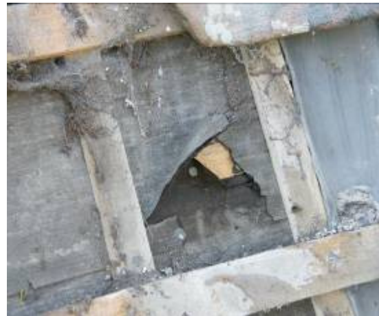
Figure 33 - Opening 1 at lowest level of investigation Figure 34 - Opening 1, detail of sarking below tile.
