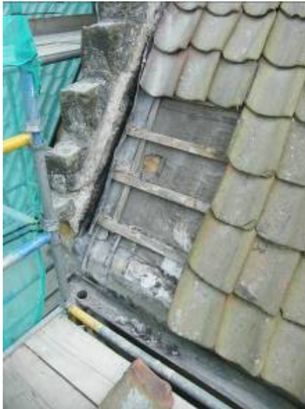
Figure 35 – Opening 2 at LOE.
