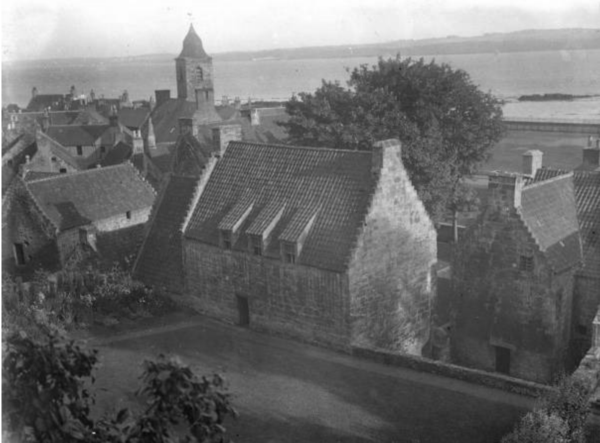
Figure 23 – Early photograph, probably mid to late 1930s 4 , showing north elevation with three dormers and the crowsteps on the W gable reinstated. The small lean-to structure to W has seemingly been demolished. ©RCAHMS [11_1104524]. Licensor www.rcahms.gov.uk .
