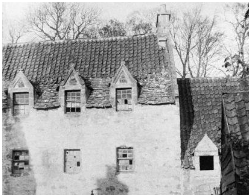
Figure 30 - Photograph of the North Range in ca. 1888, showing the lowest courses of the roof as slated. ©National Museums Scotland. Licensor www.scran.ac.uk.
