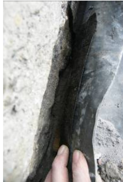
Figure 36 – detail of modern sarking below lead flashing at Opening 2
