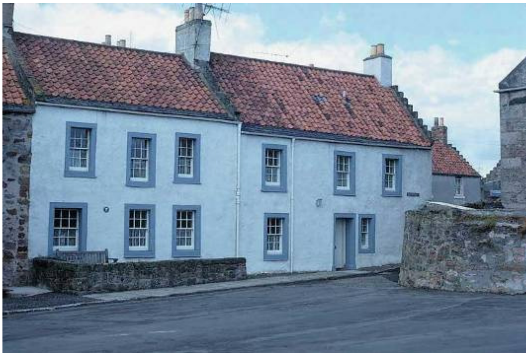
Figure 32 – Nos. 5-7 Rumford Cottage, Crail, after restoration by The National Trust for Scotland in 1961. ©National Trust for Scotland. Licensor www.scran.ac.uk .
