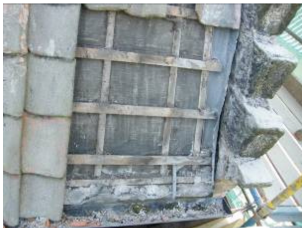
Figure 33 - Opening 1 at lowest level of investigation Figure 34 - Opening 1, detail of sarking below tile.
