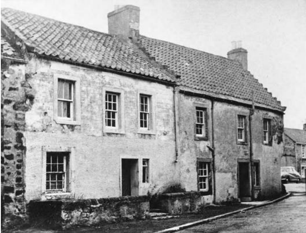
Figure 31 – Nos. 5-7 Rumford Cottage, Crail, before restoration in 1961 by The National Trust for Scotland. ©National Trust for Scotland. Licensor www.scran.ac.uk .
