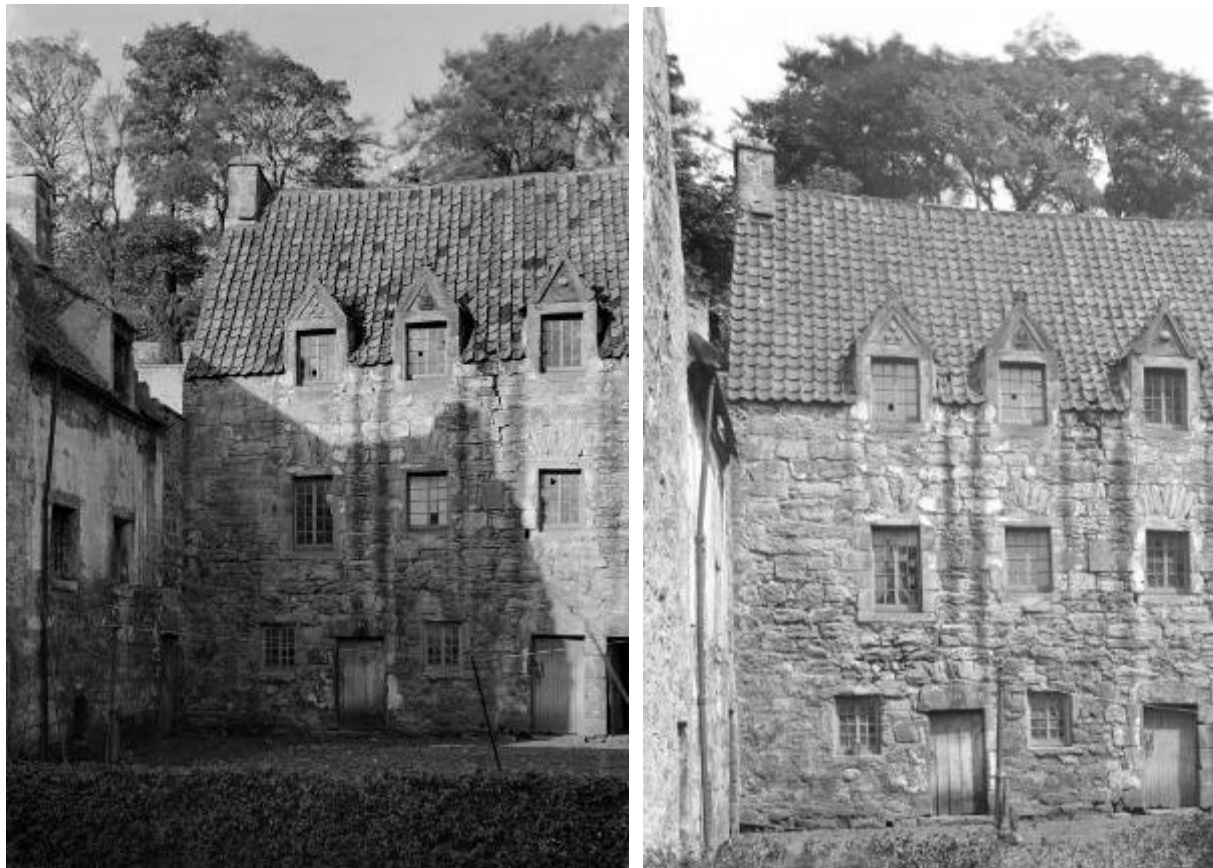
Figure 22 – Two early photographs (right one collected before 1930s, left dated 1926), showing the missing crowsteps on the W gable, S façade. ©RCAHMS [11_1106693 left and 12_1205882 cropped]. Licensor www.rcahms.gov.uk
