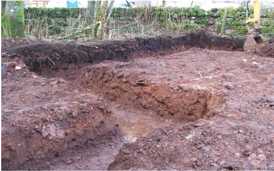
Plate 3 General view of foundation trenches under excavation (0.50m scale).
