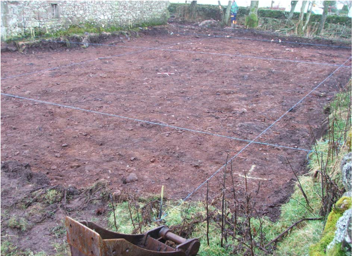
Plate 2 Post excavation of northern area (Photograph 048) with foundations being laid out.
