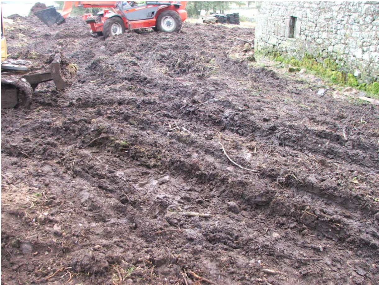
Plate 1 Pre excavation (Photograph No. 004)
