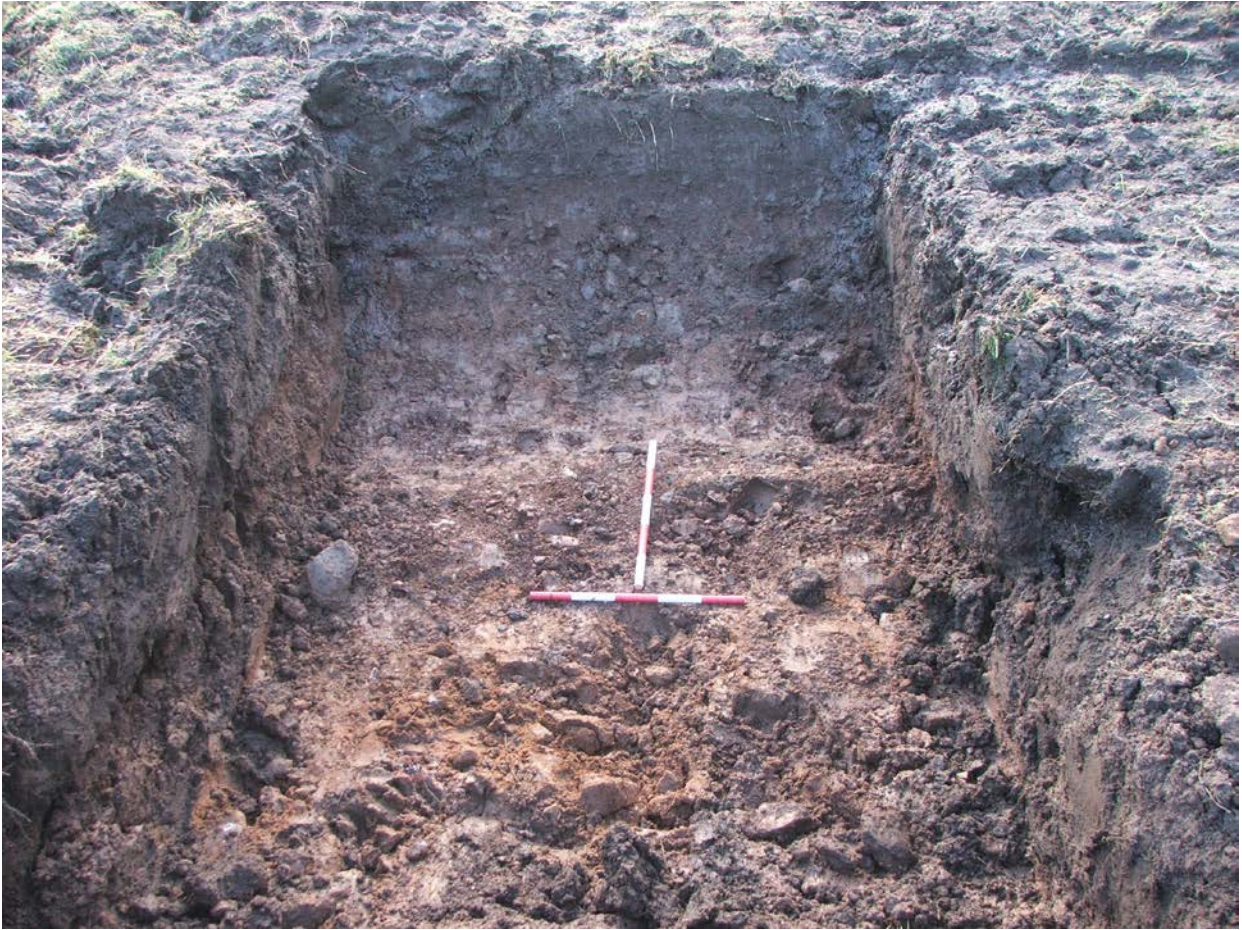
Plate 5 Septic tank trench at monitored limited of excavation (LoE) showing natural deposits at base.
