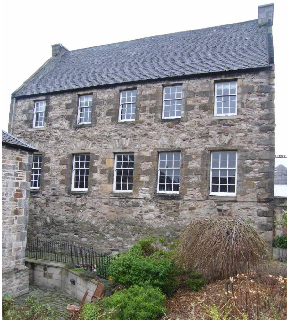
West frontage of Panmure house
