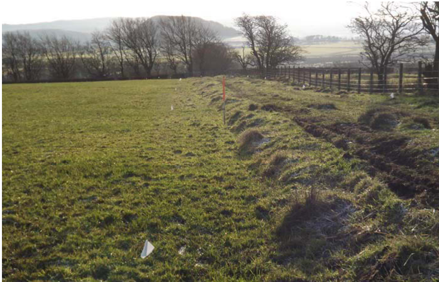
Plate 14 Looking SSW along the route of the site access track with the disused farm track visible along the fenceline
