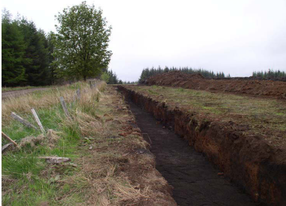
Plate 13 Cables trenches
