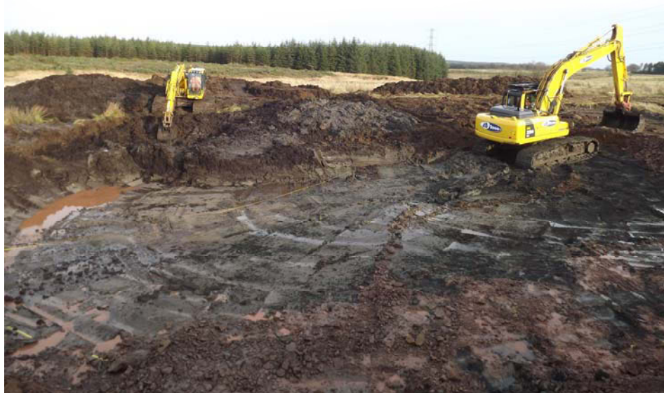
Plate 2 Excavating the original location of Turbine 4
