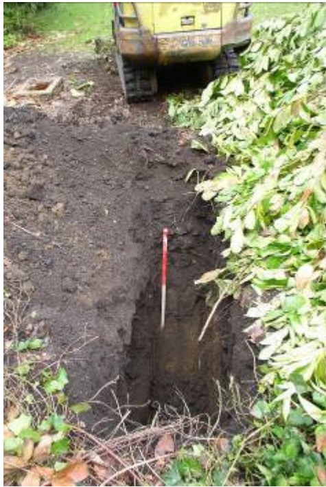
Figure 7 Trial Pit 1: post-excavation, E-facing section (Nr. 003)
