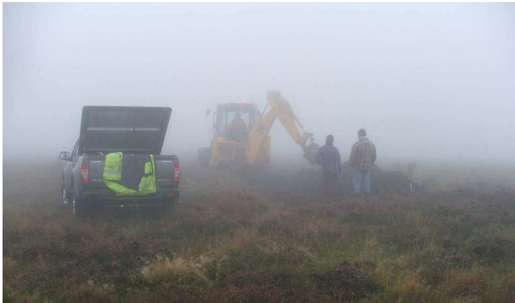
Plate 2 Opening up Trench 1 in the fog
