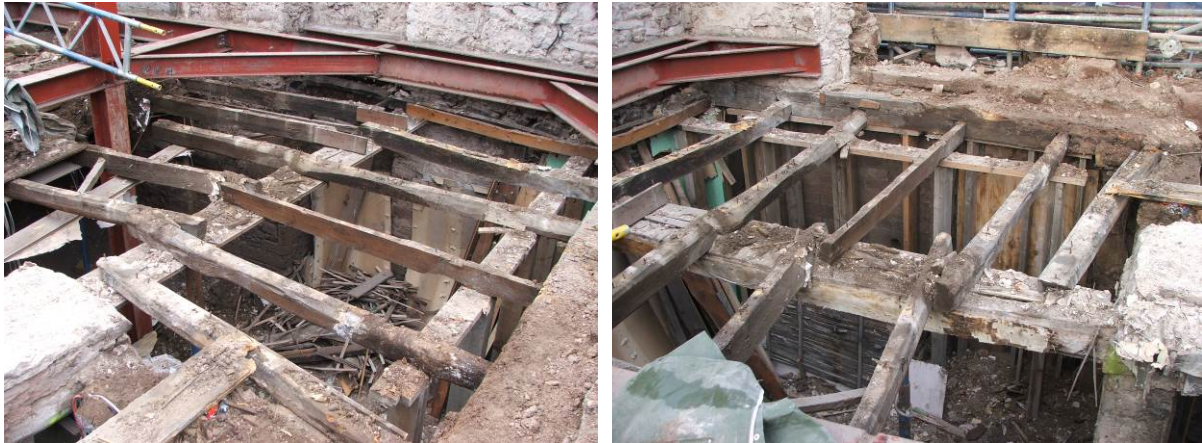
Plate 11-12 The first floor floor structure, showing the shorter panels of common joists extending to the street frontage
