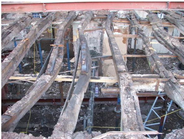
Plates 13-16 Second floor floor structure – note the sinuous and unworked nature of the timbers employed, including branched ends, plates 17-18, below
