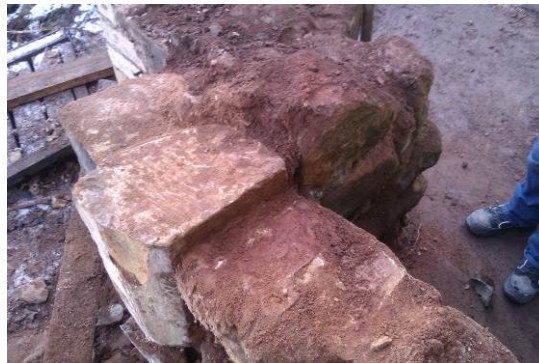
Plate 47 Junction of link (foreground) and main walling rear range
