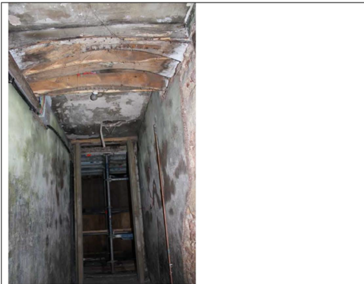
4 Curved ash (TBC) forming arched ceiling in part of central pend. There are 3 whole sections of ash (?) stems and some probably later inserted boards. Photo: C Mills.
