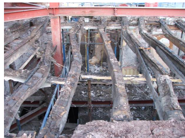
Plates 13-16 Second floor floor structure – note the sinuous and unworked nature of the timbers employed, including branched ends, plates 17-18, below
