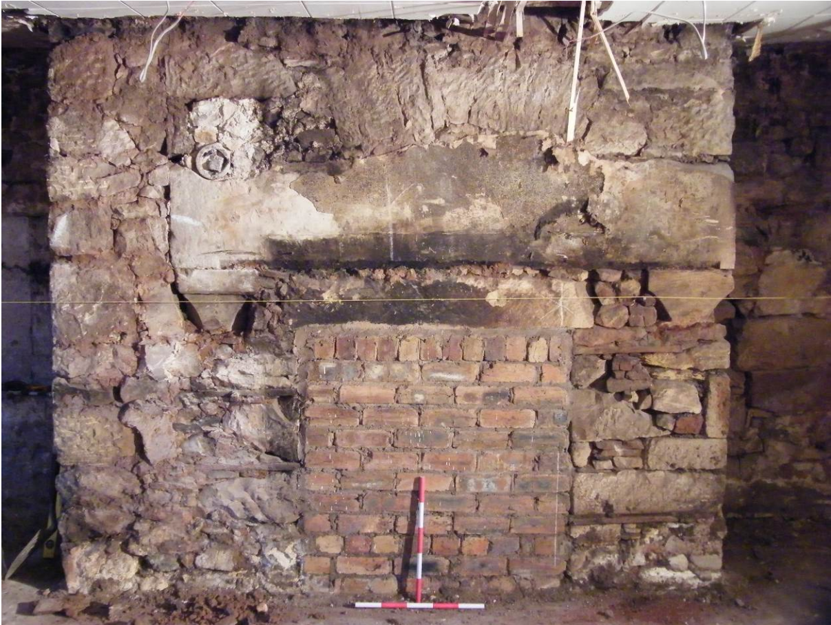
Plate 8 The remarkable fireplace within the lower stage of the SW chimneybreast
