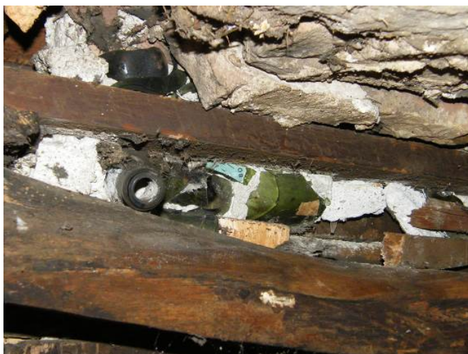
Plate 50 Glass embedded in mortar between/above joists 038/039
