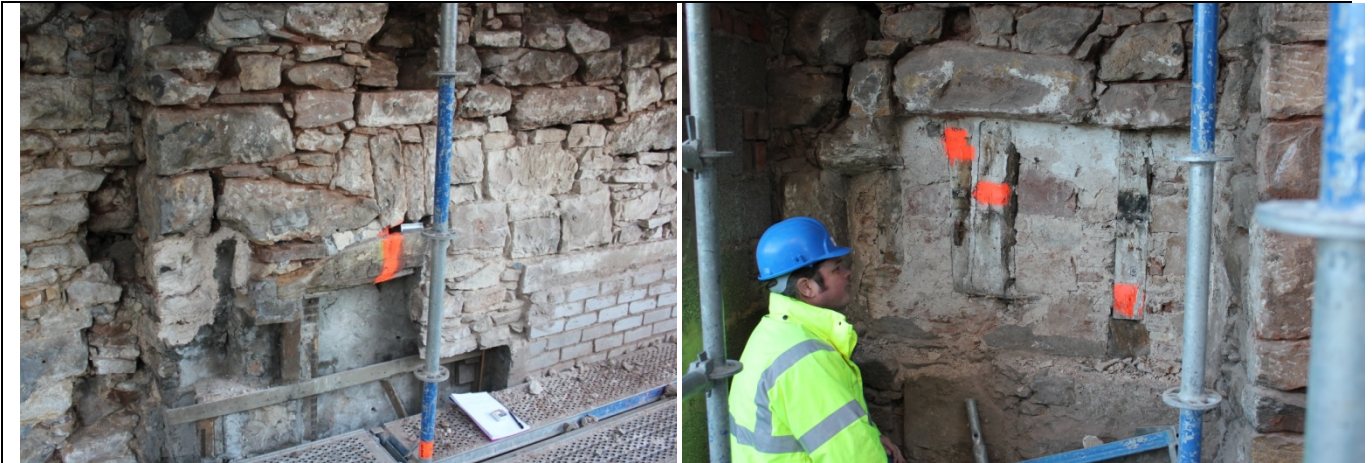
Plate 6 (L) Oak lintel F100, marked for extraction with orange paint, in the ground floor fireplace in the East gable wall. The fireplace may be one of the earliest surviving features. The fireplace and its lintel have been cut through by later modifications to this side wall. (R) Studs in F110, on the West gable wall, marked for extraction prior to gable rendering.
