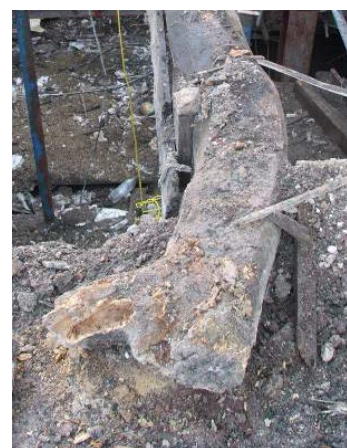
Plates 13-16 Second floor floor structure – note the sinuous and unworked nature of the timbers employed, including branched ends, plates 17-18, below
