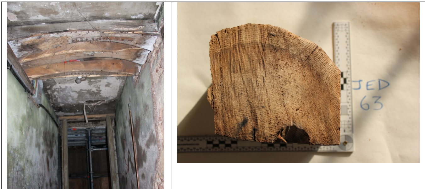
Plate 3 Some of Group B timbers: (L) The curved oak elements forming an arched ceiling to the central pend on the ground floor; (R) sample of F63 the principal oak joist in the ground floor ceiling, on the old frontage line in the NW part of the building
