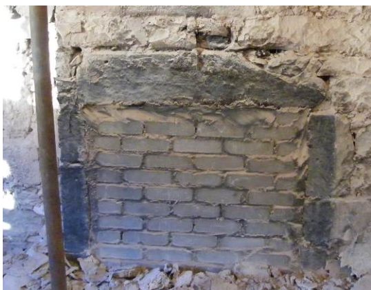
Plate 3 Remains of the turnpike stair at the east angle of the main range – note entrances behind the new steelwork and the curvature of the lower part of the stairwell to the right of the scale pole.
