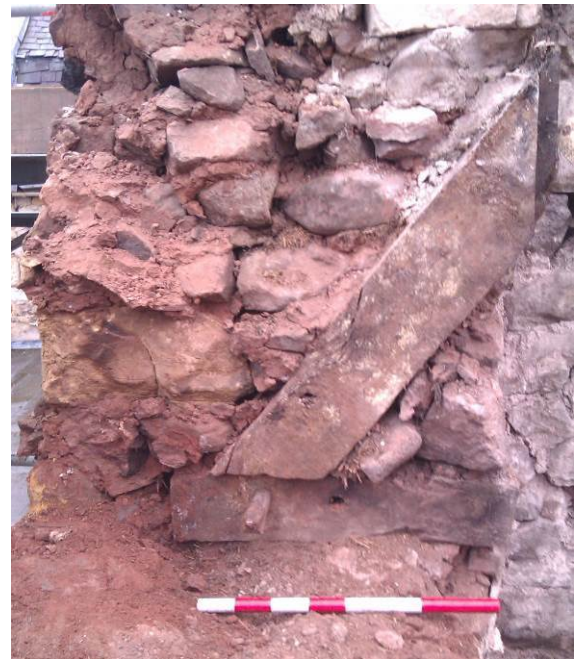
Plates 22-25 Four of the surviving rafter foot assemblies embedded within the rear wall, during demolition
