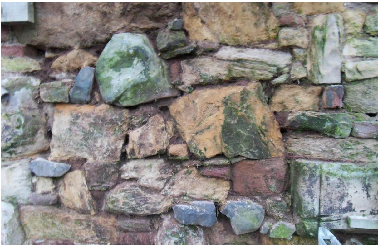
Plate 5 An illustration of the mixed nature of the stone employed in much of the phase II construction including a variety of sandstone types and some whin; some if not most of the of the former are evidently recycled from other structures – e.g. block to lower right; rear wall (context 127)
