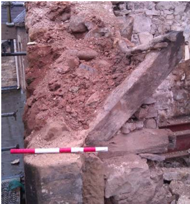
Plates 22-25 Four of the surviving rafter foot assemblies embedded within the rear wall, during demolition
