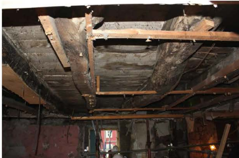
Joists of crooked and branched oak revealed in 1 st floor ceiling; potentially a very rare native oak structure of late medieval or early post-medieval date. Relicts of Jed Forest? Just one example of the remarkable timber assemblage in this building. Dendrochronological analysis is recommended for dating the structure and characterising and dendro-provenancing the timber (Photo: C Mills)
