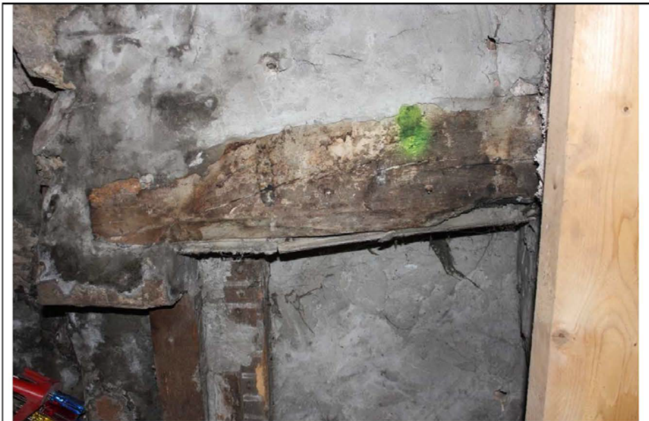
6 A substantial oak lintel rests over the fireplace on the ground floor NE side wall. Photo: C Mills.
