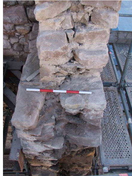
Plate 19 (left) Remains of the phase II wall head revealed as an off-set; embedded crow-steps can be seen behind the scale pole.
