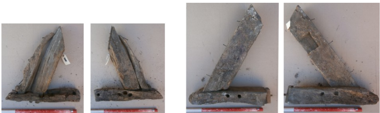
Plates 32-33 Rafter-foot assemblies 005 and 006
