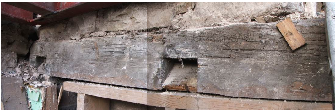
Plate 48 Timber lintel displaying shipping marks incised with a rase-knife
