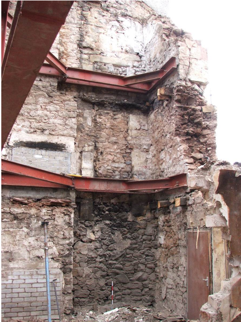
Plate 3 Remains of the turnpike stair at the east angle of the main range – note entrances behind the new steelwork and the curvature of the lower part of the stairwell to the right of the scale pole.
