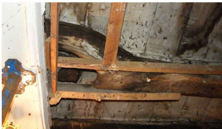
Plates 13-16 Second floor floor structure – note the sinuous and unworked nature of the timbers employed, including branched ends, plates 17-18, below
