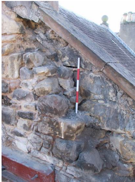
Plate 19 (left) Remains of the phase II wall head revealed as an off-set; embedded crow-steps can be seen behind the scale pole.
