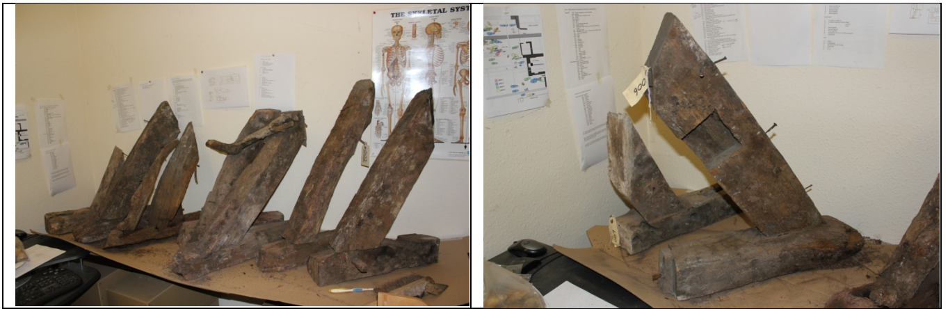
Plate 4 Group C (L) The oak rafter feet assemblies from an earlier roof, some elements with clearly redundant features, like (R) this slot on Rafter 006 which may be a sawn-through mortise slot or a former cross-lap joint. However some of the elements have no sign at all of re-use and there may be a mix of re-used and original timber, which should become evident in the tree-ring results.
