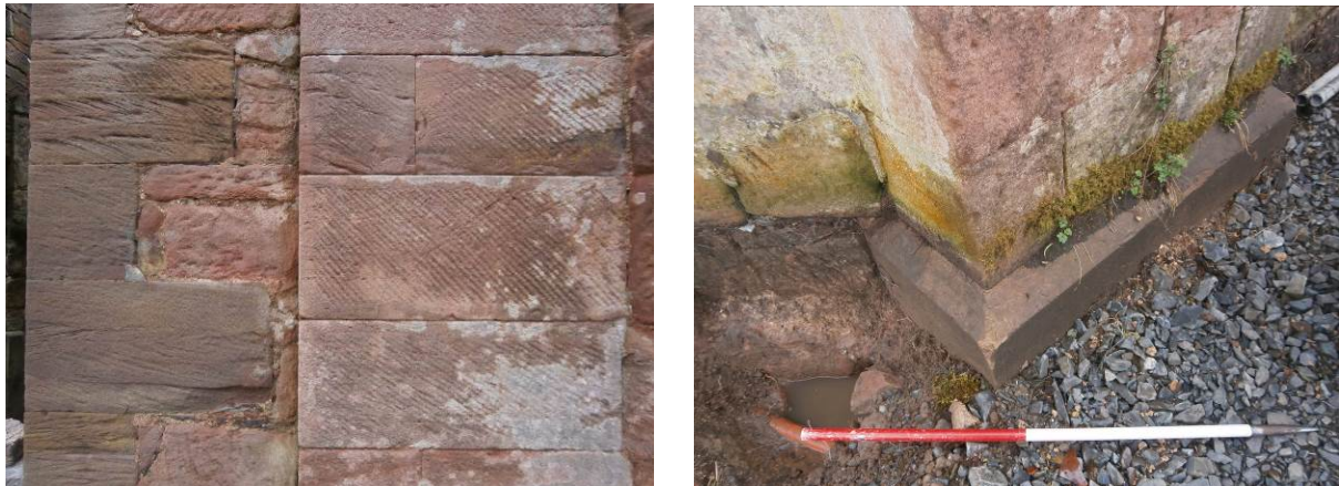
Plate 3 Details of different stone types and finishes – left: droved and polished dressings and broached rubblework; right: plinth of polished fine-grained stone (2014 - Photographs 290 and 491)
