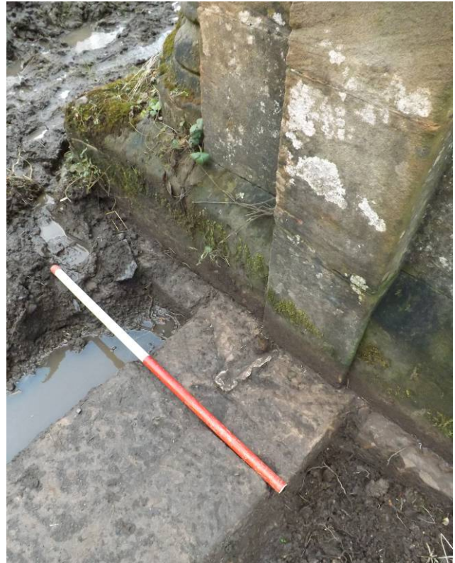
Plate 7 The westernmost lead-fast iron pintle of the gateway (2014 - Photograph 274)
