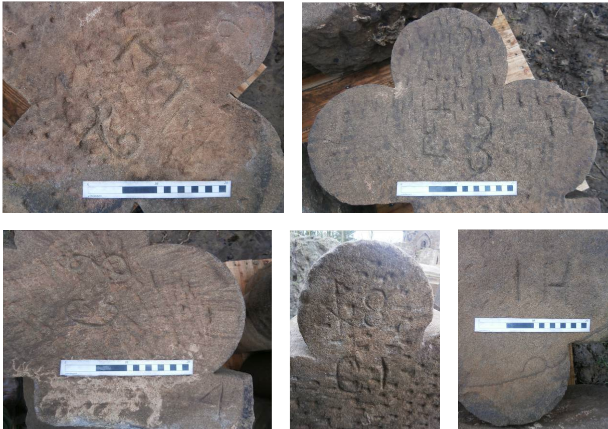
Plate 58 Carved stones from the dismantled archway showing numbering (E2, E3, C3, C1, H1) applied in the 1960s, and earlier numbering and masons' marks (2014 – Photographs 330, 332, 335, 339 and 336)
