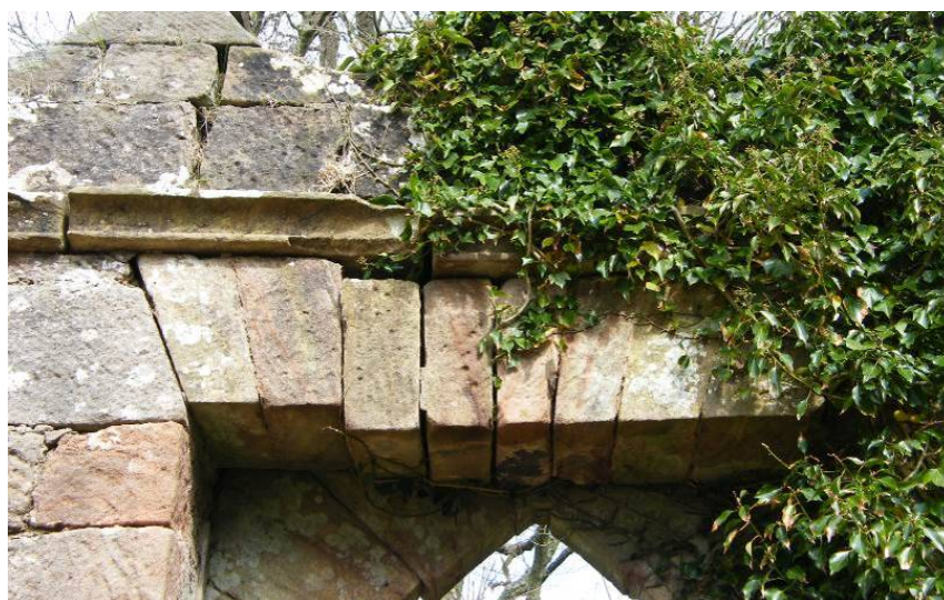
Plate 10 Detail of dropping flat arch on eastern flanking wall , (2008 – Photograph 080)
