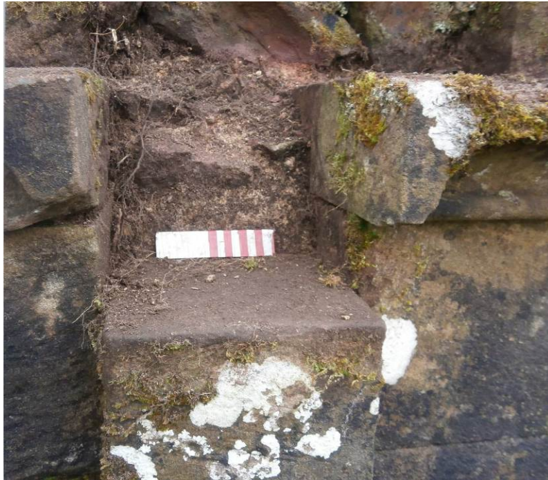
Plate 8 Detail of socket for flying lintel in top of gate pier (2014 – Photograph 350)
