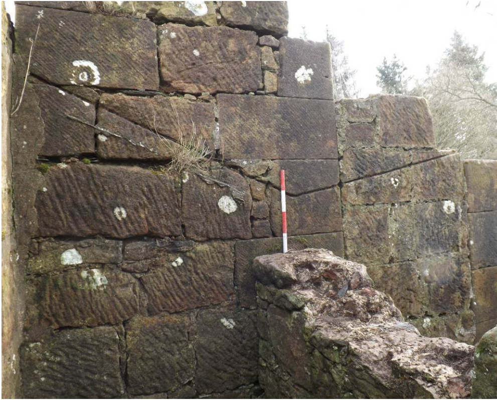
Plate 49 Detail of the raggle for the lean-to (2014 – Photograph 477)
