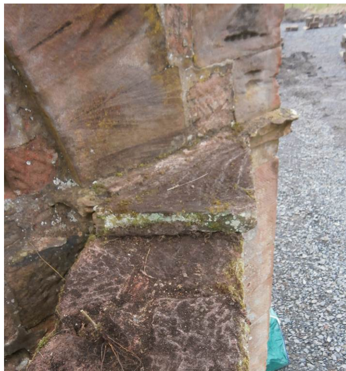
Plate 30 Cope detail on the north wall of the east wing (2014 – Photograph 354)
