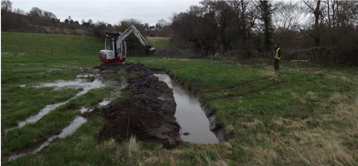
Plate 9 Temporary drainage in the north eastern corner of the Cricket Pitch (Photograph 049)
