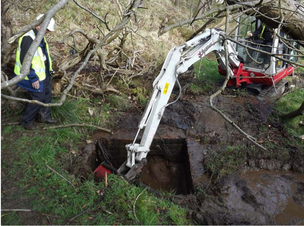
Plate 10 Opening the brick lined chamber (Photograph 042)
