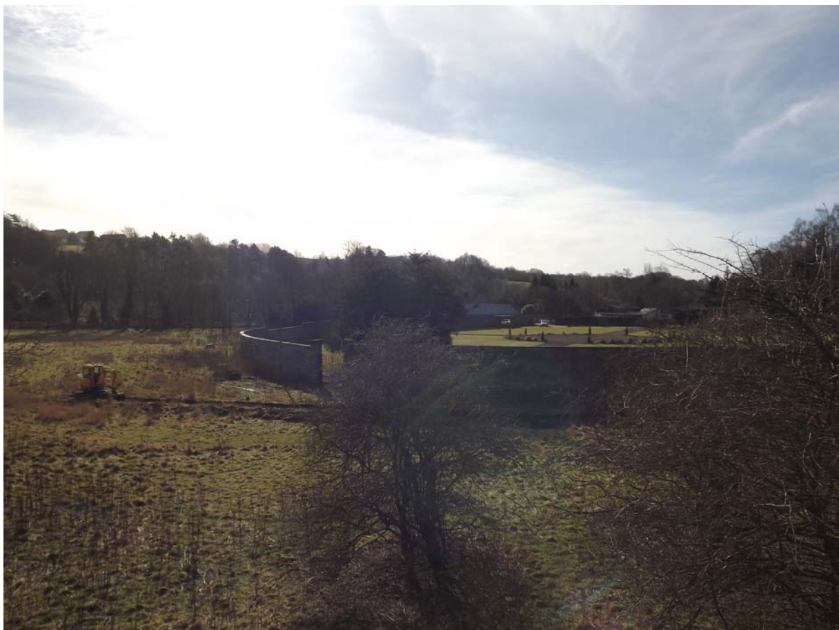
Excavating the path around the walled garden
