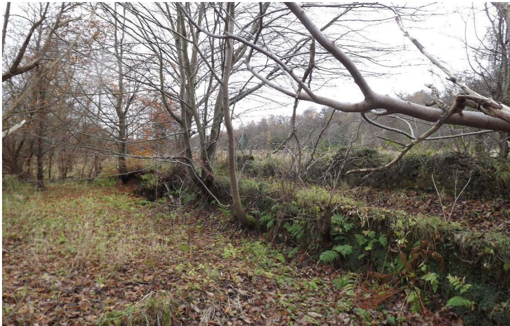
Plate 4 Revetting wall along the route of Path Two, building up this area to form a raised pathway
