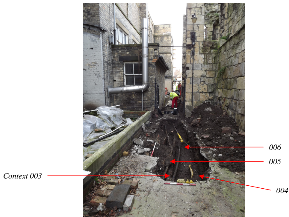
Figure 2 Post-ex view of trench facing NW (015)
