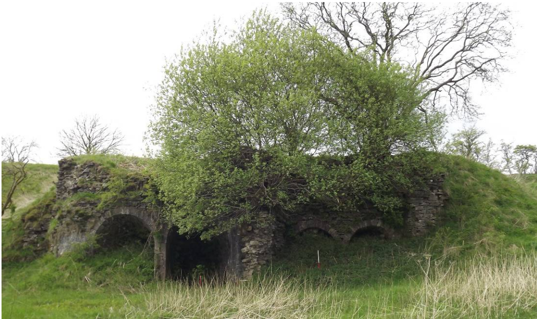
Plate 15 The SE facing elevation of Site 45
