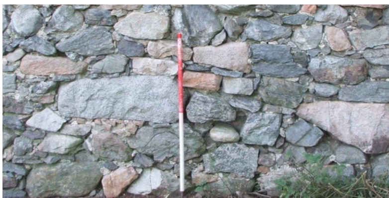
Plate 3 A typical area of masonry construction (east gable) displaying stone types present
