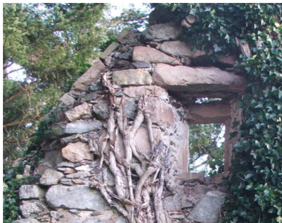
Plate 6 Interior of east gable showing detail of window and copings
