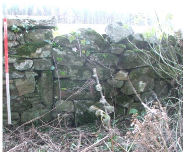
Plate 12 South wall - dry-stone masonry of existing entrance into structure towards the east end
