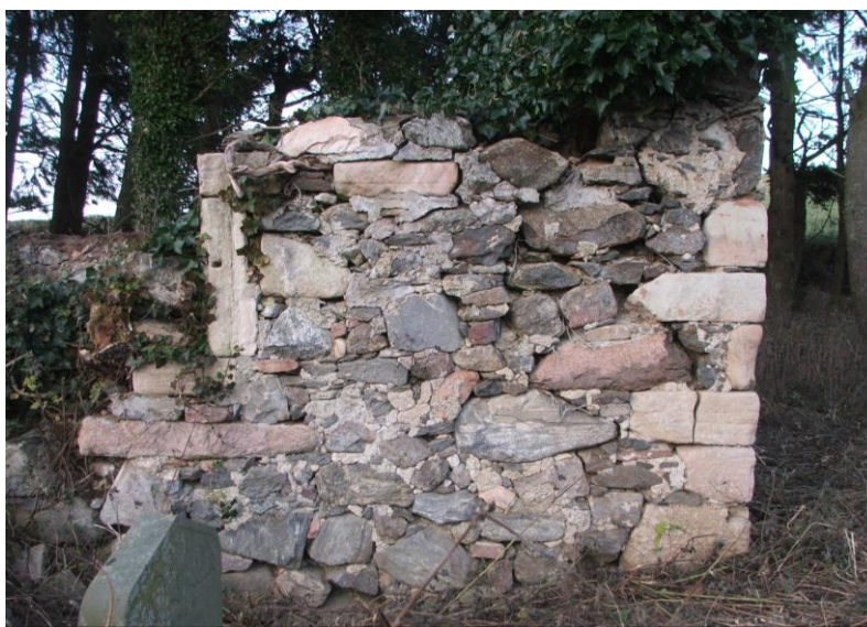
Plate 10 Remains of inserted window on at east end of south elevation and SE corner quoins
