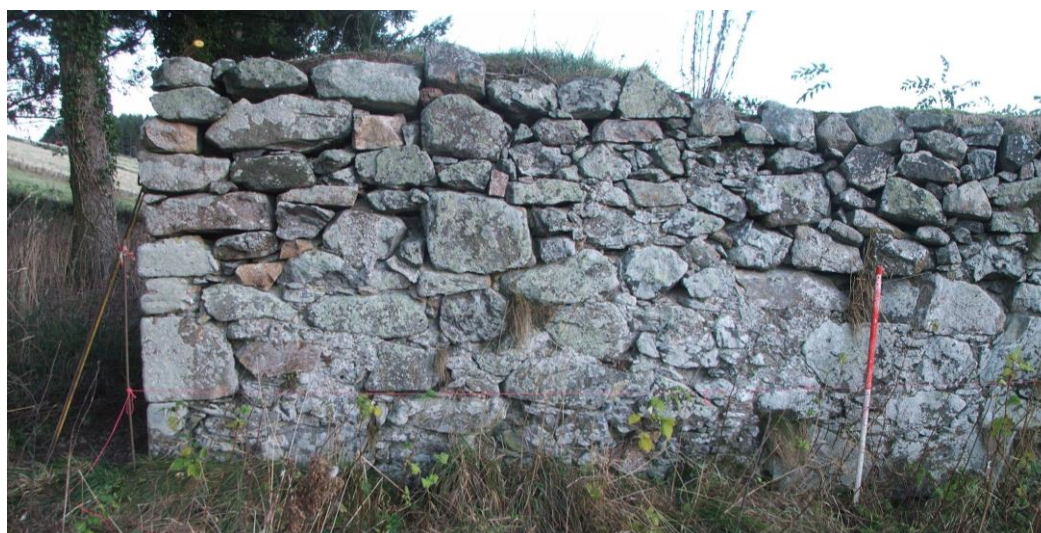
Plate 9 Detail of the NW corner of west gable, showing differing masonry
