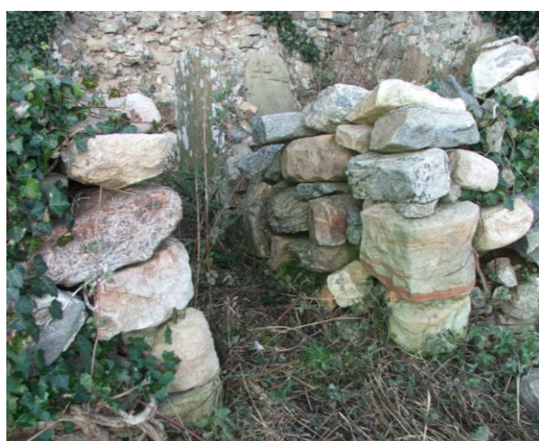
Plate 12 South wall - dry-stone masonry of existing entrance into structure towards the east end
