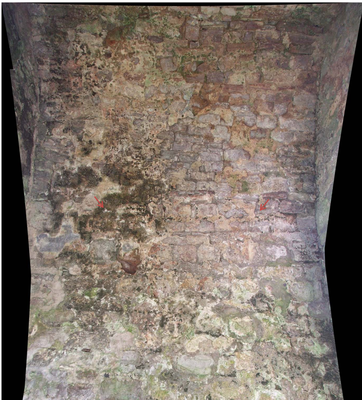
Part-rectified photographic image of the upper east wall and vault of the south transept; extensive areas of wall plaster can be seen as can zones of colouration; the horizontal band of text is indicated by the red arrows
