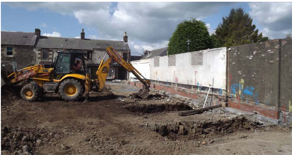
Plate 8 Digging the foundation trenches (Addyman Archaeology Photograph 121)
