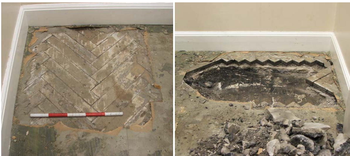
Plates 3 and 4 Parquet flooring exposed and following removal of floor to expose 202 brick floor
