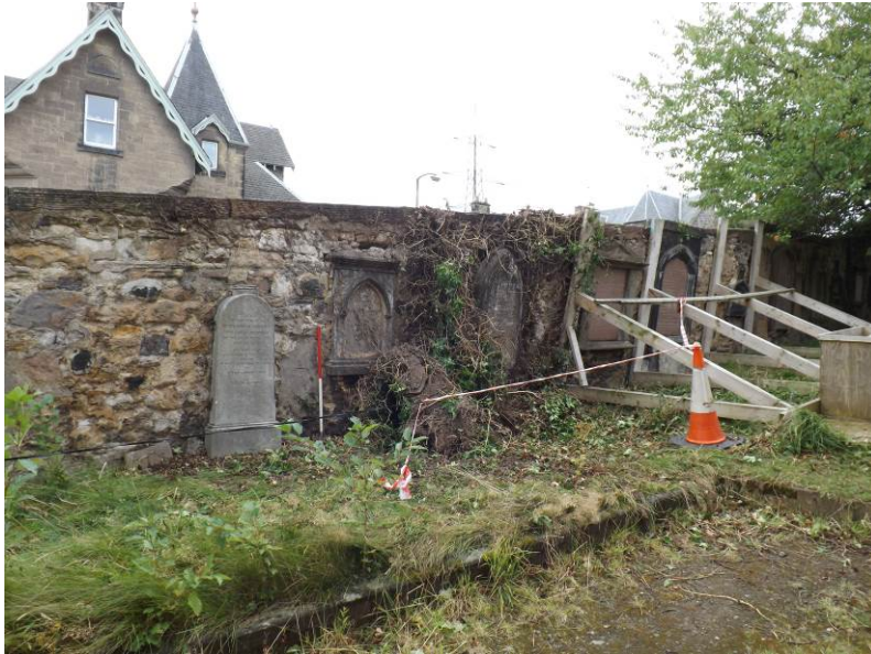
Plate 5 Collapsing wall section to be dismantled (photo 001)
