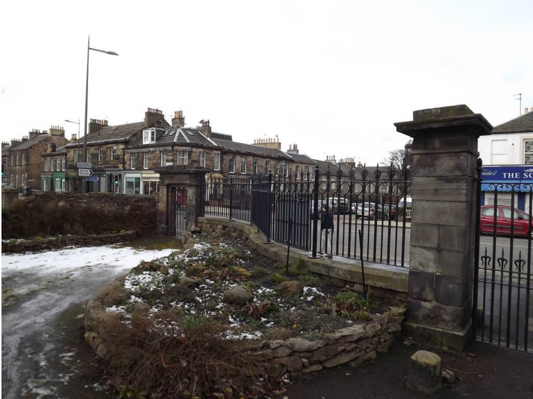
Plate 1 Northwest section of northern boundary wall showing gate and gatepiers (photo 331)
