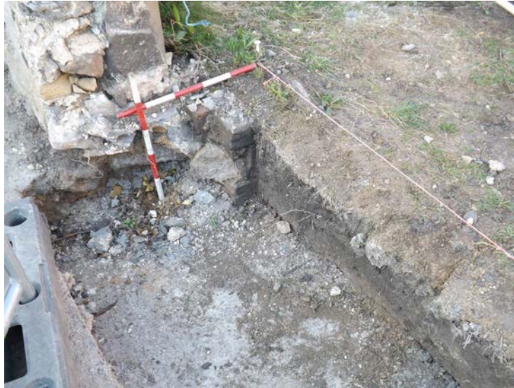
Plate 16 Trench extension pre-ex looking southwest (photo 359)
