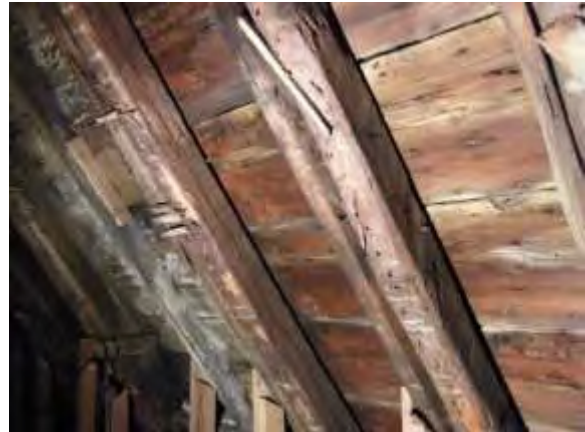
Plate 9 the carpenters' assembly mark on the northernmost surviving frame collar (for frame 'XXIII')
