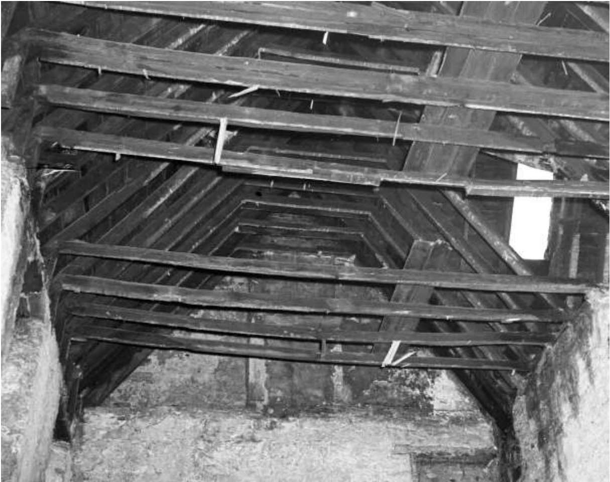
Plate 8 North end of the early roof structure of the principal range as revealed in 1956-7 following the removal of the masonry chimney stack between the main and east ranges. The hole for the chimney can be seen in the roof
