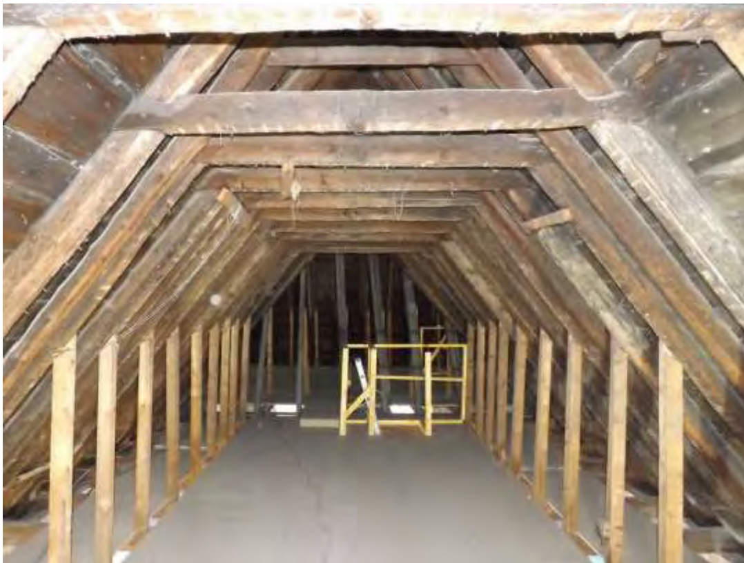
Plate 13 east jamb roof structure
