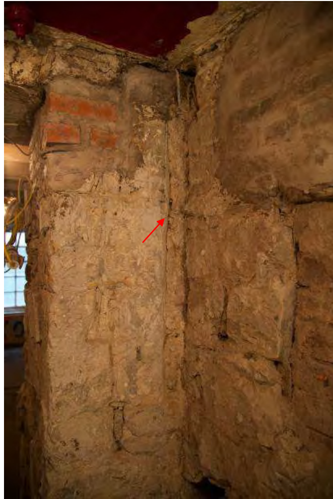
Plate 6 detail of the exterior side of window 166 (indicated), looking north
