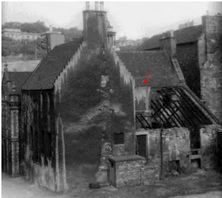
Plate 14 Photograph of c.1921 looking NNE; the upper parts of the stair tower can just be seen at the re-entrant (indicated), this in turn surrounded by a large mono-pitched lean-to infill structure.
