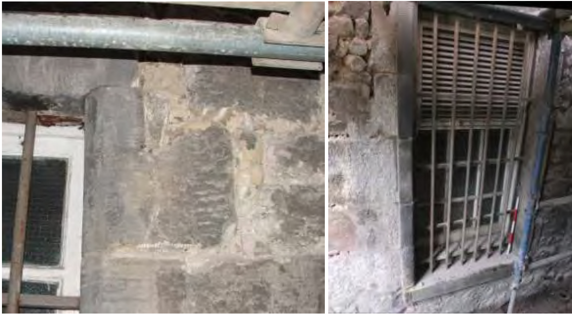
Plate 24 Window jamb 242 with window 162 cut in at top Plate 25 window 163 shows raised margins
