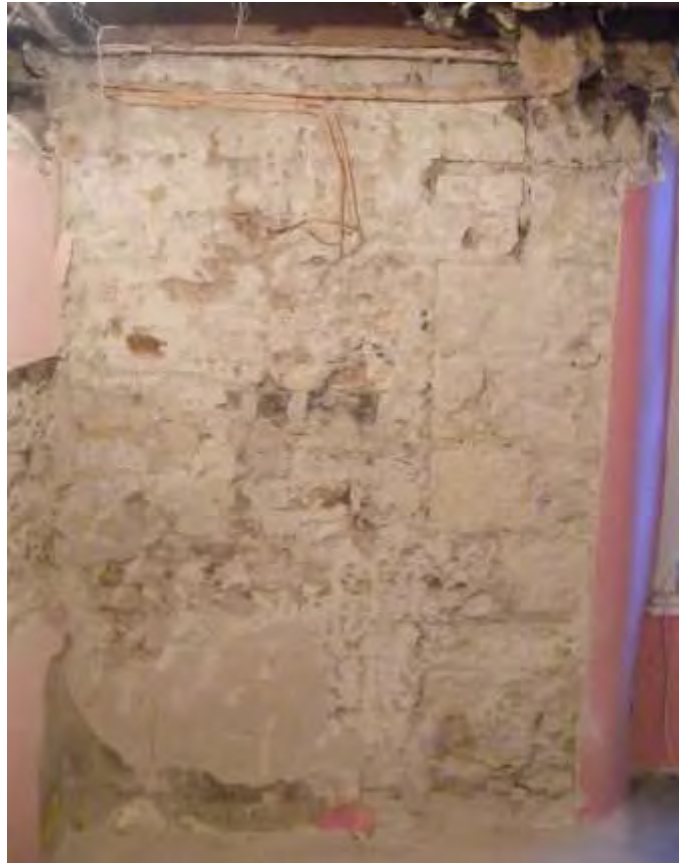
Plate 23 opening 201 (jamb to right) infilled with cemented brick 225
