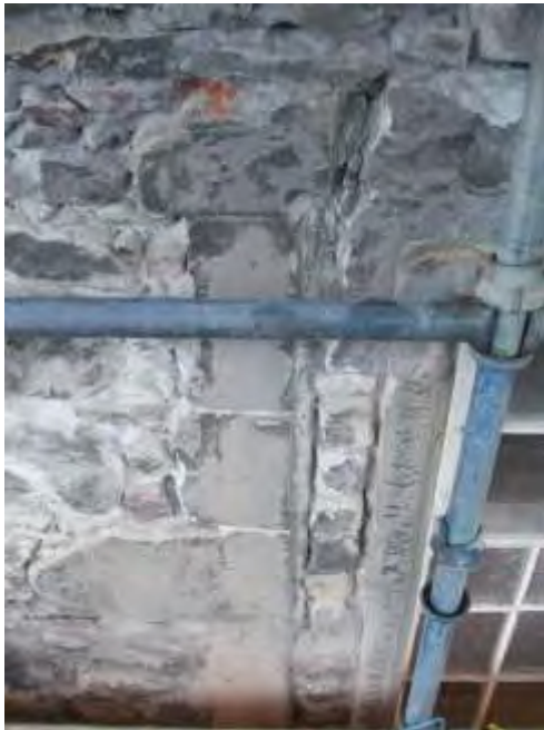
Plate 19 window 247 at left, lintel stub at top with later window 187 within
