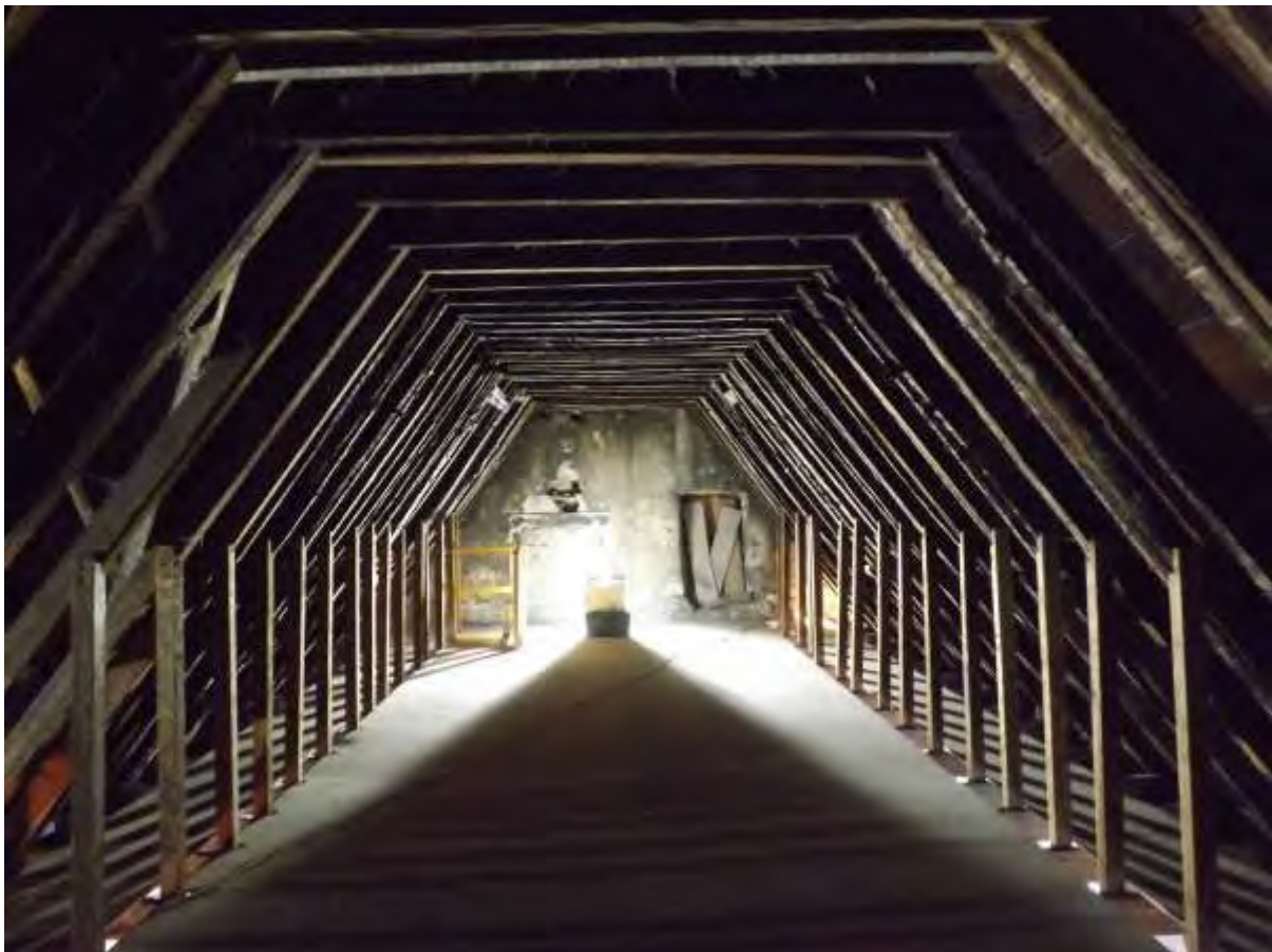
Plate 12 principal range roof structure looking south
