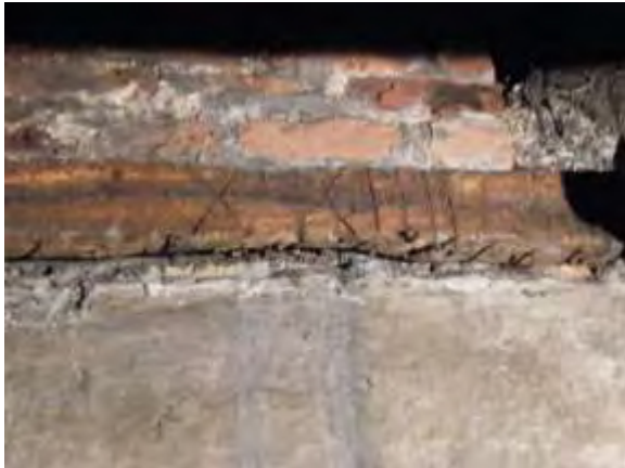
Plate 9 the carpenters' assembly mark on the northernmost surviving frame collar (for frame 'XXIII')
