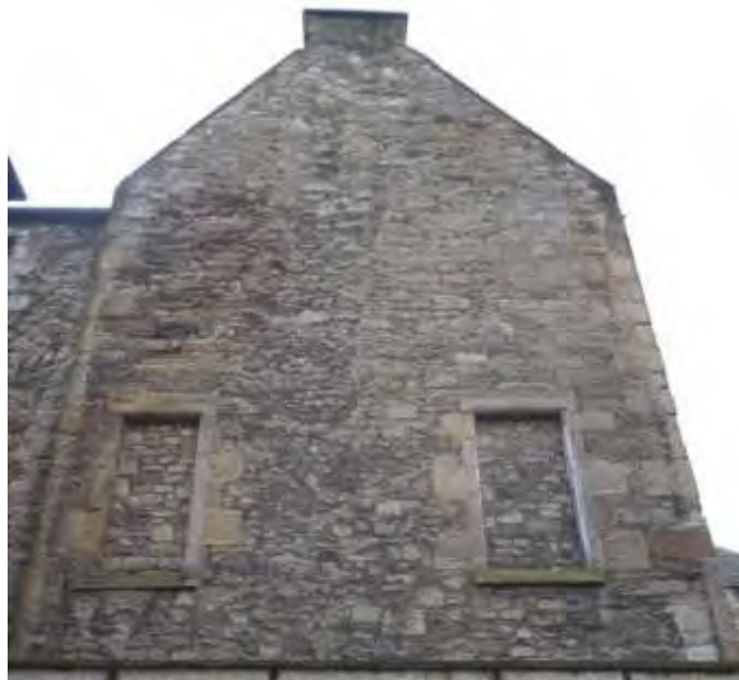
Plate 15 the existing north gable, showing extensive 19th century re-facing
