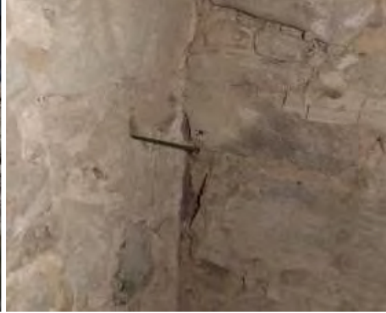
Plate 18 plaster 194 trapped behind rubble infill 196
