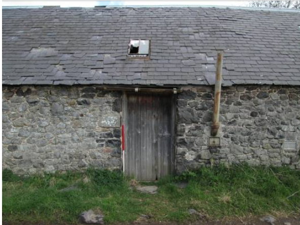
Plate 27 Workshop exterior showing 044 (041)
