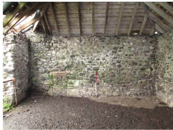
Plate 8 West interior wall (095)
