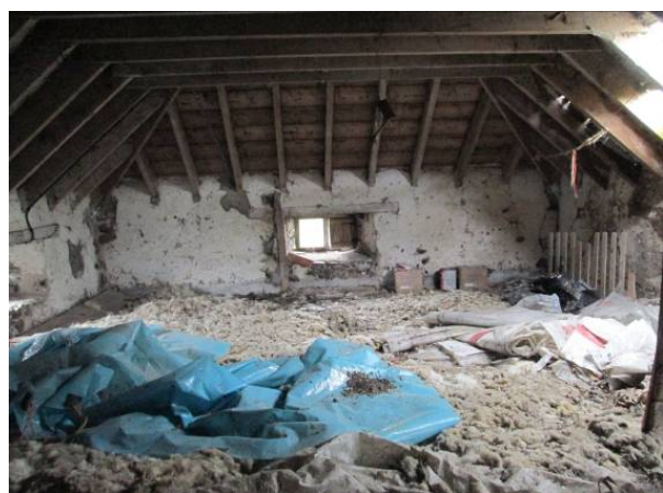
Plate 3 Area A loft looking south (175)
