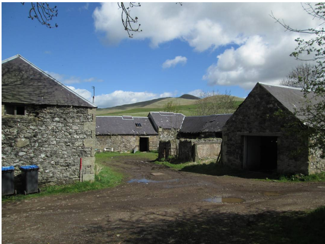
General view of the Steading looking north east
