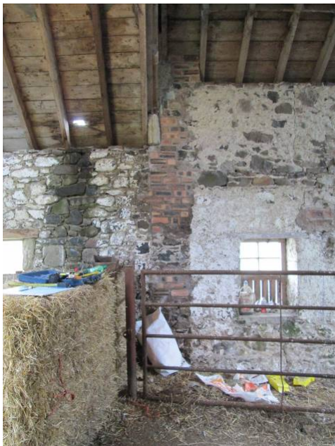
Plate 18 Mill interior looking North (120)
