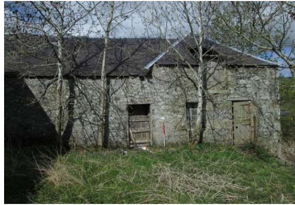
Plate 10 The East Elevation of the mill
