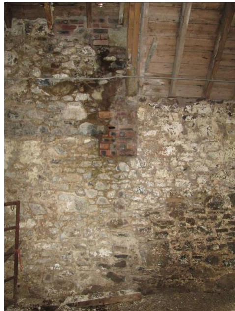
Plate 19 Mill interior looking South (103)
