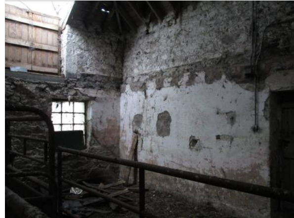
Plate 17 Mill interior showing 008 (107)
