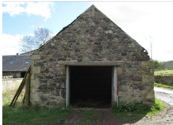
Plate 29 Area I shed exterior (045)
