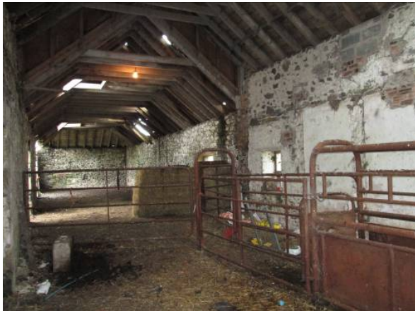
Plate 16 Mill interior looking West (114)
