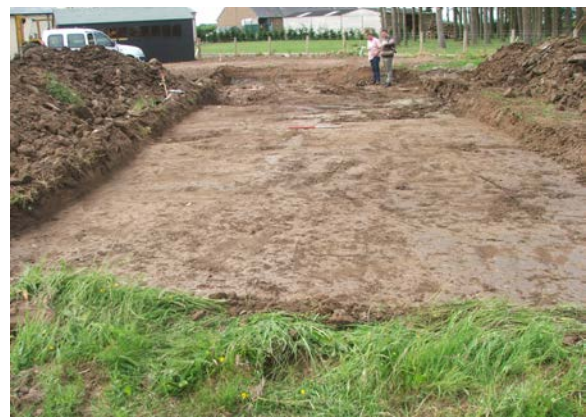
Plate 5 General view of trench following stripping ( Photograph 029 )
