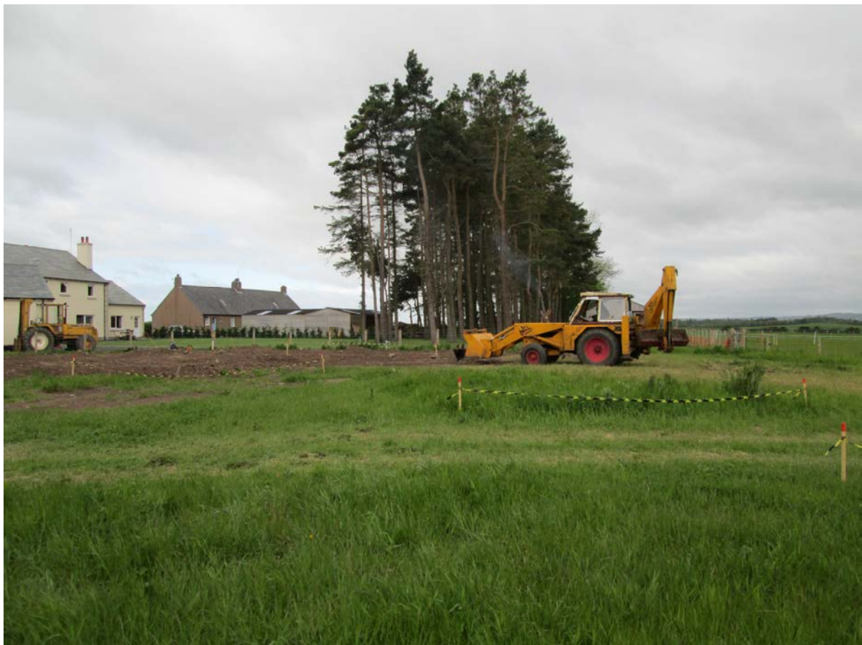
General View of the site at Blackadder West
