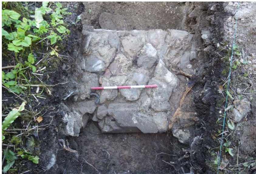
Plate 3 Wall [104] showing in-filled window and chamfered stone (at bottom of photo)
