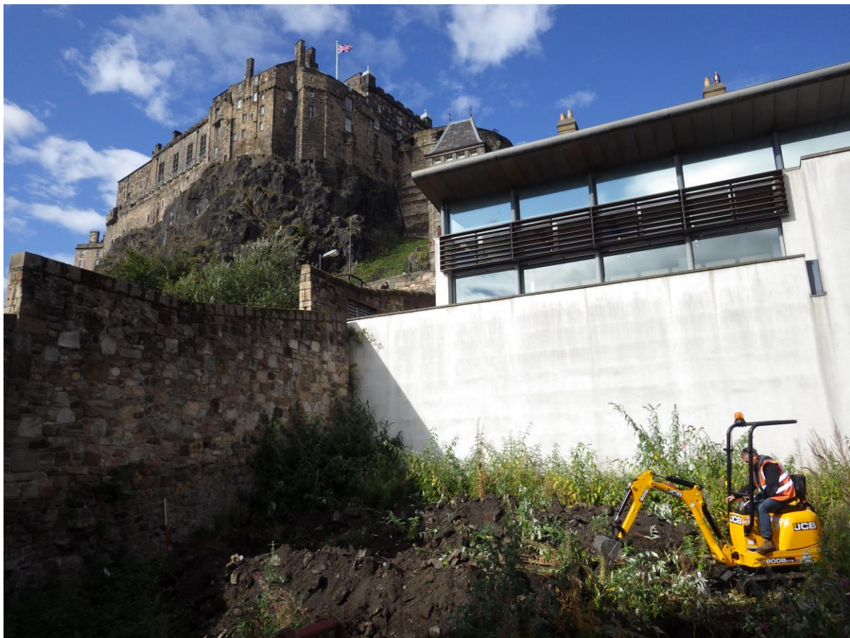
Excavation of Trench 1 (photo 007)
