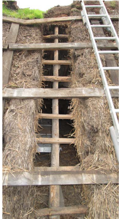
Plate 26 section through thatch
