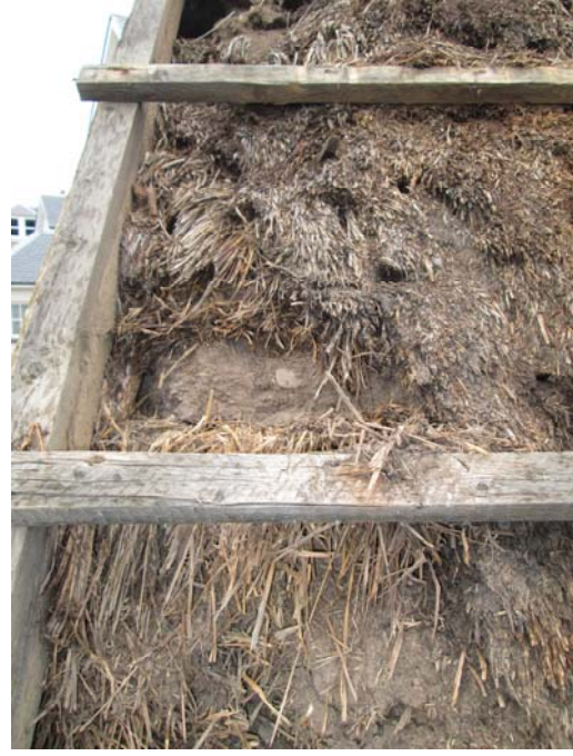
Plate 22 Turf and thatch skew, south side (173).
