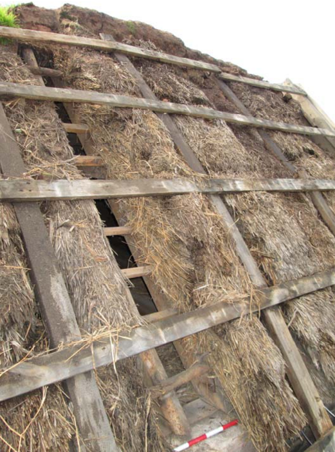
Plate 25 section through thatch
