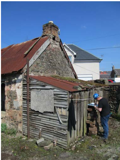
Plate 1 Working shot during initial phase (059).
