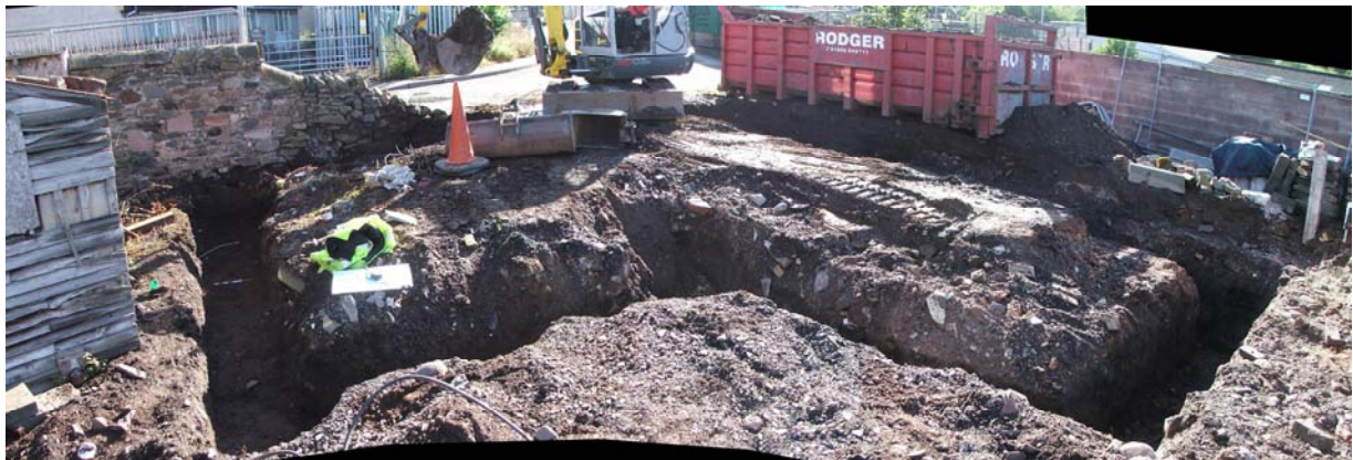
Plate 27 general view of trenching
