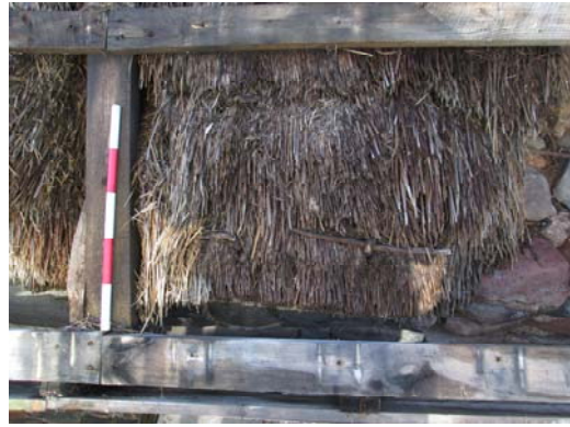
Plate 24 Scob and hazel rod holding down thatch (113).
