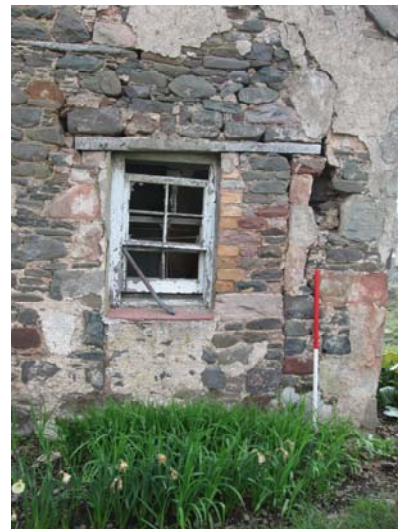
Plate 5 Detail of blocking around window (013)
