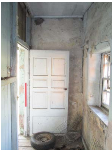
Plate 17 Bedroom looking south (050)
