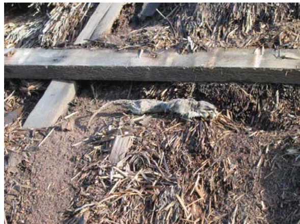
Plate 20 Rat runs within the Thatch (100).
