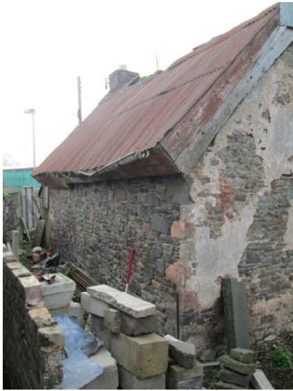
Plate 8 General view of north elevation (016)
