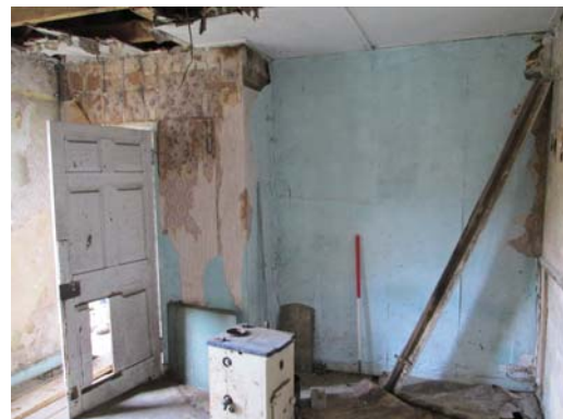
Plate 14 West elevation of main room (039)
