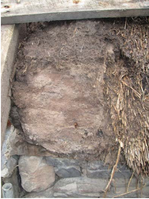
Plate 21 Turf Skew with abutting thatch north side (175).
