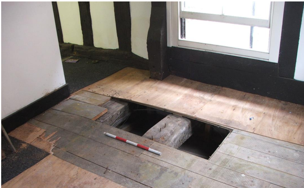
Plate 6 First floor - joisting revealed to north of stack
