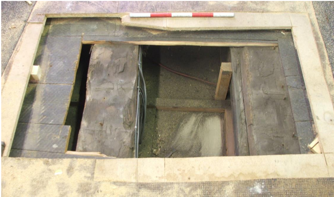
Plate 5 First floor - joisting revealed to south of stack – detail
