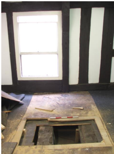
Plate 4 First floor - joisting revealed to south of stack
