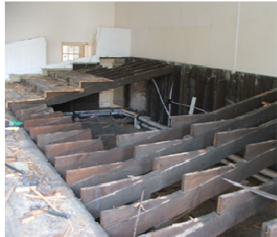
Plate 13 19 th century seating part removed showing construction
