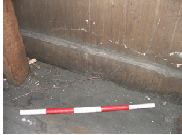
Plate 11 original skirting in situ on north elevation
