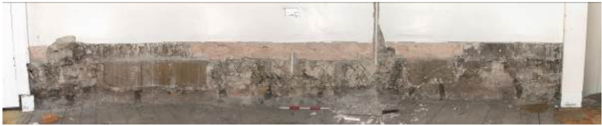
Plate 14 Room G175 east wall showing early plaster behind secondary podium
