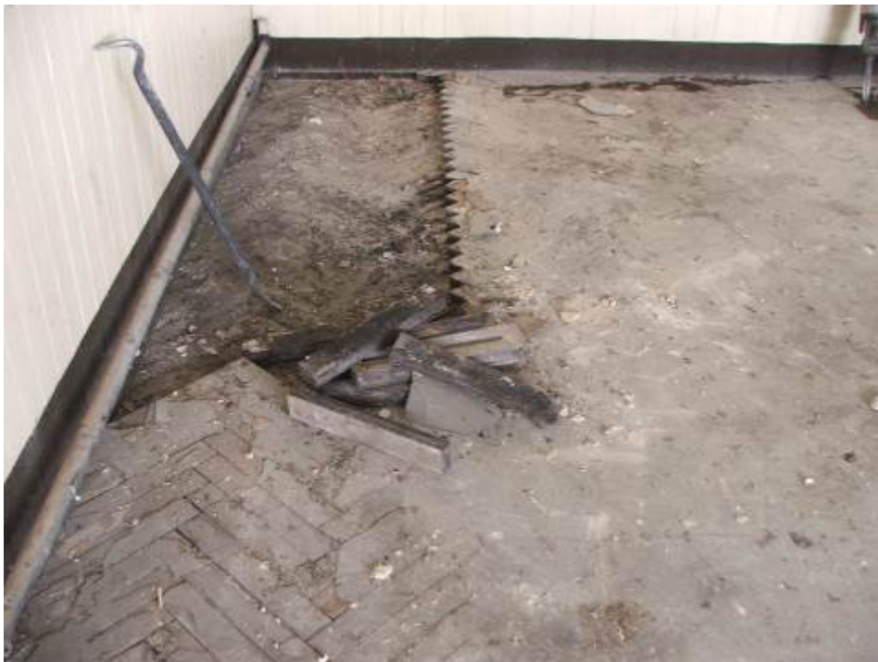
Plate 24 Herring bone floor being lifted
