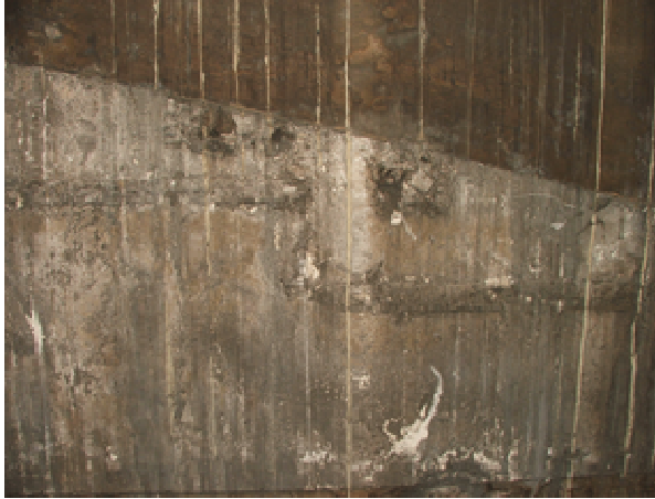
Plate 10 Impressions of timber seating in plaster on west elevation
