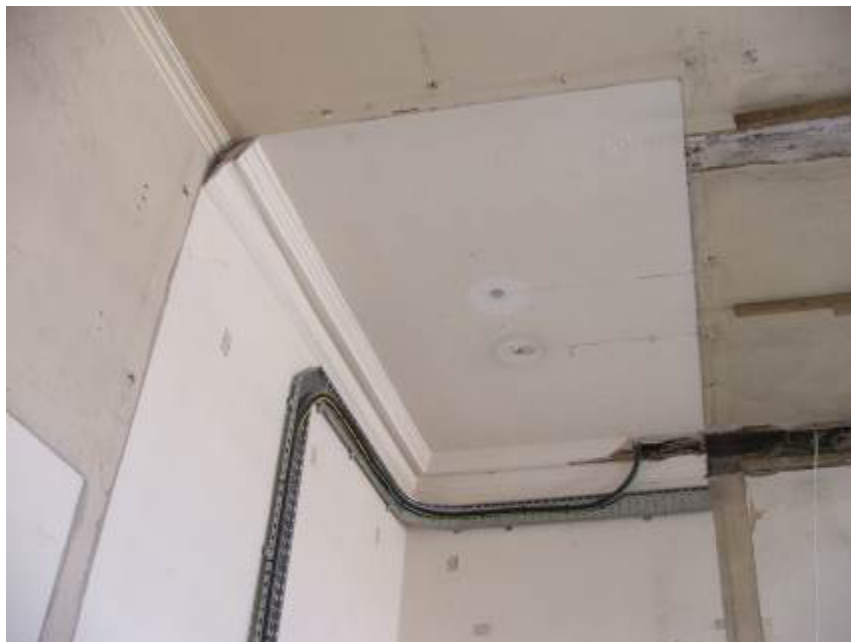
Plate 16 Secondary plaster cornice within partitioned area
