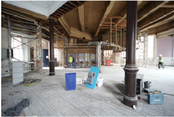
Plate 5 Columns supporting steelwork
