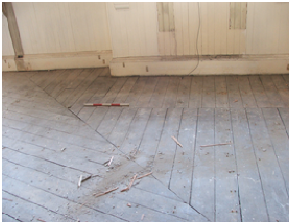
Plate 7 Diagonal edge to the floorboards of former lecture room north-east corner
