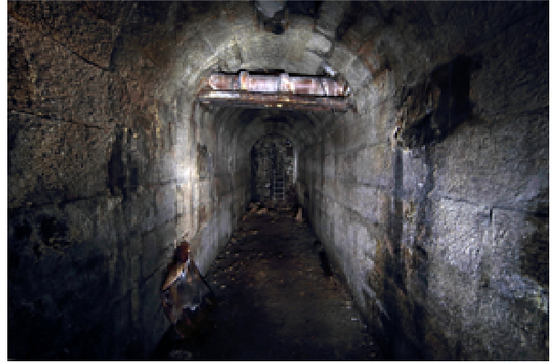
Plate 4 The tunnel looking in the opposite direction
