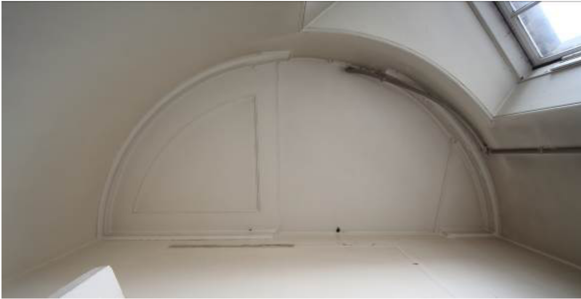
Plate 15 Infilled spiral stairwell void, middle of roof looking up
