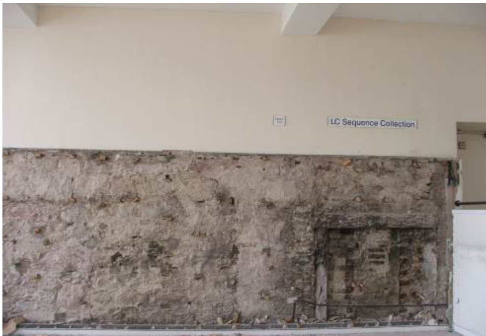
Plate 17 Room 1.274 east elevation showing fireplace
