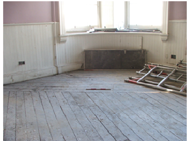
Plate 8 Diagonal edge to the floorboards of former lecture room north-west corner
