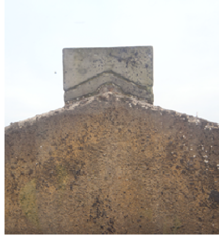
Plate 23 Rear of pediment showing former roof lines
