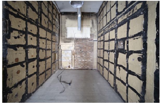
Plate 2 Ashlar elevations of room
