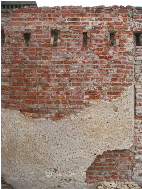
Plate 9 Early 006 brickwork with 070 joists ends cut into and partition 021 built up to /with 070 joists and flooring above
