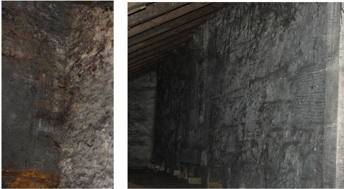
Plate 10 Window 025 and window 084 on exterior of north east stairs
