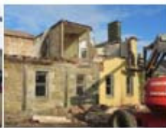
Last day of demol...
