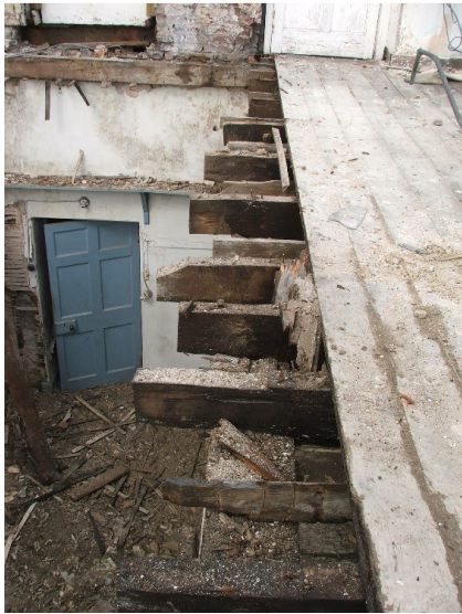
Plate 7 West joist ends of east floor 020 formerly bedded into 011
