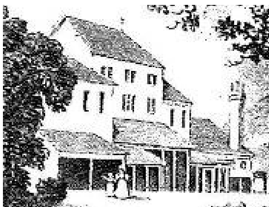
Figure 2 Lithograph of 1835 showing the south range as it had originally been built, drawn by John Clerk of Eldin – view from the south-west
