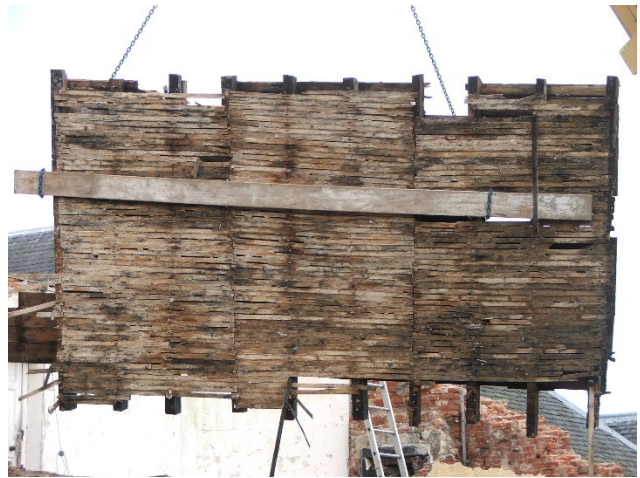
Plate 8 Floor 092 within bay 5 being lifted out in 1 piece
