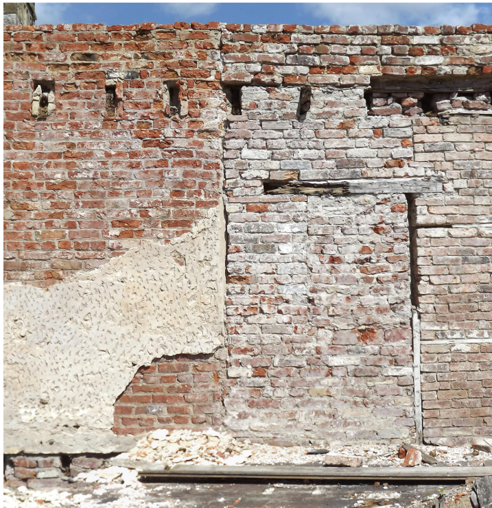
Plate 3 west end of 010 shown by plaster returning to north behind brickwork 024
