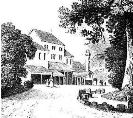
Figure 2 Lithograph of 1835 showing the south range as it had originally been built, drawn by John Clerk of Eldin – view from the south-west
