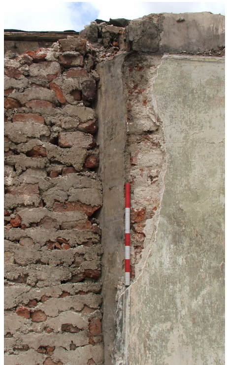
Plate 4 east end of 010 plaster behind 024 blocking and later plaster to right
