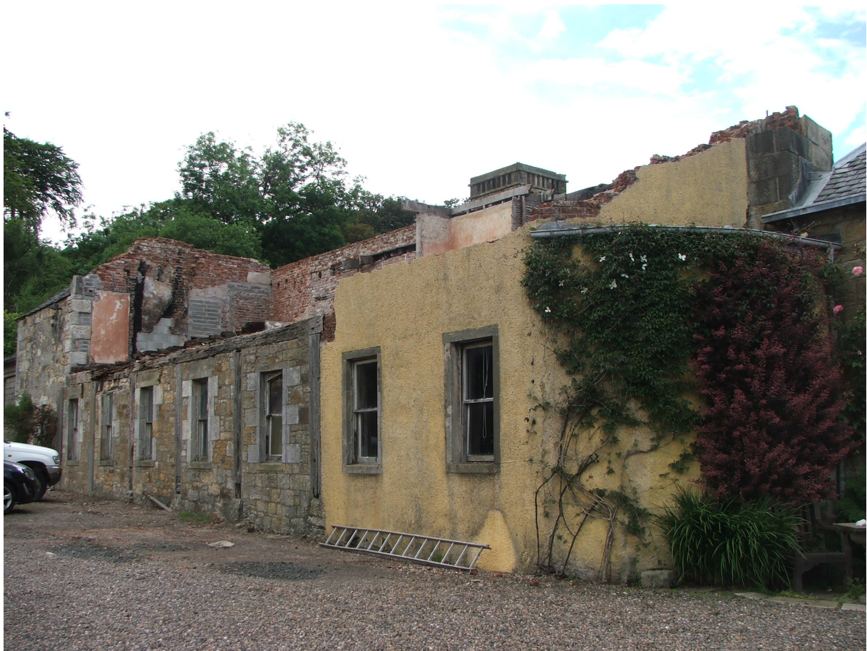
South Range during demolition. Copyright Addyman Archaeology
