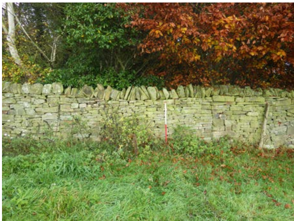
Plate 9 Site 011. Blocked former opening in northern field boundary (Photo 012).
