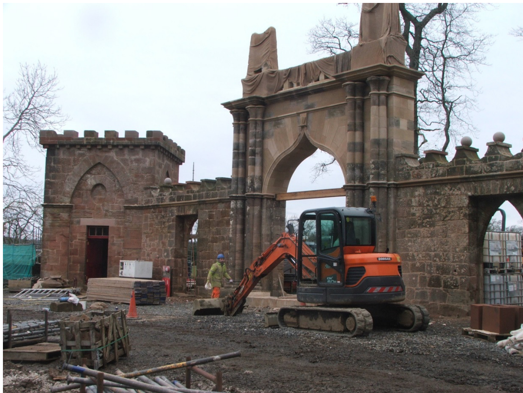
The Temple under restoration
