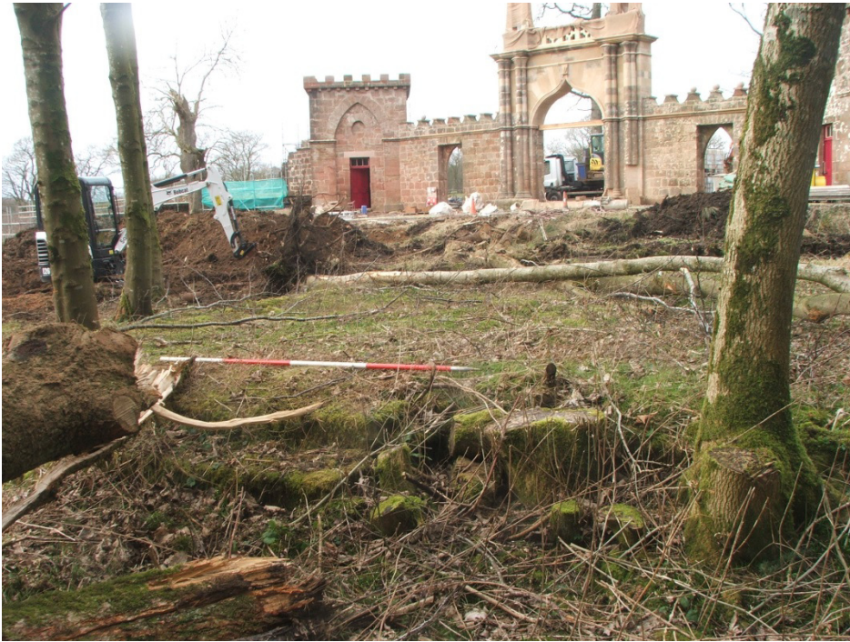
Plate 3 Steps at south end of Building [1004].
