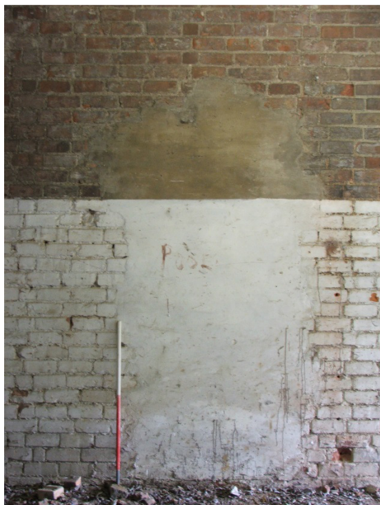
Figure 18 Blocking in southern internal elevation
