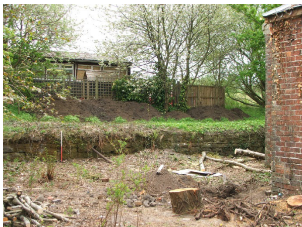
Figure 9 Platform to rear of goods shed
