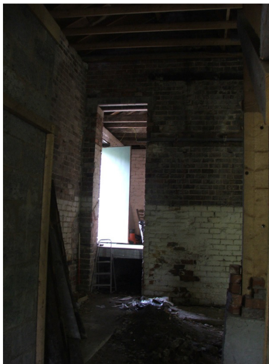
Figure 19 View into office from shed
