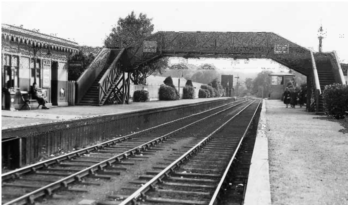
Figure 2 View of Currie station looking west. Water tank (directly under bridge) is located on northern boundary of site. ©RCAHMS
