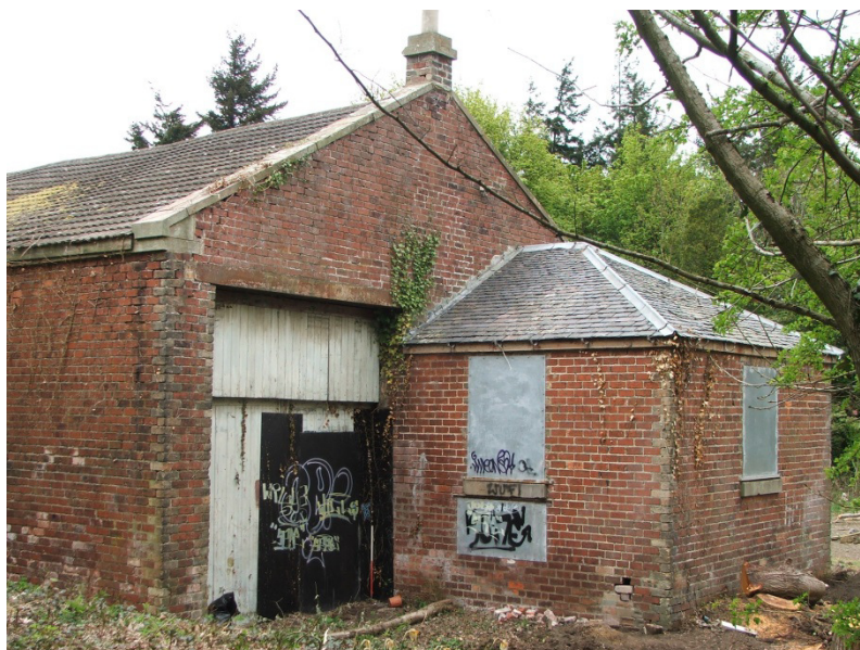
Figure 15 East elevation and office block, looking north-west
