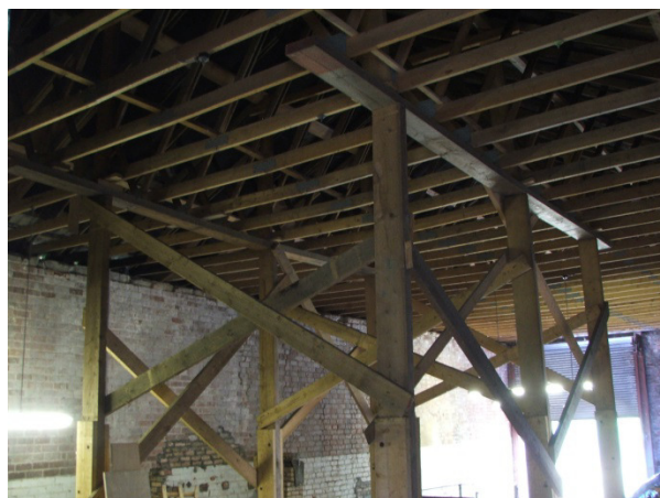
Figure 10 Timber propping up modern roof
