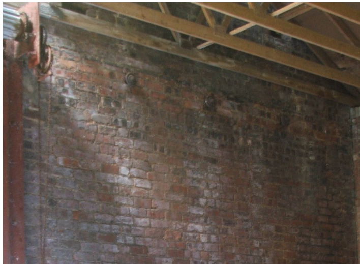
Figure 17 Iron bosses to right of roller shutter on west internal elevation
