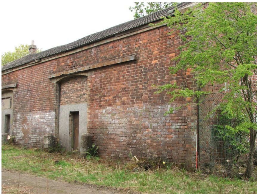
Figure 12 Western blocked archway, looking south-east
