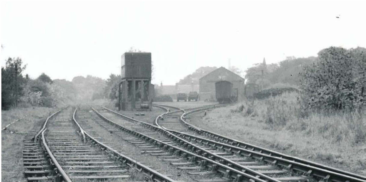
Figure 3 View of Currie sidings looking east after removal of the footbridge and station. The Goods station is on the right with the water tank in the centre of the picture. ©RCAHMS
