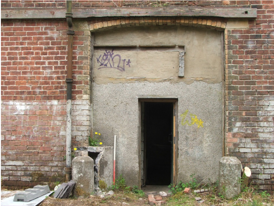
Figure 11 Eastern blocked archway in northern elevation
