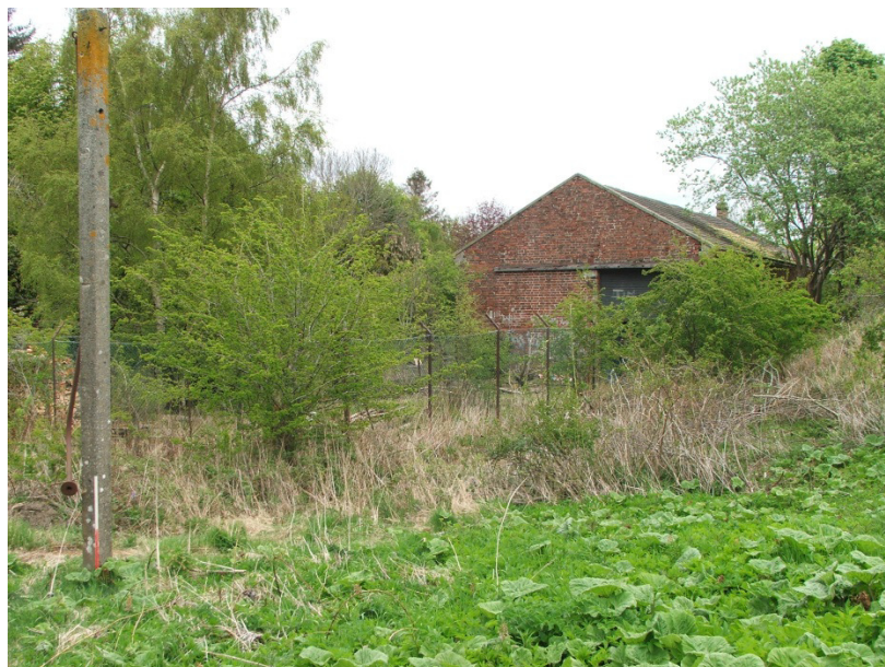
Figure 23 View of concrete pole looking towards west end of goods shed
