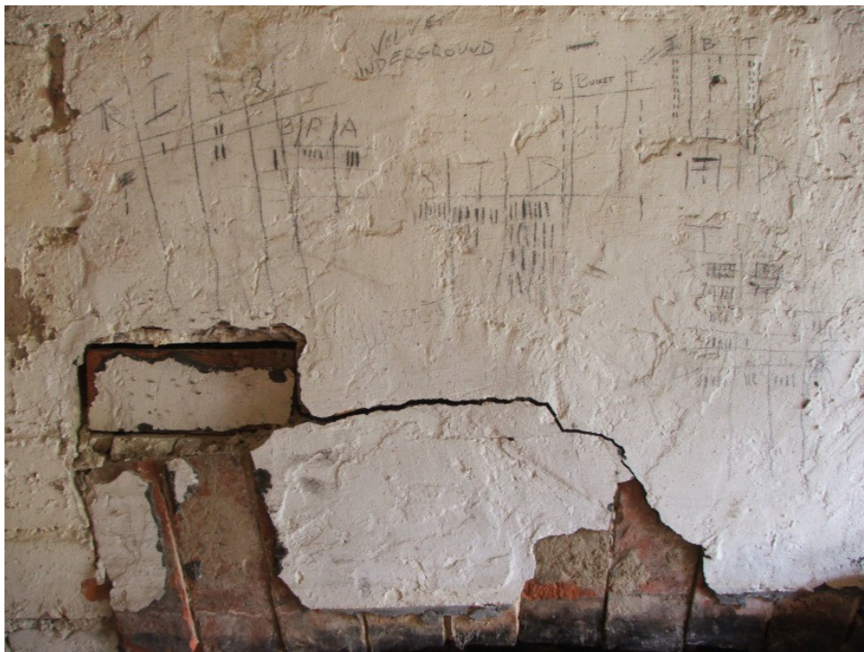
Figure 22 Graffiti above fireplace
