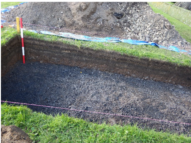
Plate 21 Trench 4, general view south end post-excitation. Facing north-west.
