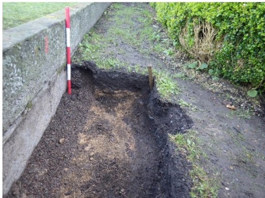
Plate 13 Trench 2, detail of far south end showing parterre garden path (208) and planting bed deposit (209) Facing NW.
