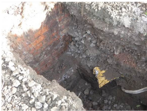
Plate 14 TP7 Building foundation (photo 039)
