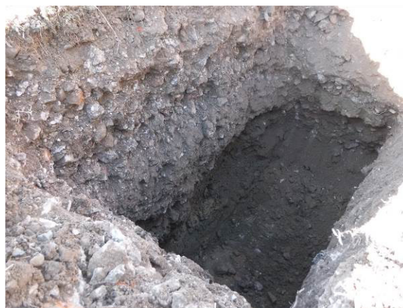
Plate 2 TP1 Northeast facing section (photo 019)
