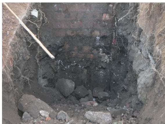
Plate 16 TP8 Foundation base detail (photo 043)
