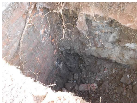
Plate 15 TP8 Wall foundation (photo 041)
