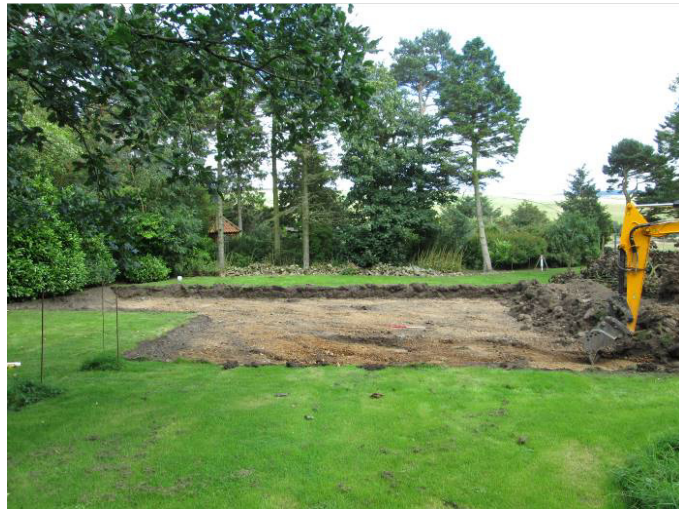
Plate 1 Area after stripping looking east 008
