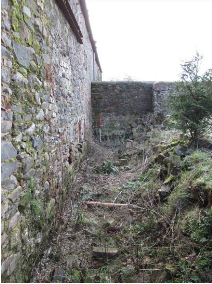
Plate 3 Former mill lade looking south (photo 012)
