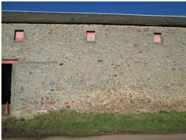
Plate 12 Exterior elevation of south range showing different phases (photo 103)
