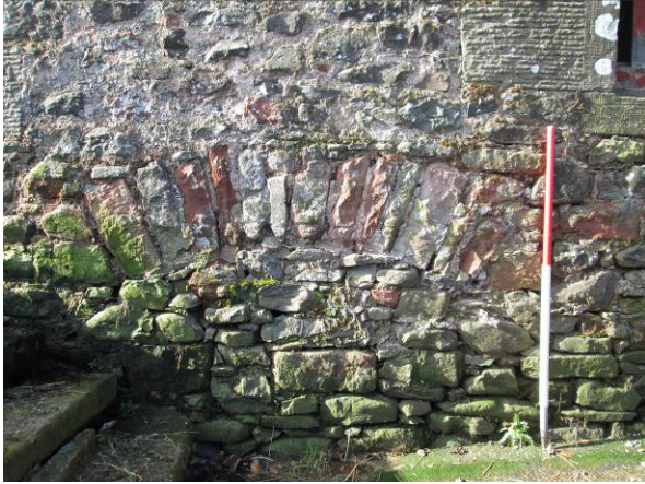
Plate 8 Relieving arch on west range, beside steps (photo 065)
