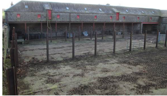
Plate 11 Interior/courtyard elevation, south range (photo 127)
