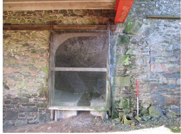
Plate 9 Partially blocked cartshed opening, south and west range (photo 058)
