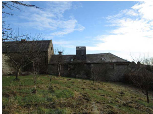
Plate 2 Lower part of west range, from west (photo 001)
