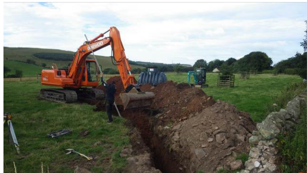
Plate 18 Excavation of the septic tank pit (photo 241)
