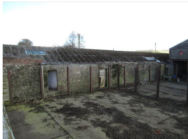
Plate 14 Interior/courtyard elevation of east range (photo 126)
