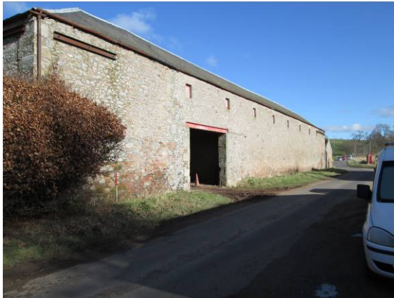
Plate 10 Exterior elevation, south range (photo 096)
