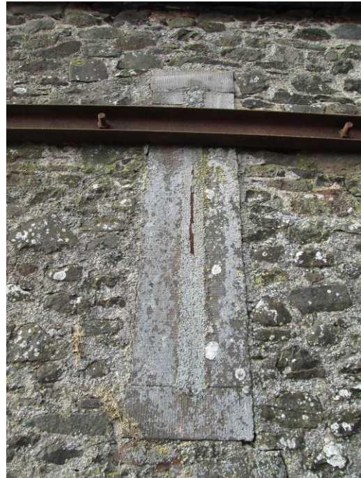
Plate 6 Ventilation slit on east elevation (photo 027)
