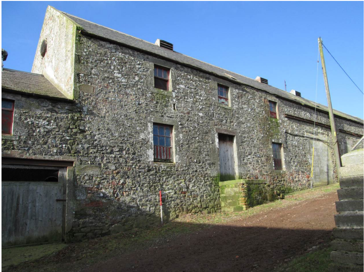
West Range, East Elevation (photo 045)
