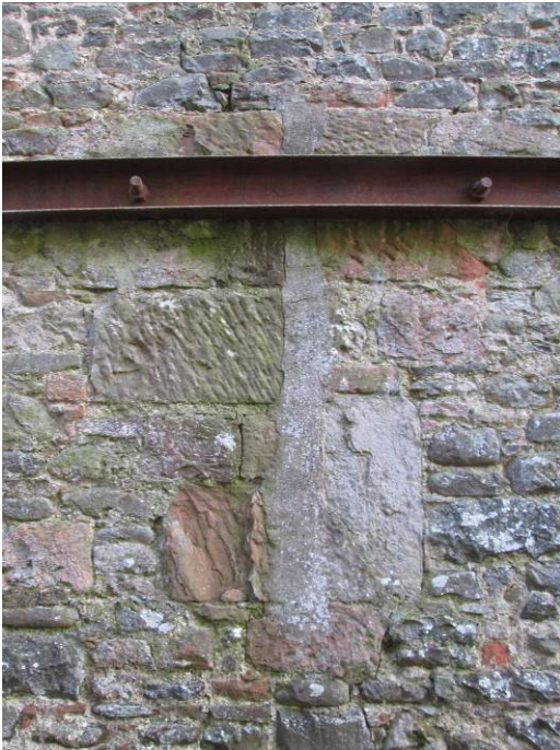
Plate 5 Ventilation slit on west elevation (photo 021)
