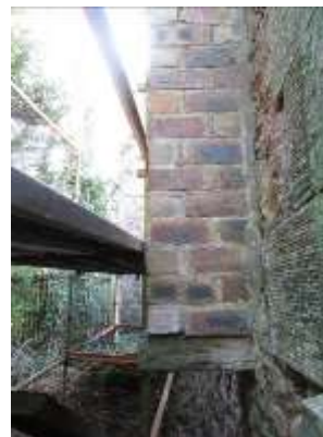
Plate 8 Chimney supported on slab
