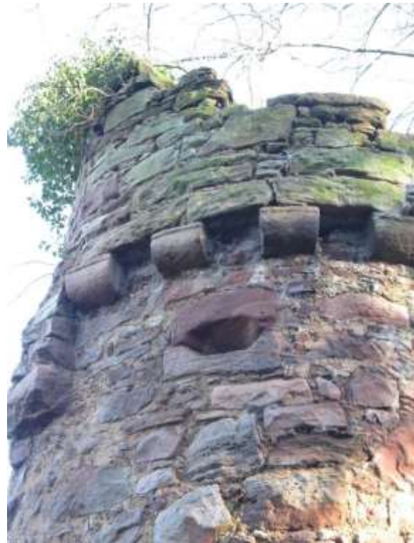
Plate 2 Detail of parapet and gun port 2208 042
