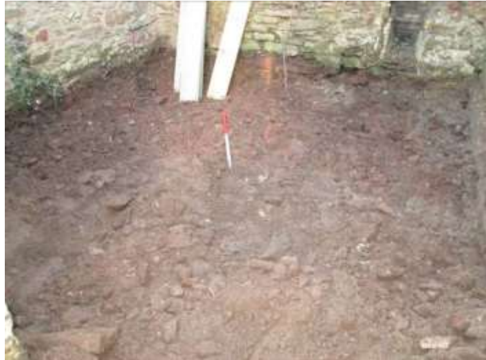
Plate 13 North room of east wing following ground reduction 2208 250
