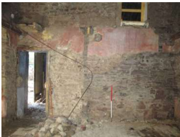
Plate 11 Outline of timber stall on east wall 2208 123
