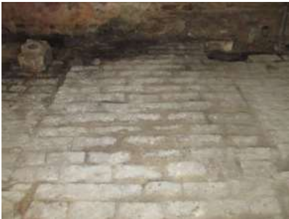
Plate 9 Cobbled stable floor looking north 2208 134
