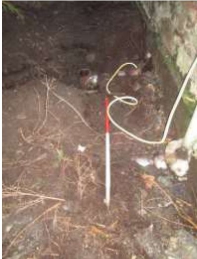
Plate 12 Hand excavated area showing drains 2208 217
