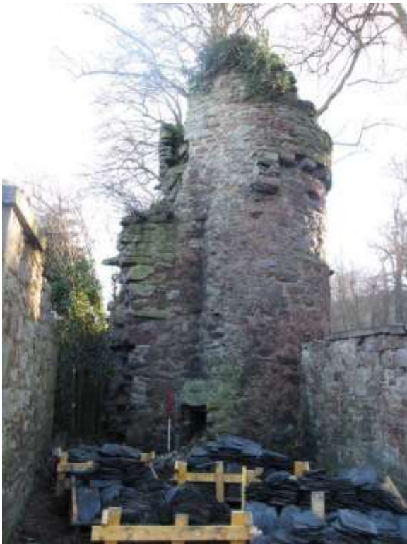
Plate 1 General view of tower looking east 2208 031
