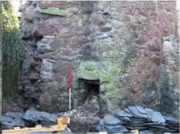
Plate 4 Blocked opening into dovecot 2208 030
