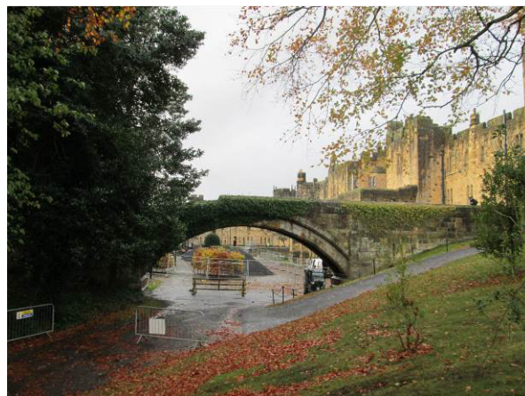
Plate 4 View from east side below Duchess Bridge
