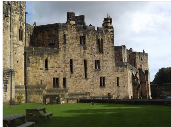
Plate 8 West facing elevation
