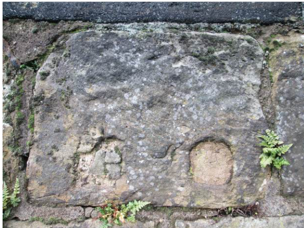
Plate 12 Possibly reused stones in retaining wall
