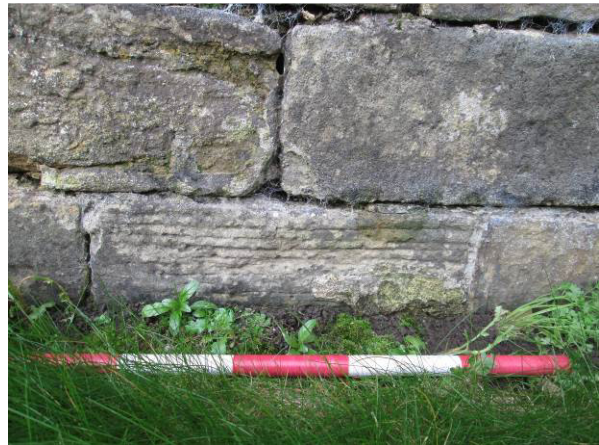
Plate 13 Possibly reused stones in retaining wall
