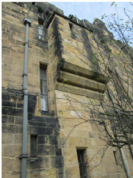
Plate 10 20 th century window insertion in south facing elevation
