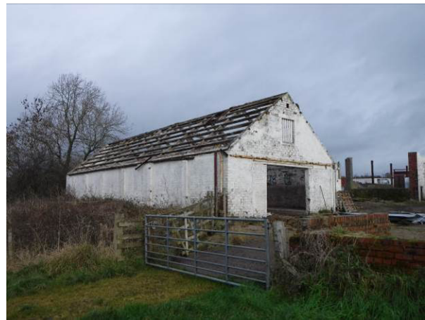
Plate 19 : Building 7, from south west (photo 133)
