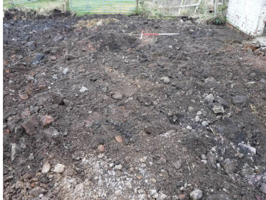
Plate 67 : Post-concrete removal, South of Building 7 (photo 352)
