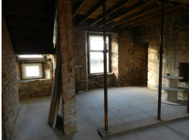
Plate 33 : Building 8, Store and Kitchen (photo 579)
