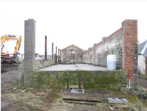
Plate 10 : Building 2, Room C, west elevation (photo 081)
