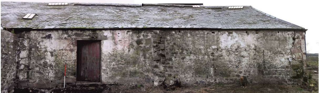
Plate 49 : Building 8, Byre, north-facing elevation (photo 291-4)
