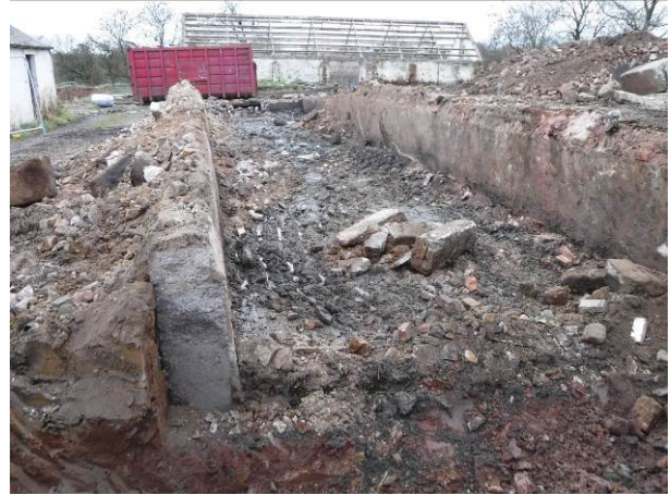
Plate 59 : Building 2, Concrete skin below Room C (photo 273)
