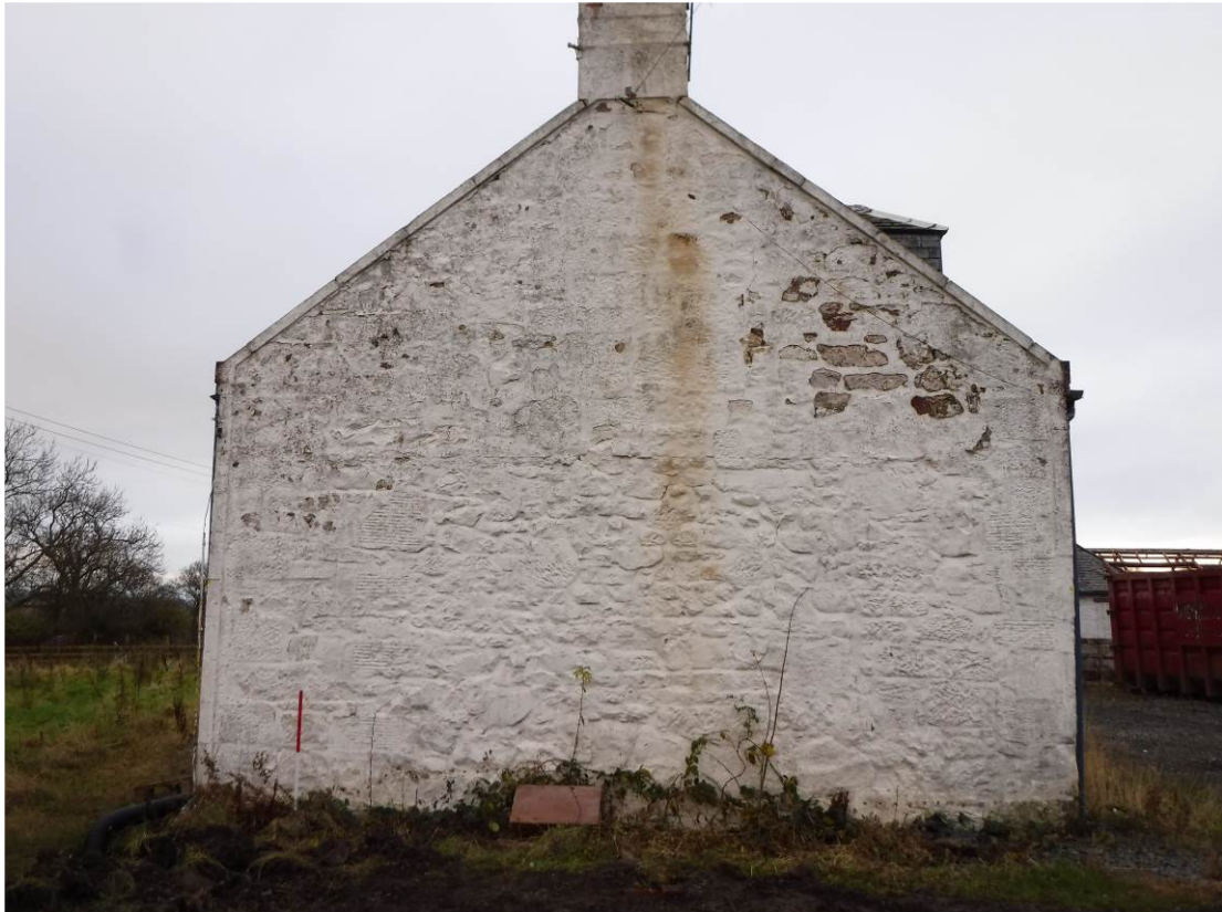
Plate 28 : Building 8, Farm House, east gable (photo 409)
