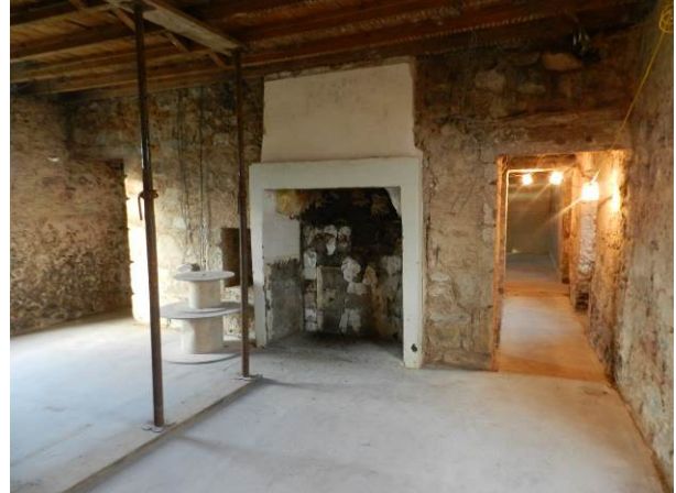
Plate 34 : Building 8, Kitchen (photo 580)
