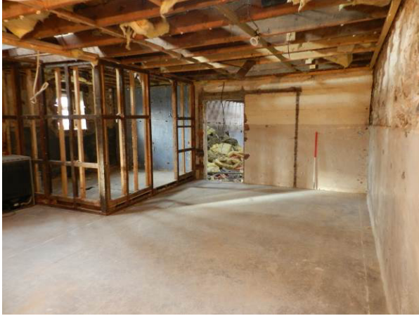
Plate 39 : Building 8, Family Room (photo 649)
