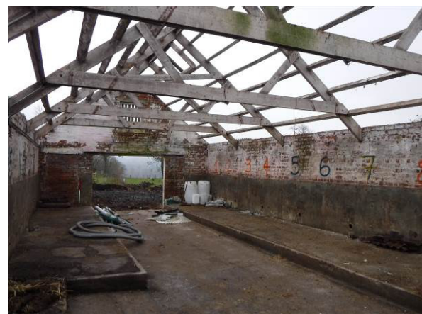
Plate 21 : Building 7, interior (photo 360)
