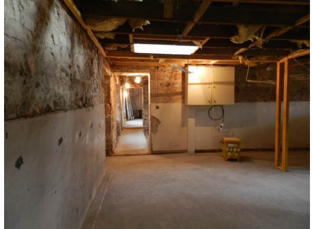
Plate 40 : Building 8, Family Room (photo 654)
