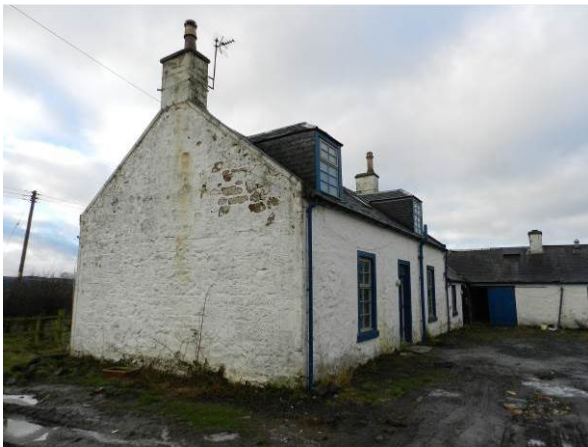
Plate 26 : Building 8, Farm House, east gable (photo 719)
