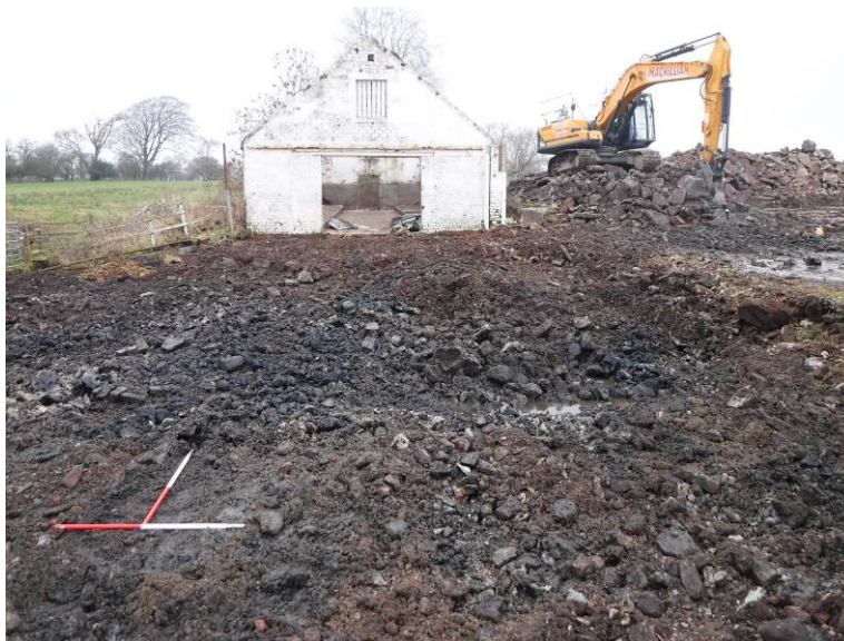
Plate 66 : Structure 9, post-demolition (photo 346)
