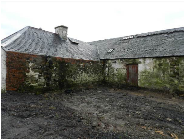
Plate 24 : Building 8, Bothy, Store, Byre (photo 716)
