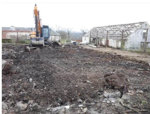
Plate 57 : Structure 1, post-demolition (photo 140)
