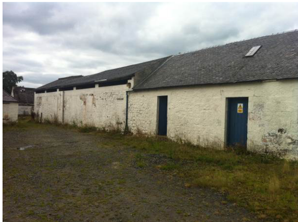
Plate 3 : Building 2, south elevation (photo 470)
