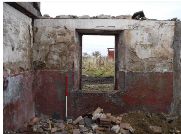
Plate 8 : Building 2, Room B, south facing interior (photo 073)
