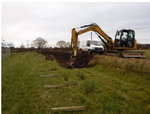
Plate 68 : Road Widening, mid-ex (photo 402)
