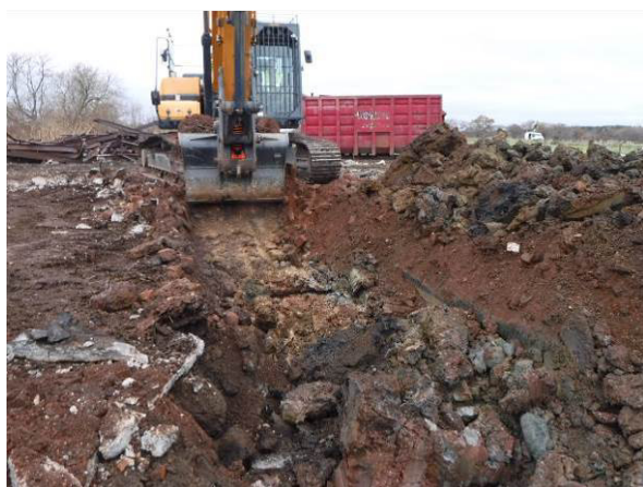
Plate 56 : Structure 1, mid-demolition (photo 019)
