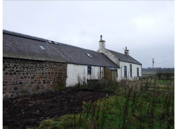
Plate 53 : Building 8, south-facing elevation (photo 368)
