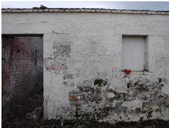
Plate 5 : Building 2, Room A, south facing exterior (photo 029)
