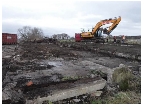
Plate 2 : Structure 1, concrete slab (photo 012)
