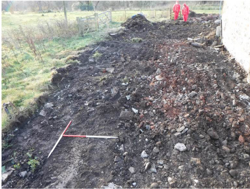
Plate 62 : Structure 5, post-demolition (photo 327)
