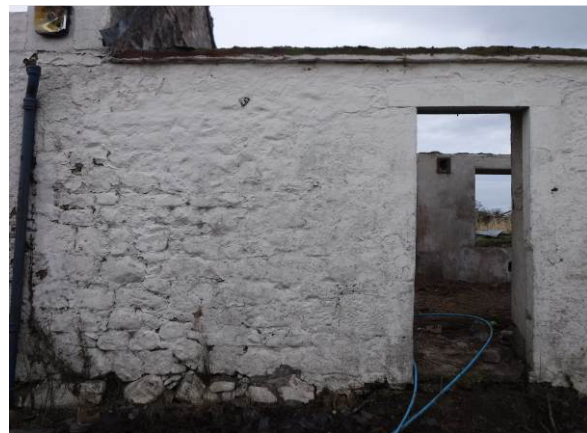
Plate 7 : Building 2, Room B, south facing exterior (photo 032)
