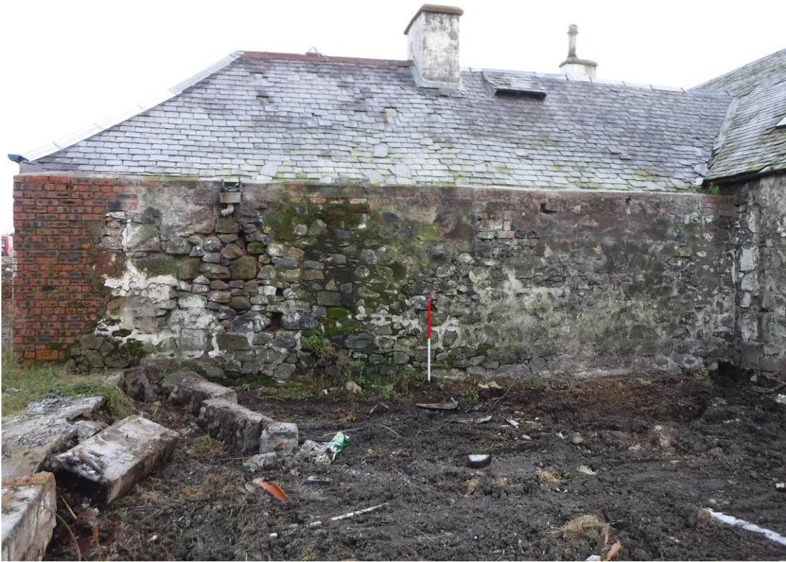
Plate 48 : Building 8, Bothy and Store, west-facing elevation (photo 287)
