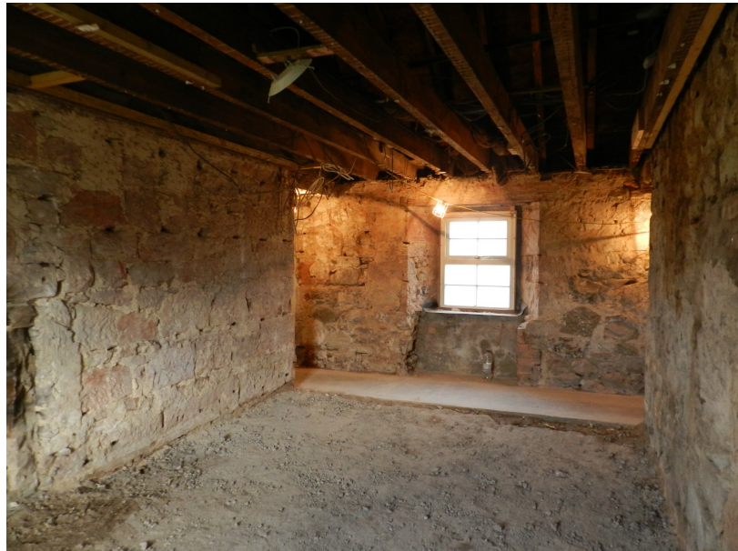
Plate 38 : Building 8, Dining Room, north wall (photo 621)
