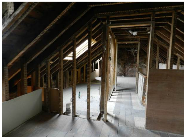
Plate 43 : Building 8, Box Room/Landing (photo 696)
