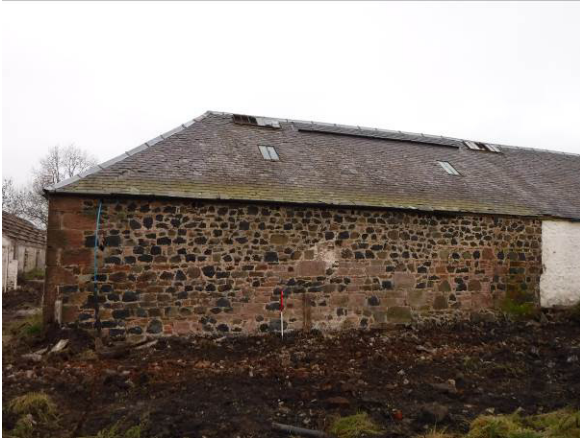
Plate 52 : Building 8, Byre, south-facing (photo 367)
