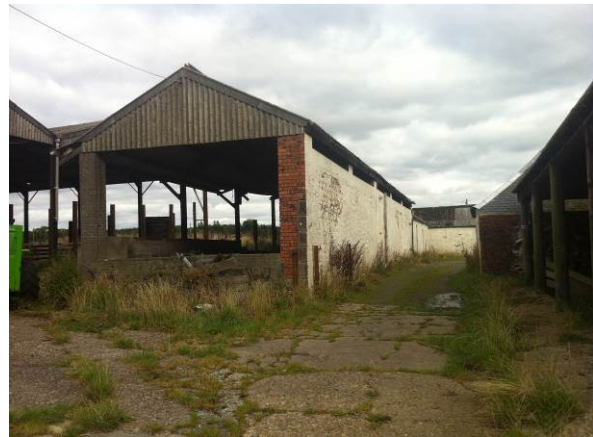
Plate 4 : Building 2, from southwest (photo 477)
