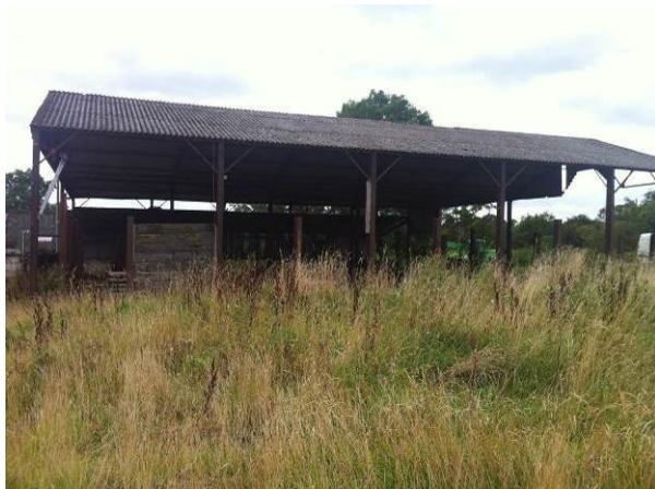
Plate 1 : Structure 1, from east (photo 484)
