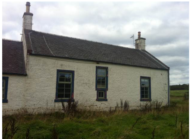
Plate 27 : Building 8, Farm House, south elevation (photo 493)
