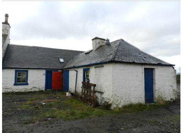
Plate 23 : Building 8, Bothy and Store (photo 711)
