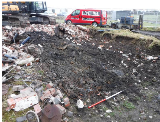
Plate 60 : Building 3, post-demolition (photo 147)
