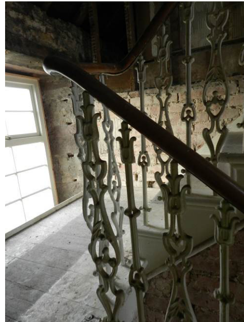
Plate 32 : Building 8, Stair (photo 673)
