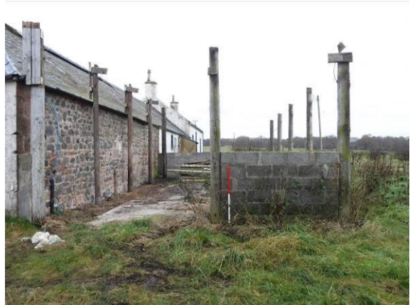
Plate 17 : Structure 5, from west (photo 236)
