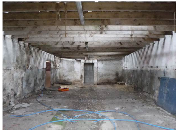
Plate 51 : Building 8, Byre interior (photo 365)
