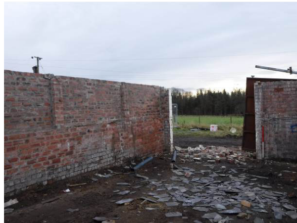
Plate 13 : Building 3, interior (photo 126)
