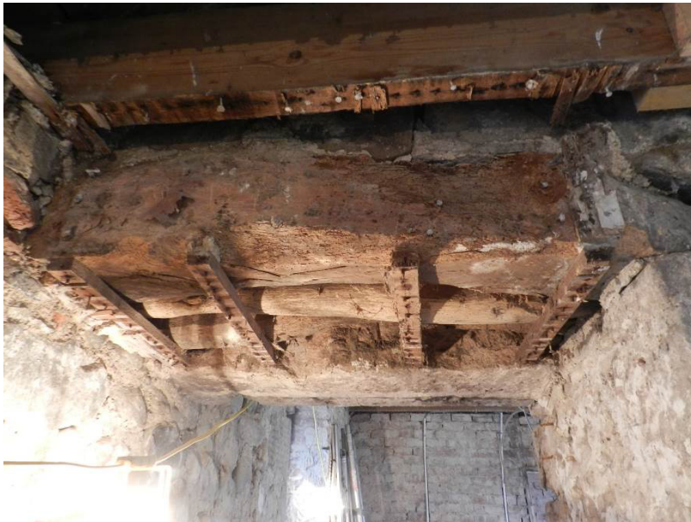
Plate 35 : Building 8, Wood lintels east of Kitchen (photo 616)
