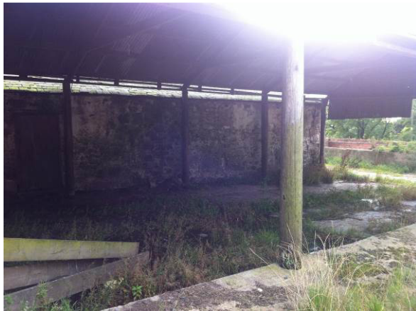
Plate 14 : Structure 4, superstructure (photo 475)
