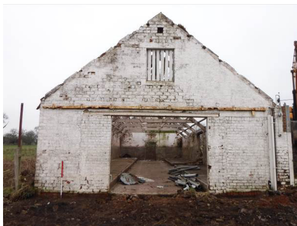
Plate 20 : Building 7, south gable (photo 354)
