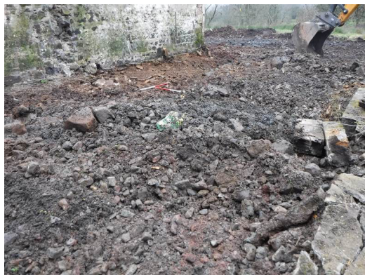
Plate 61 : Structure 4, post-demolition (photo 393)
