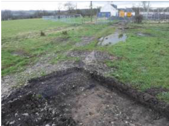
Plate 30 : Trench 10, Trackway (photo 255)
