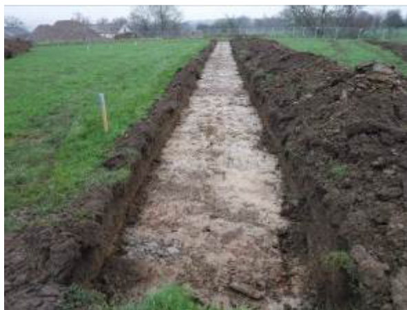
Plate 13 : Trench 5, Overall, Facing WSW (photo 168)
