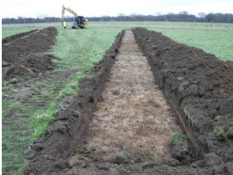
Plate 37 : Trench 12, Overall, Facing ENE (photo 419)
