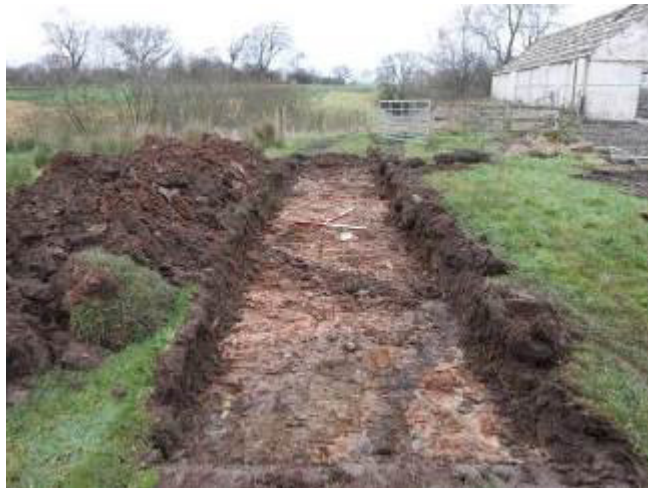
Plate 35 : Trench 11, Overall, Facing northwest (photo 329)
