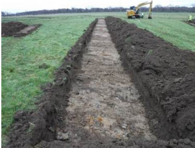
Plate 40 : Trench 13, Overall, Facing northeast (photo 366)
