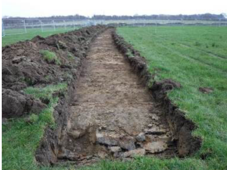
Plate 2 : Trench 1, Overall, Facing northeast (photo 011)
