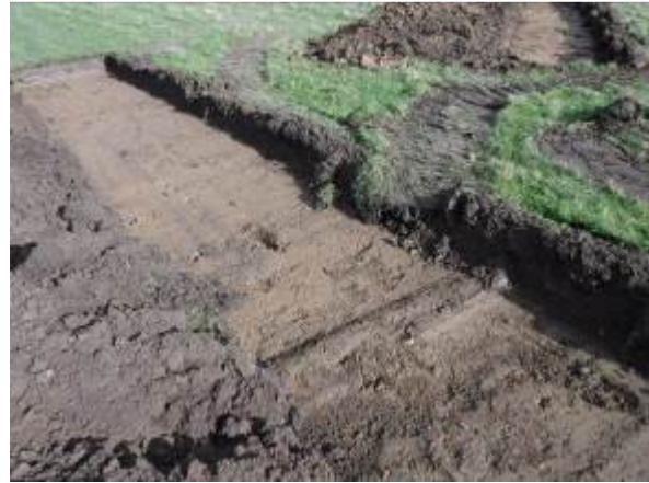
Plate 18 : Trench 6, North end detail (photo 199)
