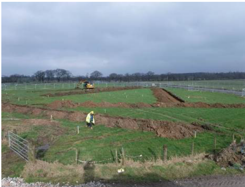
Plate 1 : North field, Showing Trenches 1-5 (photo 075)
