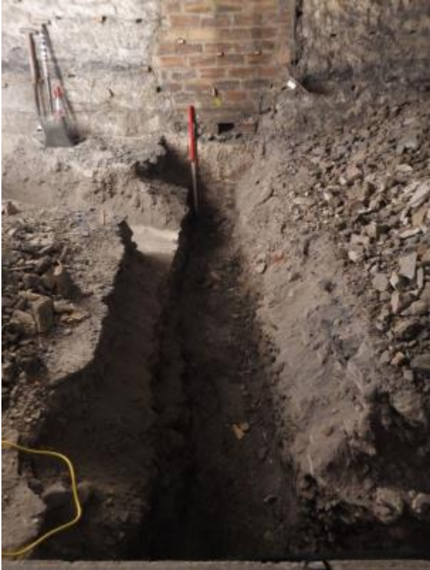
Plate 11 ST4, general view. Facing N
