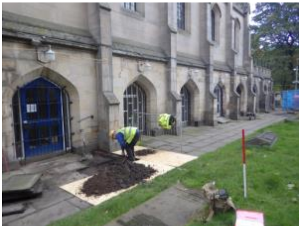
Plate 1 Hand-excavating test pits. Facing NE
