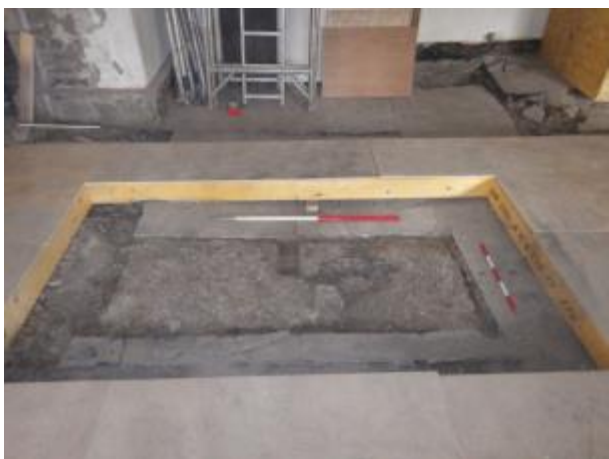
Plate 66 Foundations [017] after removal of overlying Paterson monument. Facing north.
