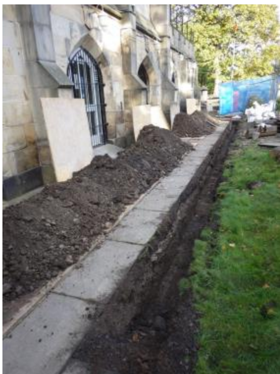
Plate 5 ST1, general view. Facing ENE
