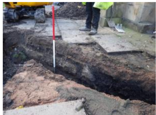
Plate 4 ST1, south-east-facing section. Facing NW
