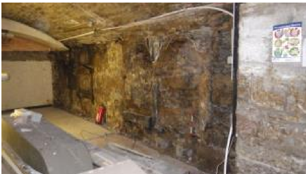
Plate 80 Arbuthnot Lair, general view with blocked round-headed windows. Facing north-west.
