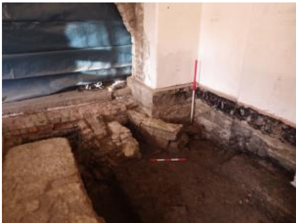
Plate 18 General view Drain [032]. Facing north-west
