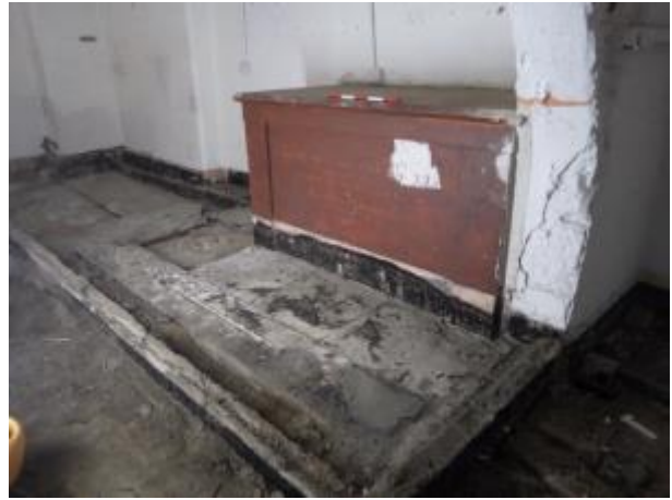
Plate 63 General view of Finch Hatton monument during works. Facing north-west
