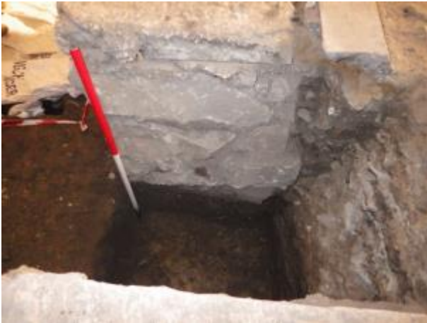
Plate 68 Foundations [017], W-facing elevation. Facing east.
