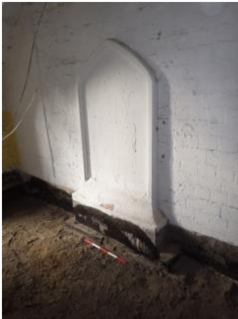
Plate 64 General view of Macdowal monument during works. Facing south-west
