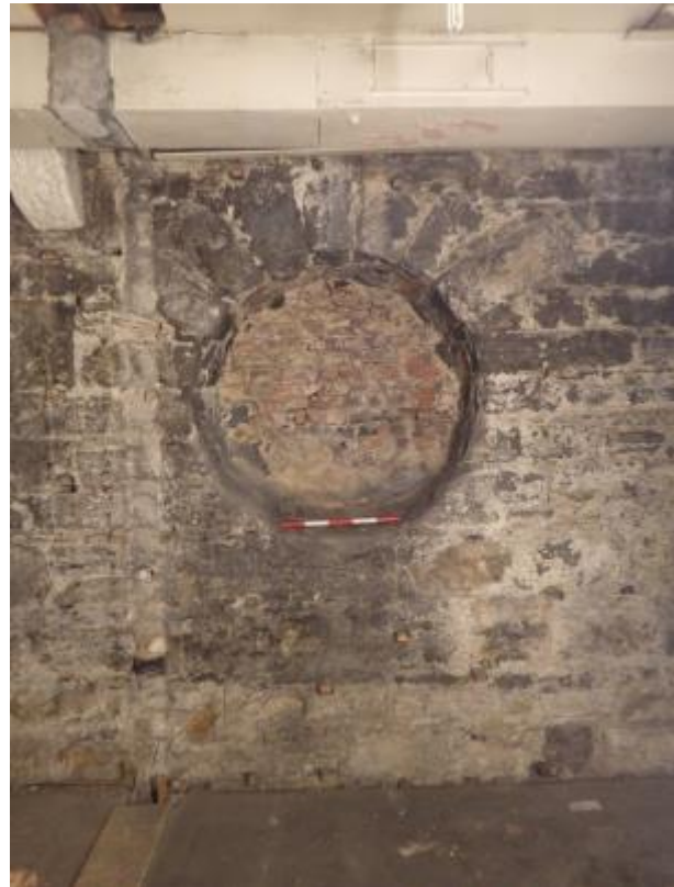
Plate 78 Blocked round light in undercroft. Facing north.
