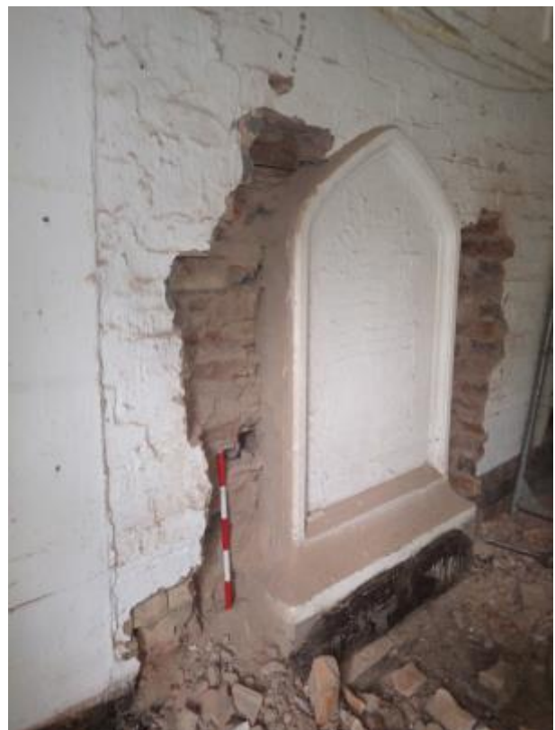
Plate 84 Partition wall in Macdowal Lair with monument. Facing north-west.
