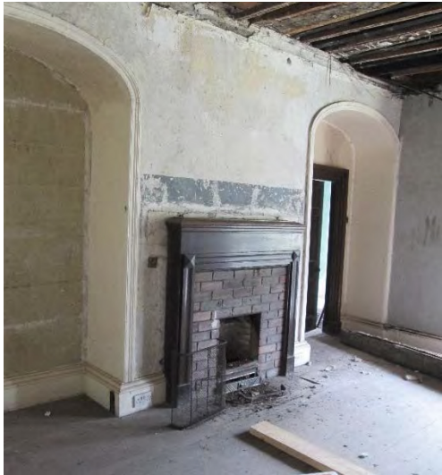
Plate 64 room G06 fireplace
