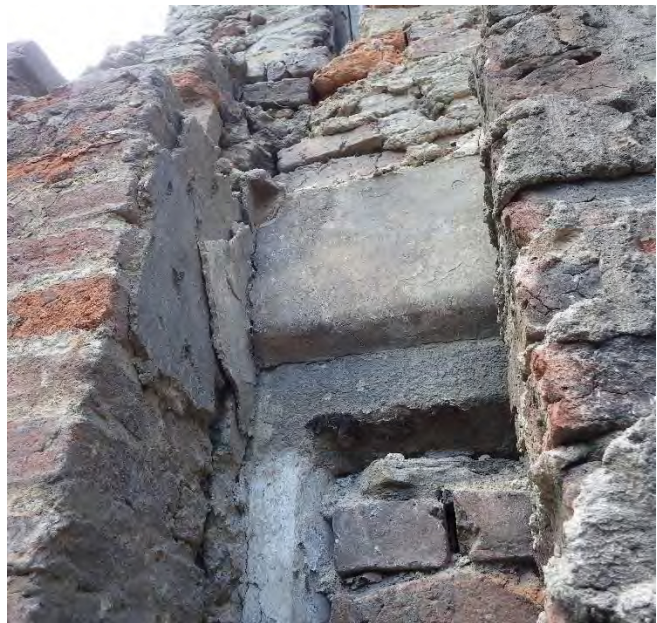
Plate 67 early window G03/G05 detail of plaster
