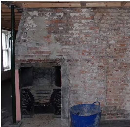
Plate 24 S08 fireplace in situ
