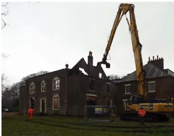
Plate 6 Mechanical demolition
