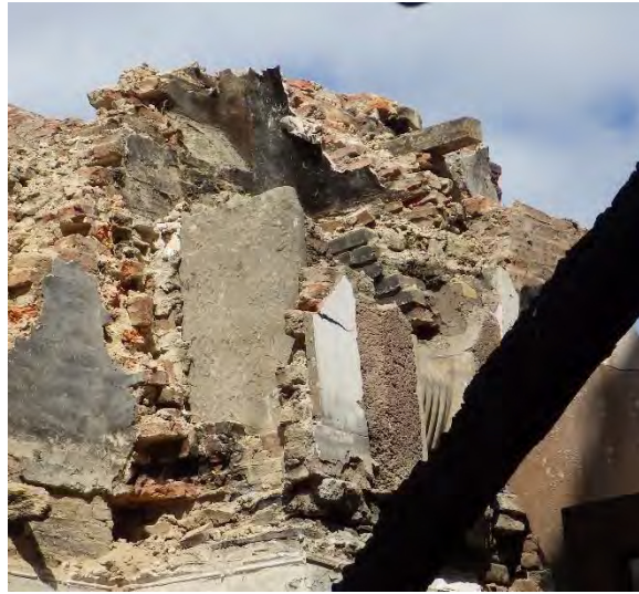
Plate 51 F09 - fireplace under demolition, revealing rear of side slab of original
