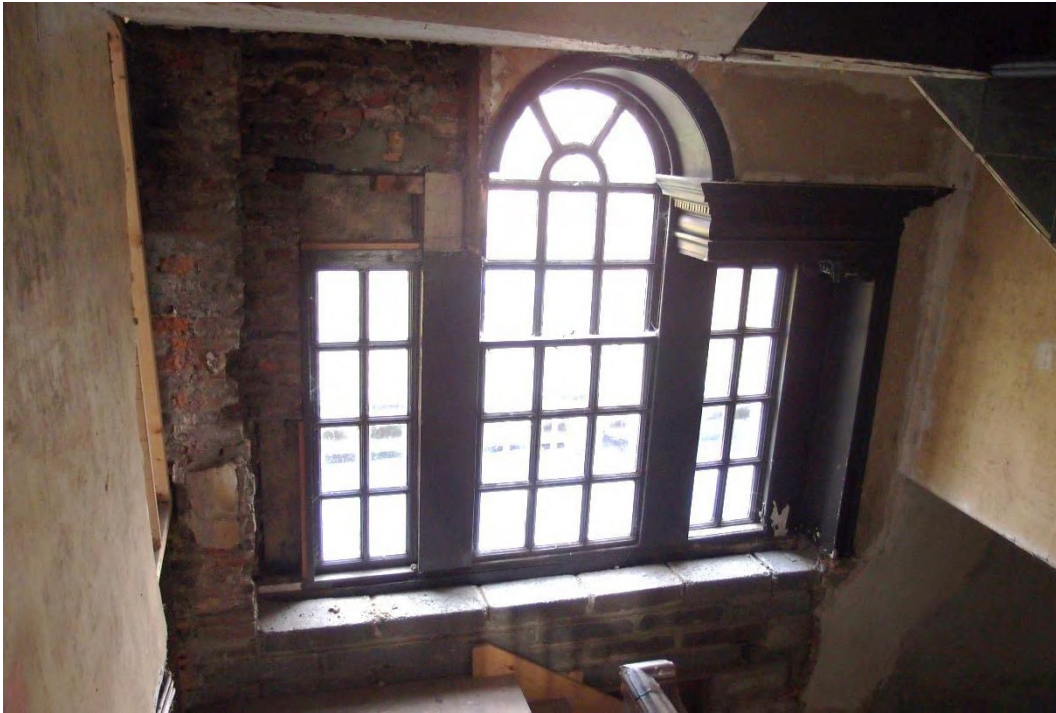
Plate 81 Stair window – view before the fire
