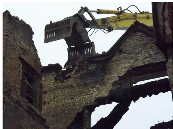
Plate 7 South-east gable during dismantling
