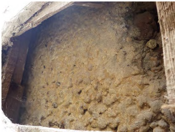
Plate 73 room G10 original exterior finish
