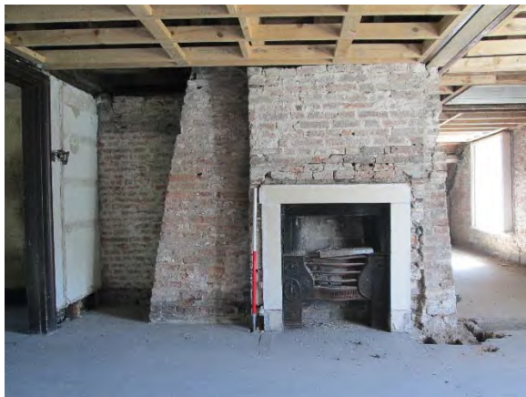
Plate 28 S07/6/5 fireplace in situ
