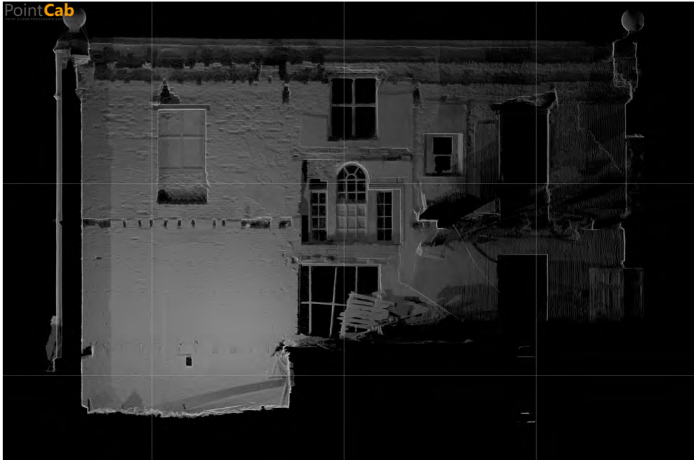
Northern interior (initial scan)
