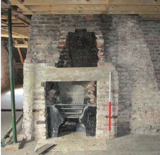
Plate 30 S04 fireplace in situ
