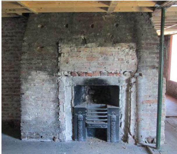
Plate 20 S09 fireplace in situ
