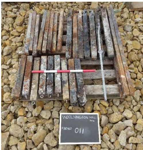
Plate 62 find no 011 bay window sash weights
