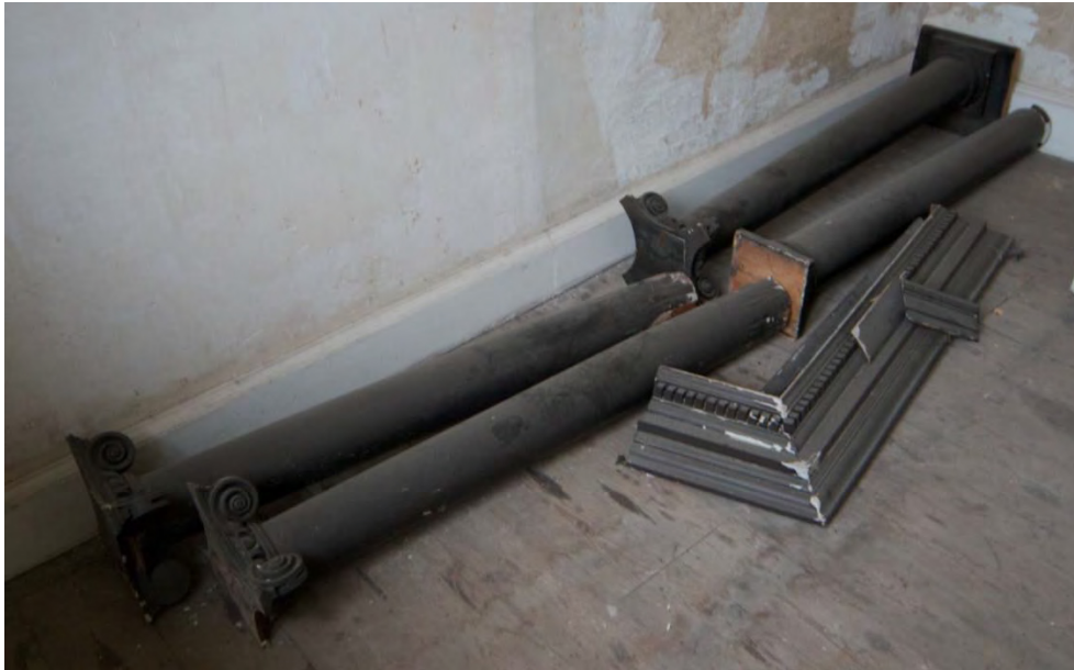
Plate 83 Stair window – ex situ sections of woodwork – destroyed in the fire
