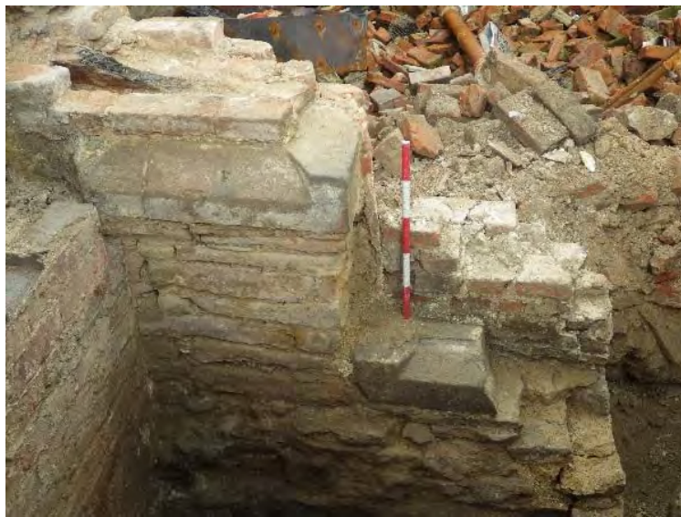
Plate 84 Room B03 - basement window remnants, looking east
