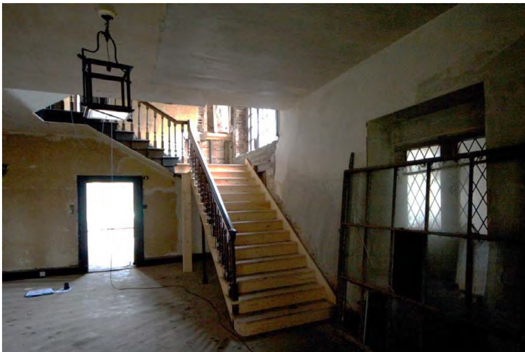
Plate 77 Stair hall, room G6, looking WNW towards the stairwell, showing re-alignment of the lower flight
