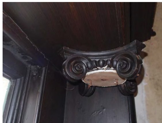
Plate 84 Stair window – detail of capital
