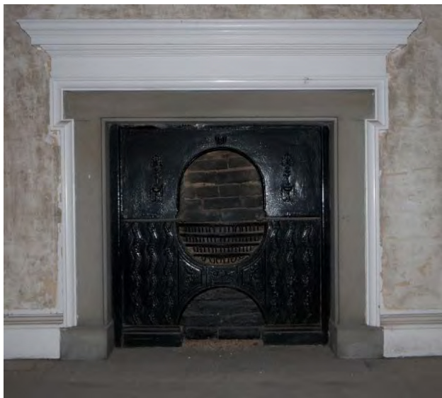
Plate 34 room F04 fireplace and surround in situ
