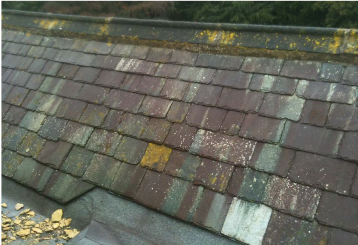
Plate 18 Roof ridge before the fire
