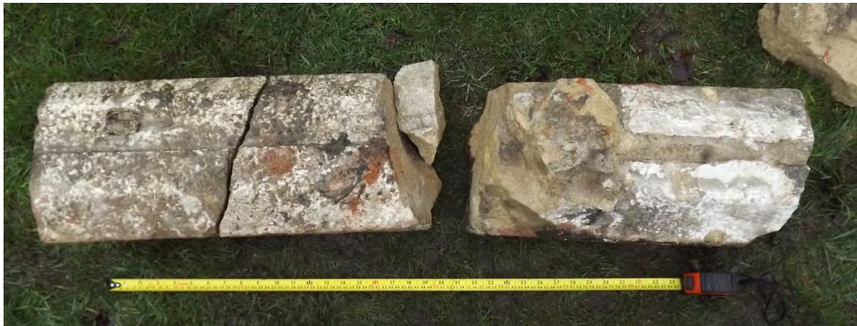
Example - initial identification, recovery and laying-out of shattered dressed window elements, prior to recording labelling and storage
