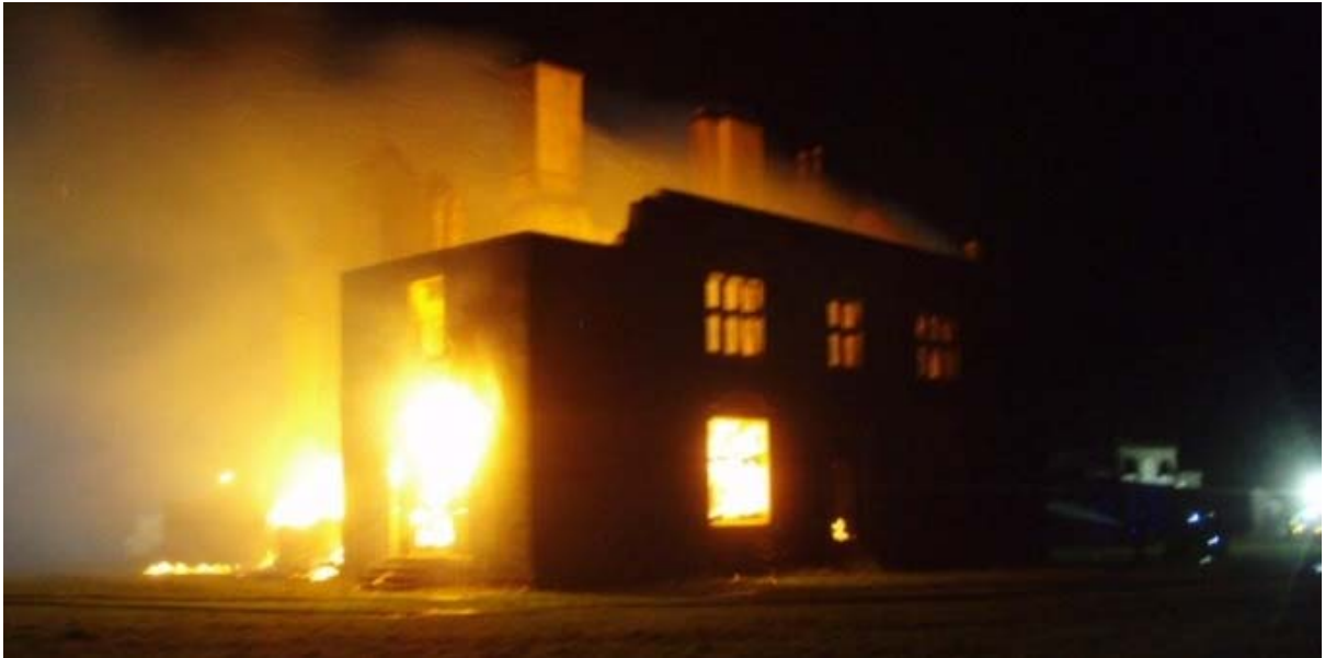
Plate 1 Fire in progress – evening of 29 December 2015 (Tyne Tees - ITV.com)
