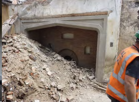
Plate 76 room G06 fireplace under excavation
