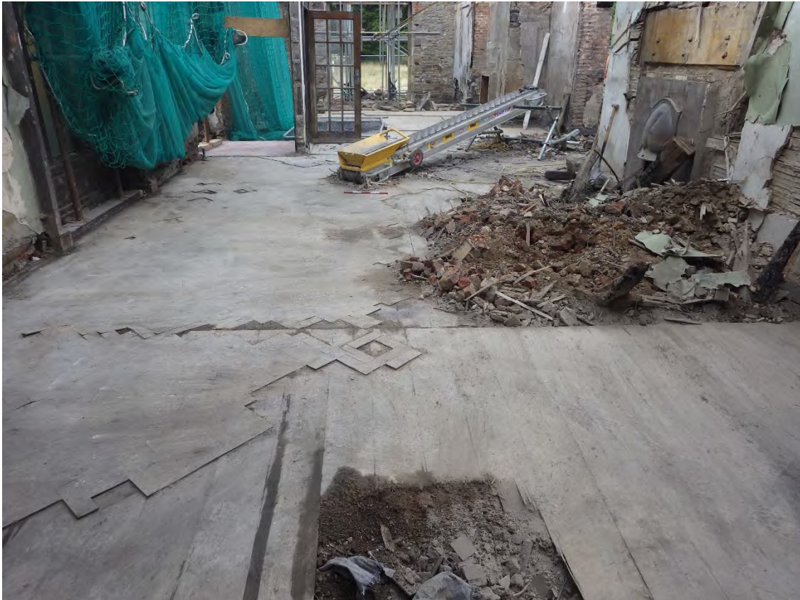
Plate 56 Room G09 flooring as exposed
