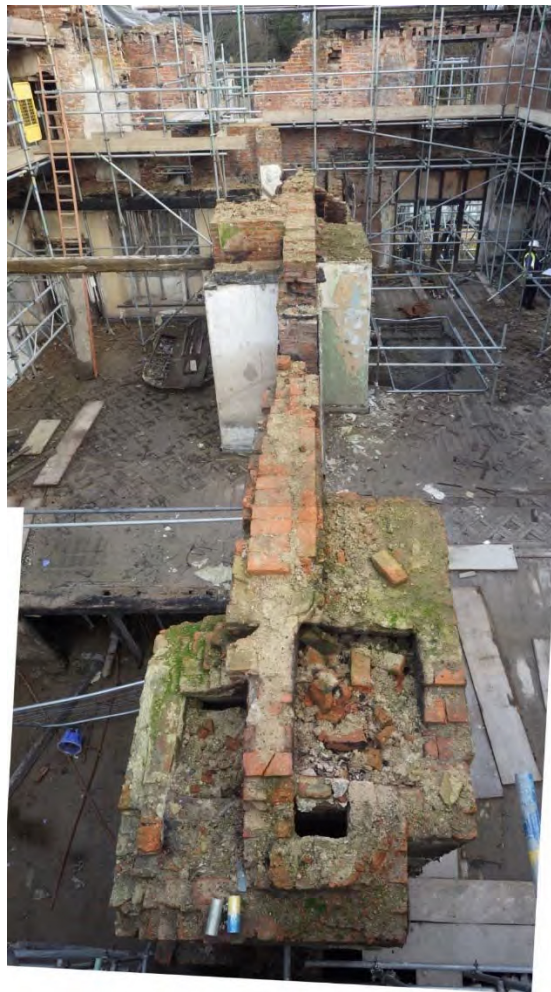
Plate 14 The masonry of the spine wall following further reduction
