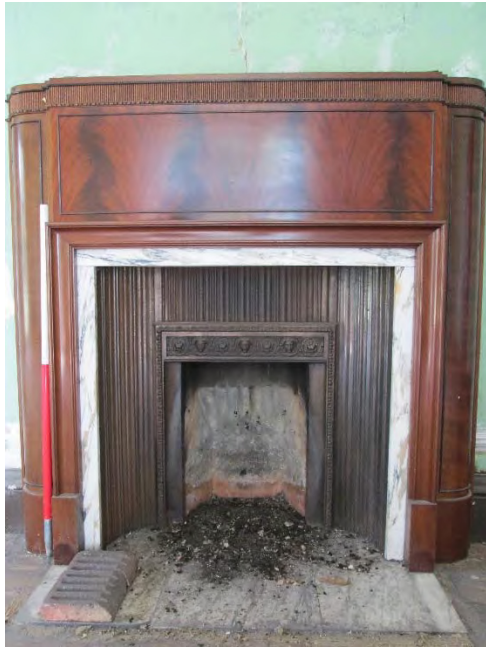
Plate 57 room G03 fireplace pre fire
