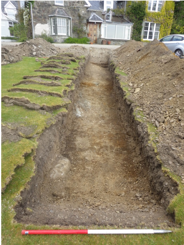
Plate 7 Trench 3, general view post-ex. Facing north-east
