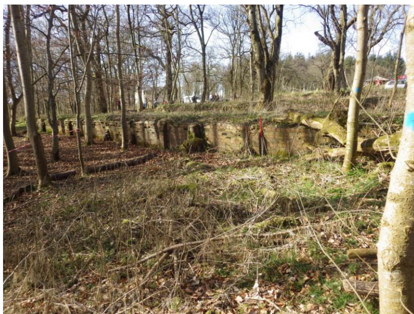
Plate 13 Hut 5, south elevation, looking north-west
