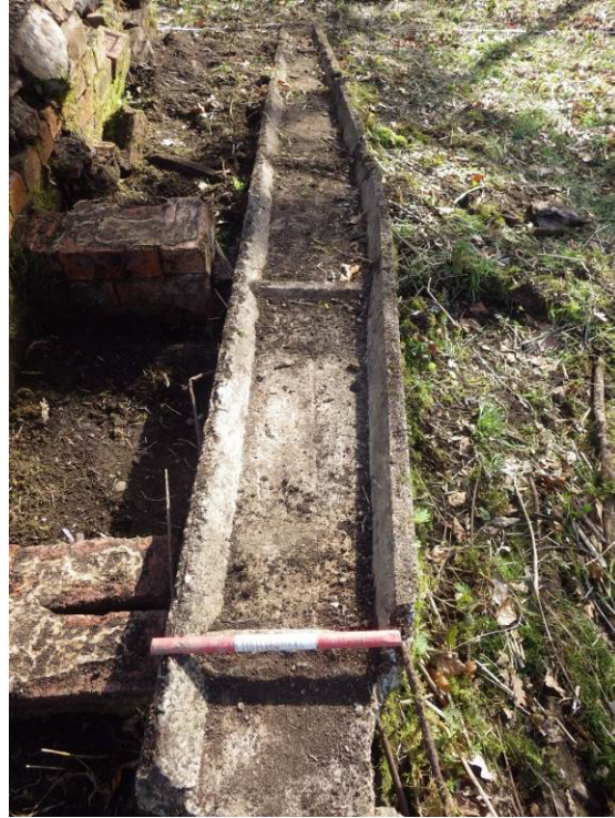
Plate 12 Hut 3, concrete drainage feature, looking south
