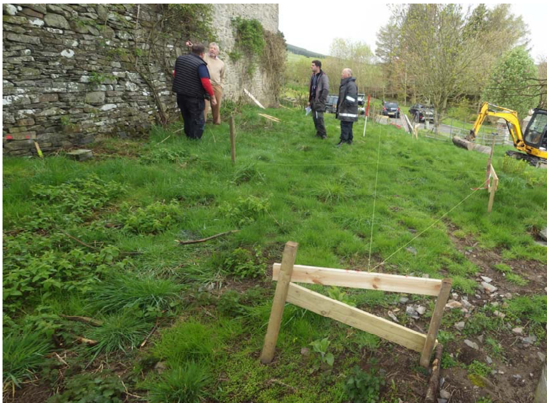
Plate 1 pre excavation view of building with foundations laid out
