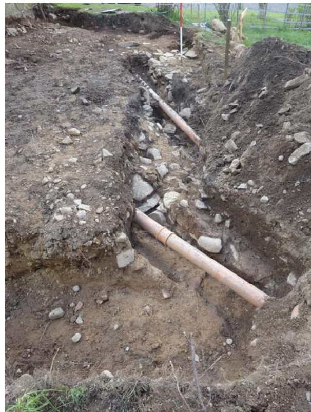
Plate 5 north trench general view to west showing 014 clay and rubble stone cut by modern services
