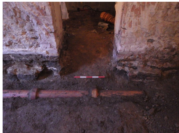
Plate 4 Drain (9131) in Cut [9130] with masonry blocks [9132] (left) and [9133] (right). Facing west
