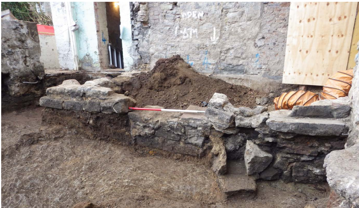
Plate 11 East elevation of Walls [9003] (right, with Drain [9007]) and [9004] (left) showing differences in coursing. Facing south-west.
