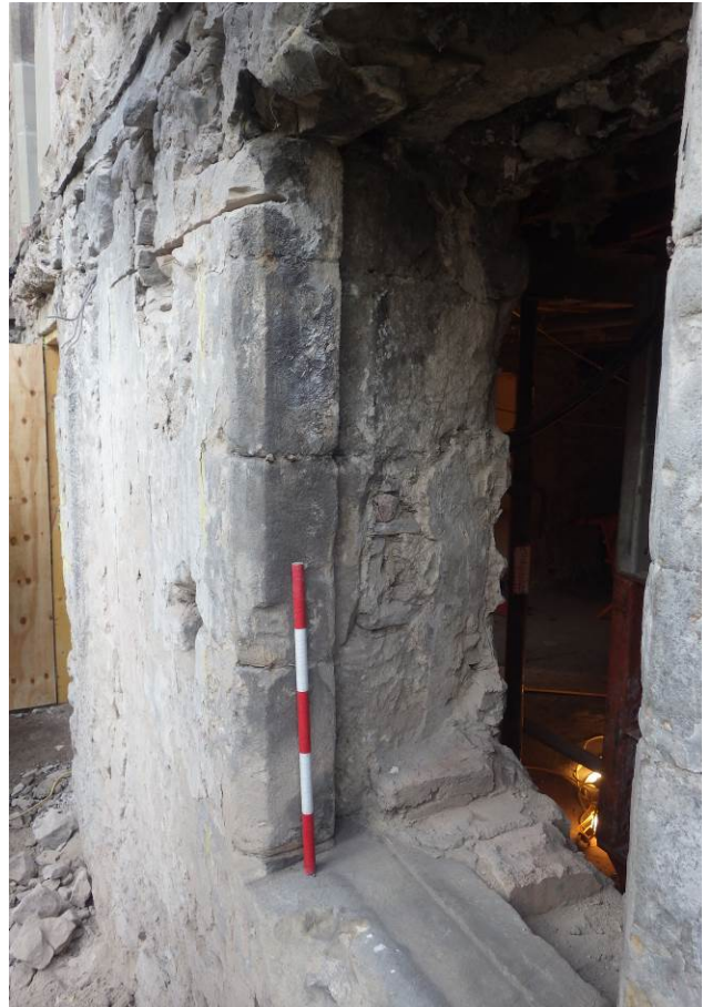
Plate 16 Window fully opened up shows west jamb
