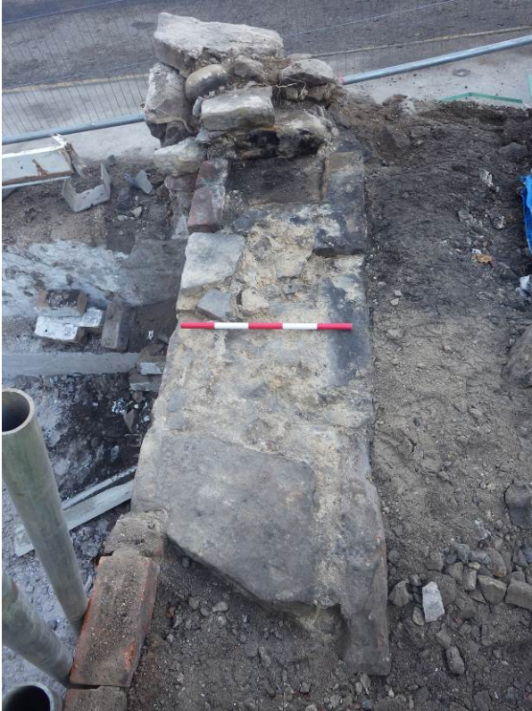
Plate 8 South elevation of lean-to, shows flue at east end (top)
