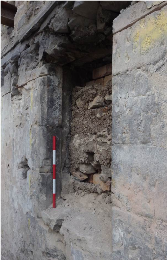
Plate 15 Window exterior rubble blocking removed exposing back of modern infill
