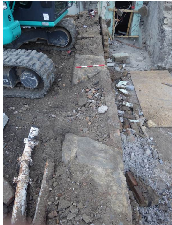
Plate 4 Window exposed on south elevation of lean-to
