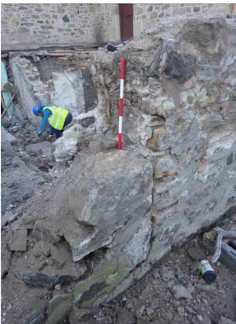
Plate 6 Vertical jamb at end of clay masonry to west under excavation. Lime bonded masonry of lean-to formerly abutting to right
