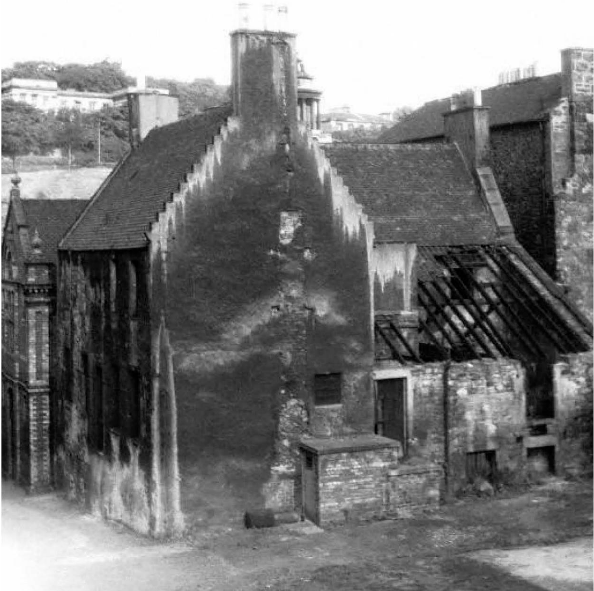
Plate 2 Historic photo from the 1920s? Shows earlier stair arrangement to the basement at the south gable
