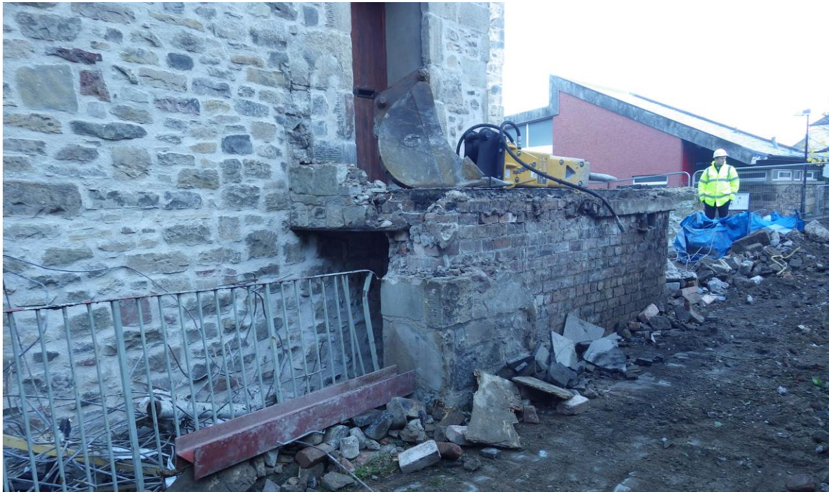
Plate 1 Stairs under demolition, showing rubble skin over brick
