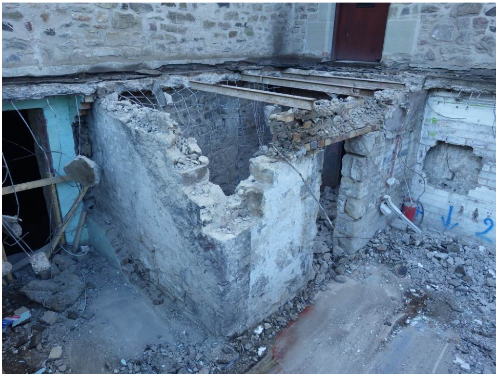
Plate 11 Stair tower remnant as exposed following demolition of concrete roof
