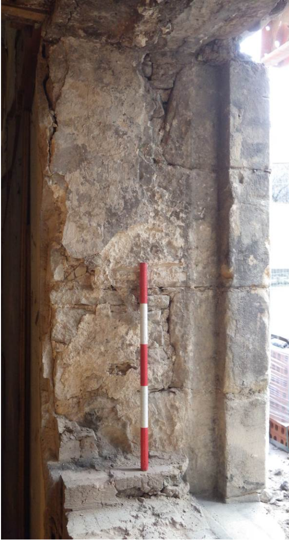
Plate 19 East ingo of window showing plaster in situ
