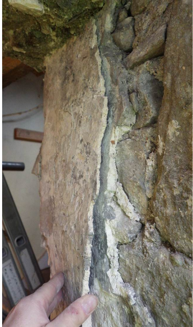
Plate 20 Plaster on ingo showing 2 phases
