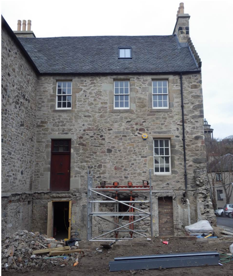
Demolition works in progress, Panmure House
