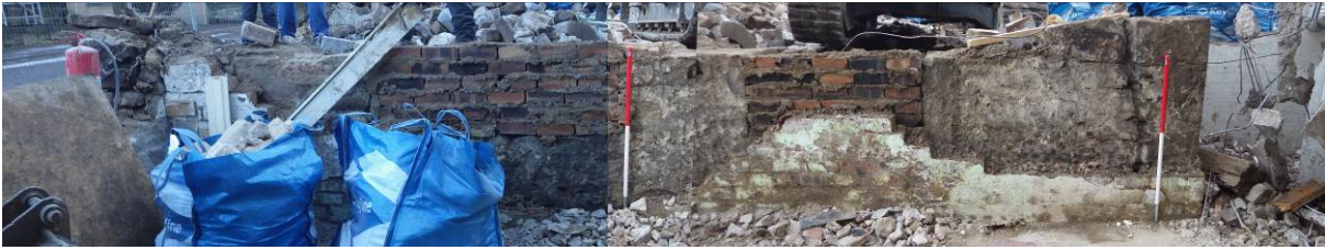
Plate 5 Interior face of south wall, lean-to shows blocked openings
