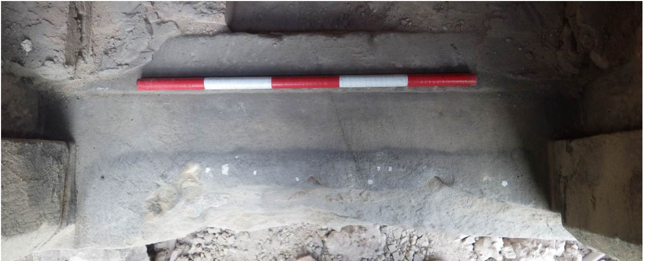
Plate 17 Window cill showing imprint of window case and 3 bar holes
