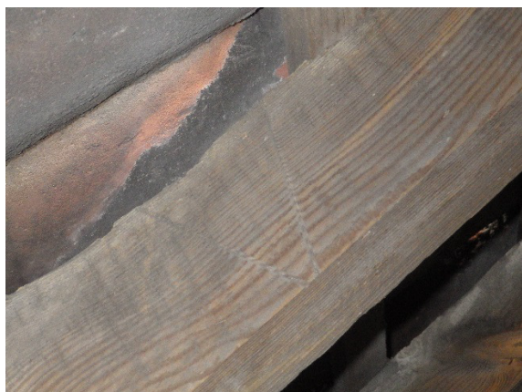
Plate 15 Truss 14 rafter 039 cut number "V" 100
