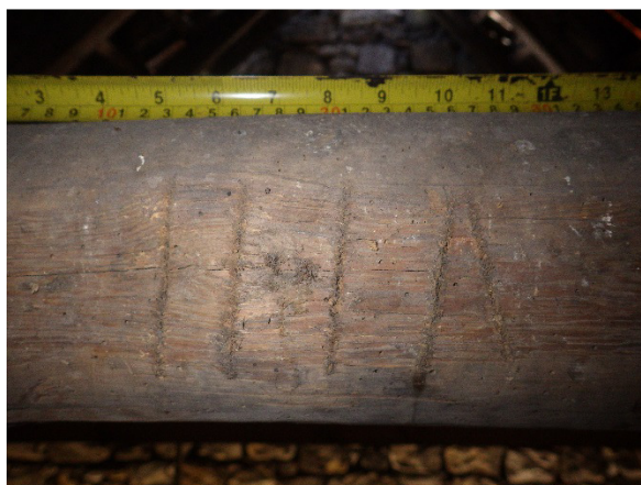
Plate 29 Truss 13 cut no 097
