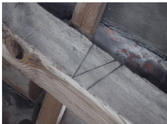
Plate 16 Truss 15 rafter 041 cut number "VI" 102
