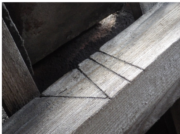
Plate 17 Truss 16 rafter 045 cut number "VII" 107
