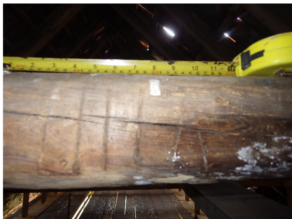
Plate 30 Truss 6 cut no 068
