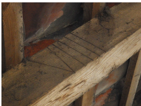
Plate 19 Truss 7 rafter 018 cut number "VIII" 070
