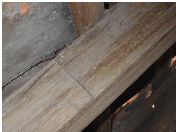
Plate 11 Truss 10 rafter 027 cut number "I" 081
