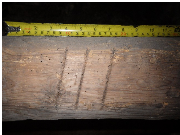
Plate 26 Truss 3 cut no 057
