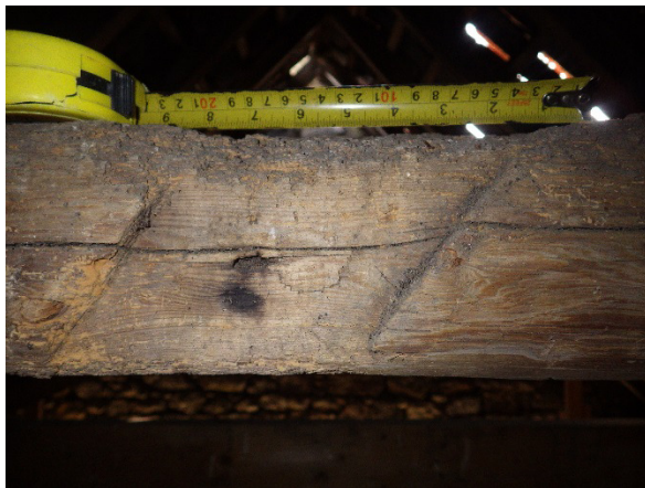
Plate 3 Rafter 031 , collar joint 086
