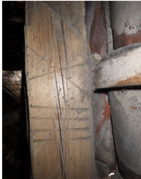
Plate 6 Truss 3 rafter 007 , shows cut number 055
