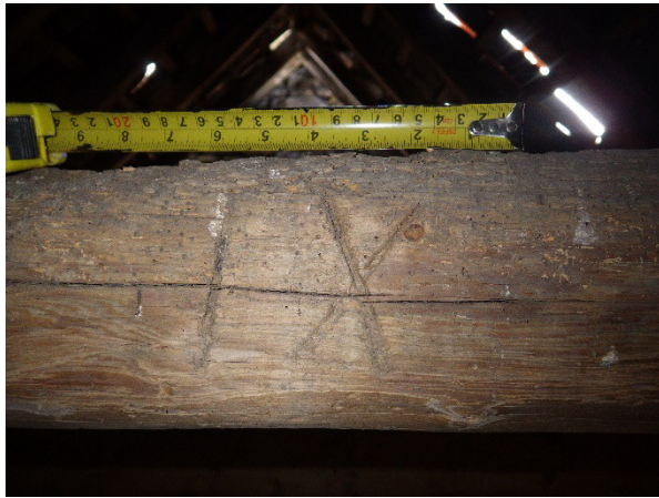
Plate 1 Feature 087 Sawn "IX" on rafter 031
