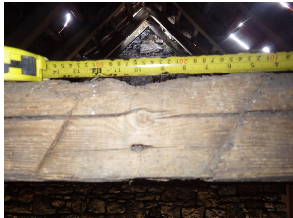
Plate 4 Rafter 034 , collar joint 091
