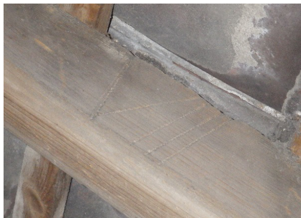
Plate 18 Truss 8 rafter 021 cut number "VIII" 075
