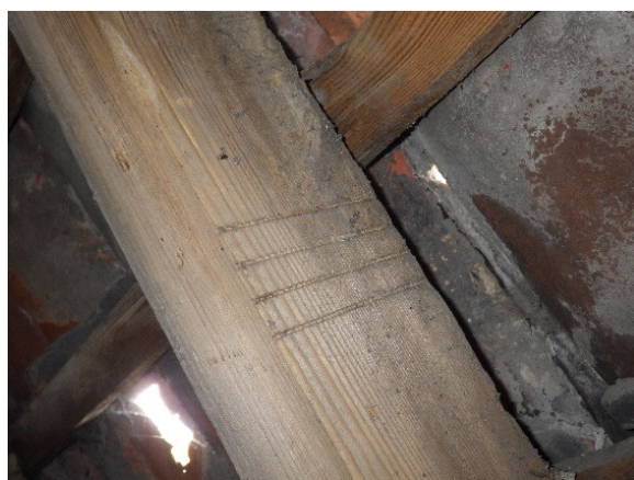
Plate 14 Truss 12 rafter 032 cut number "IIII" 089
