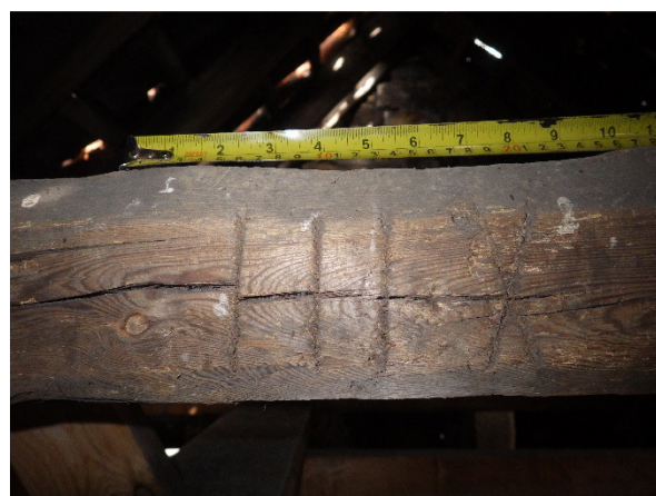
Plate 34 Truss 5 cut no 064
