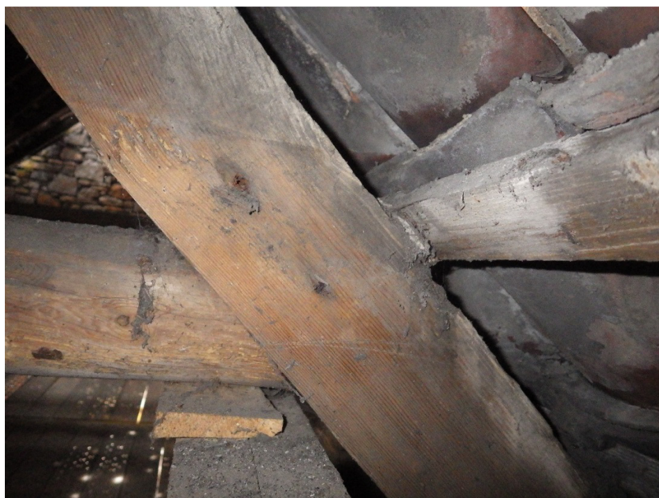
Plate 10 Truss 6 rafter 016 shows scribing and spike/s for original collar
