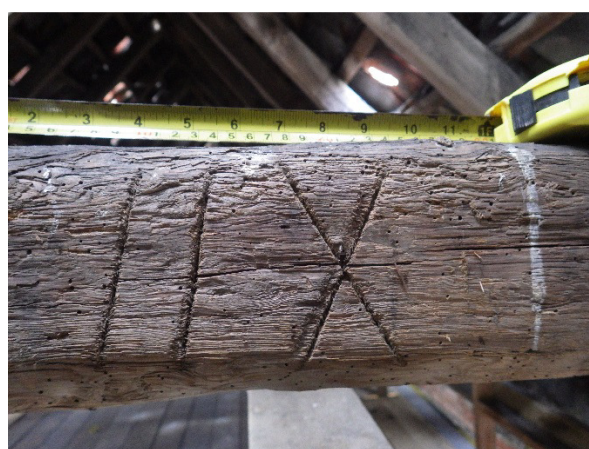
Plate 33 Truss 16 cut no 108
