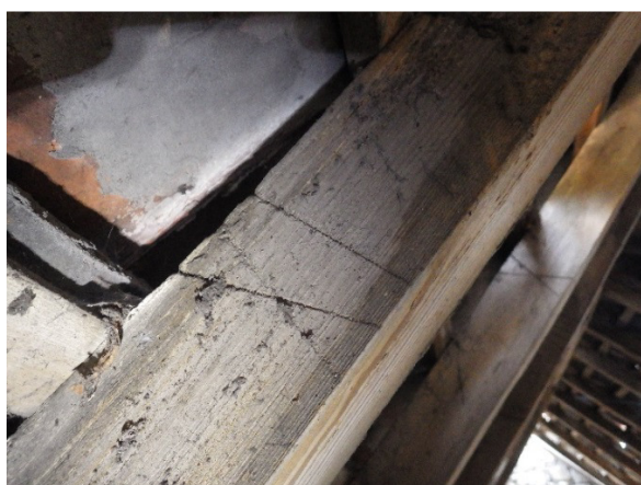
Plate 21 Truss 5 rafter 012 cut number "XI" 062
