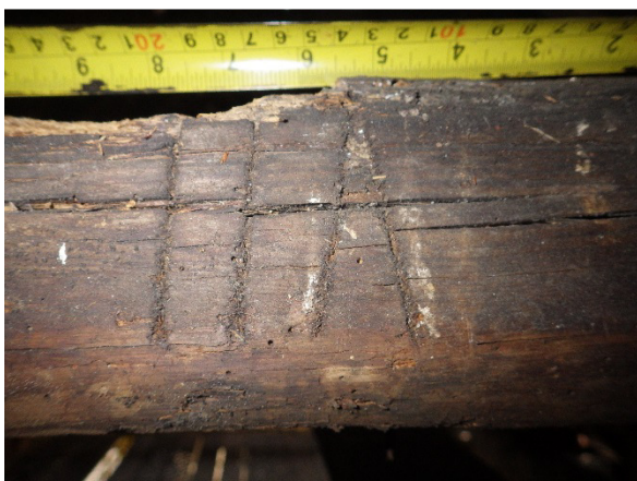
Plate 28 Truss 8 cut no 076
