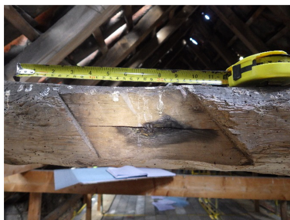
Plate 35 Truss 16 relic collar slot 109
