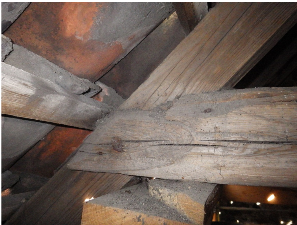
Plate 9 Collar 031 shows original form with end chamfered and spiked
