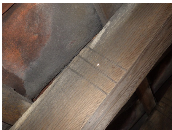
Plate 13 Truss 13 rafter 036 cut number "III" 096
