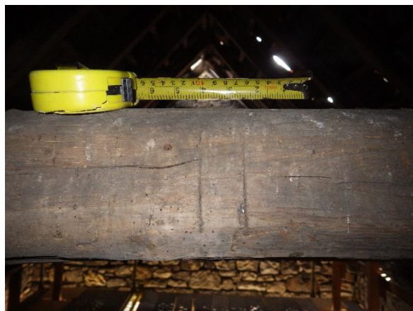
Plate 25 Truss 10 cut no 082
