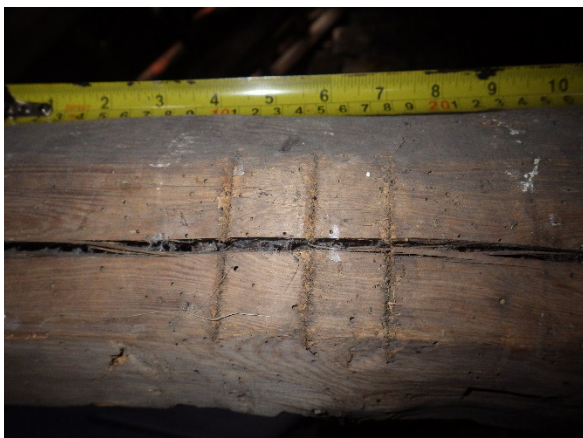
Plate 27 Truss 4 cut no 060
