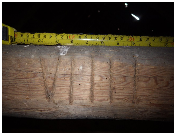
Plate 31 Truss 7 cut no 072
