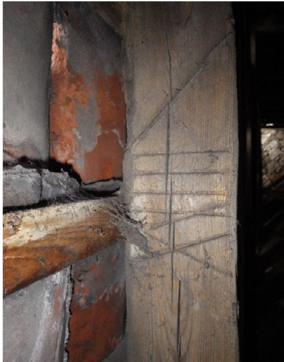
Plate 5 Truss 3 rafter 006 , shows cut number 054
