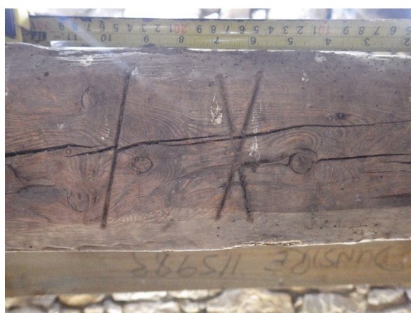
Plate 32 Truss 15 cut no 104
