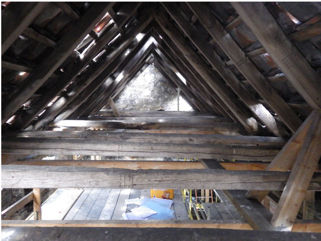
Plate 23 View along roof showing phase C collars
