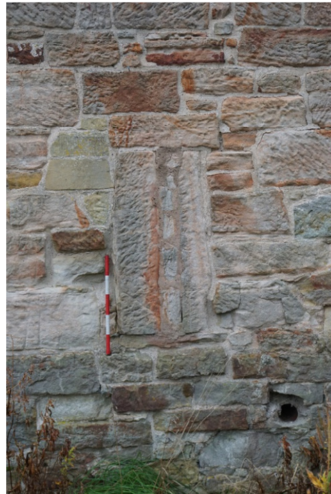
Plate 9 Blocked vent 41
