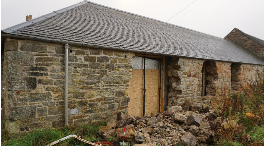
Plate 6 Building 2 NW elevation
