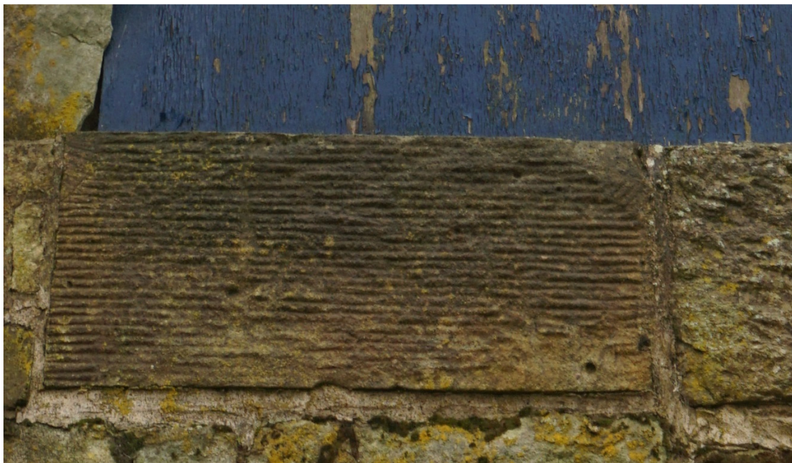
Plate 16 Reused stone with droved margins
