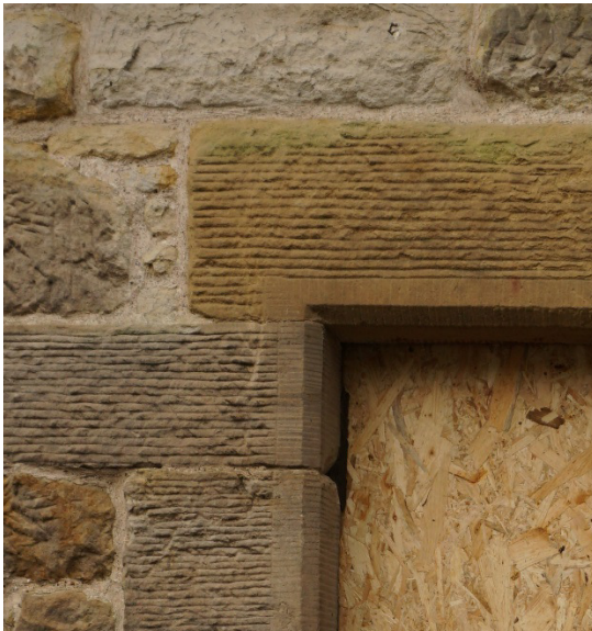
Plate 4 Detail of door chamfer and tooling on jambs
