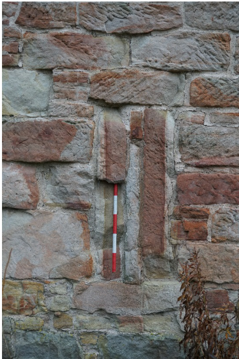
Plate 8 Blocked vent 38
