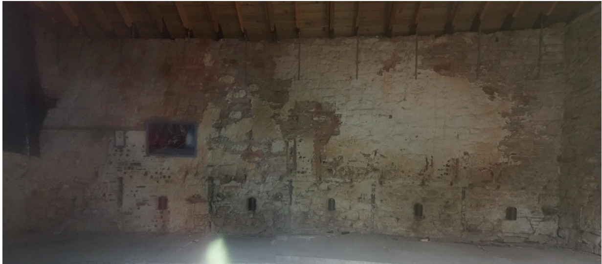
Plate 7 Building 3 north room composite north internal elevation (shot through glazed window)
