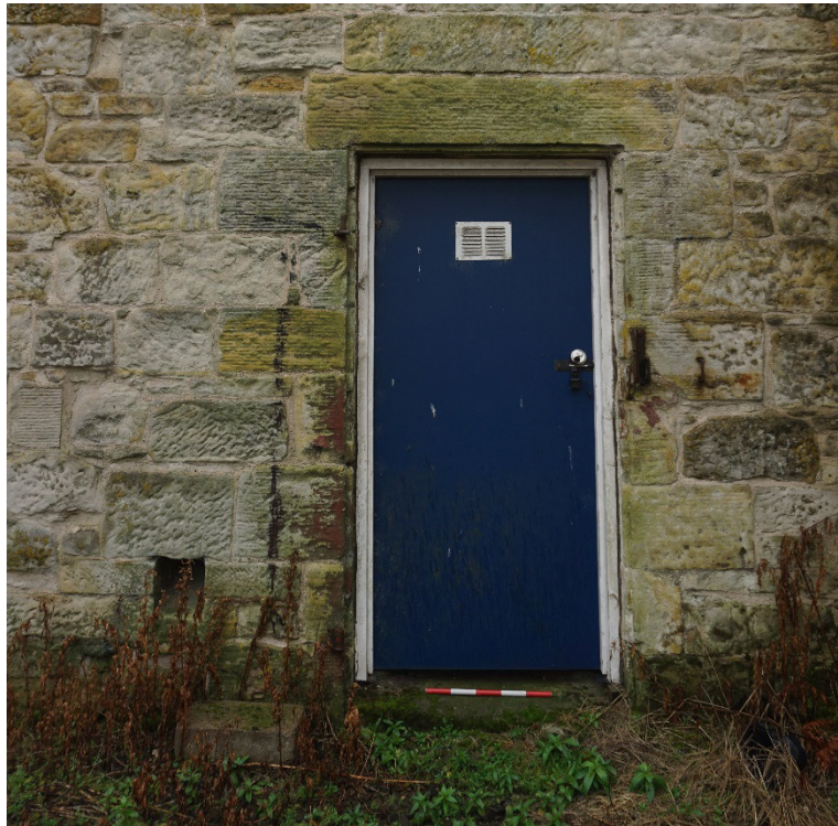
Plate 14 Building 4 west room door 26
