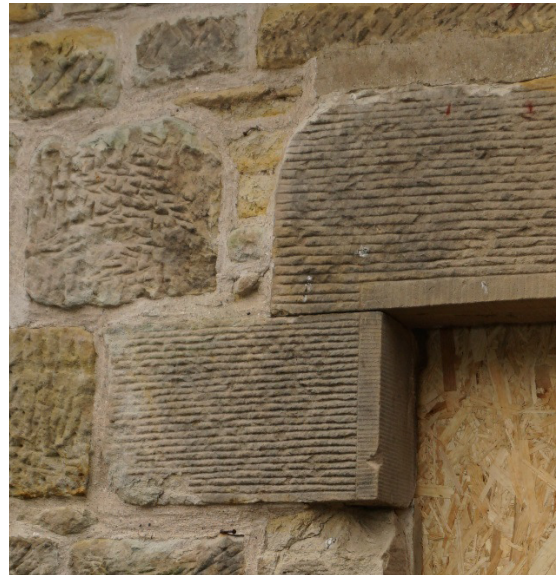
Plate 5 Detail of window jamb tooling
