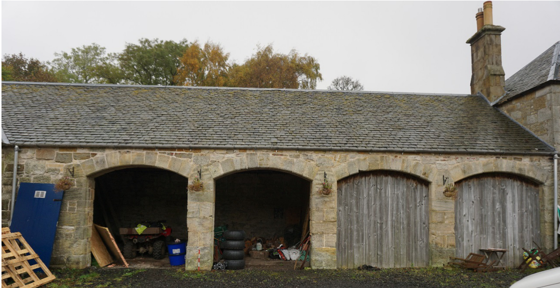
Plate 1 Building 1 shows arched openings
