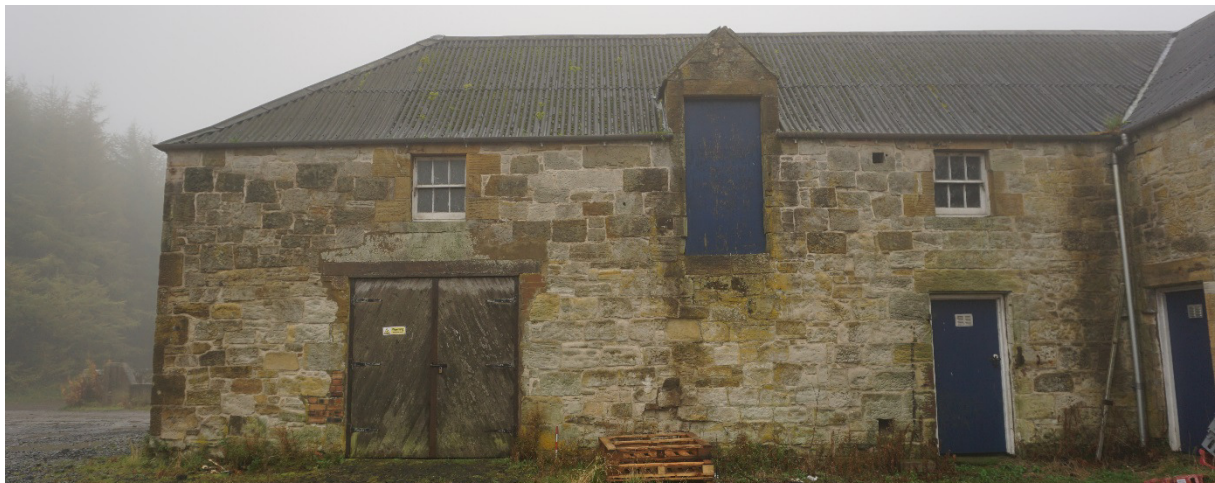
Plate 15 Building 4 NE elevation
