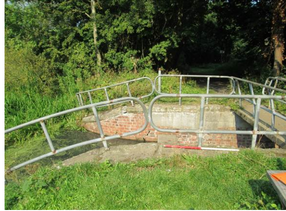
Plate 5 Site Outflow from reservoir facing north (061)
